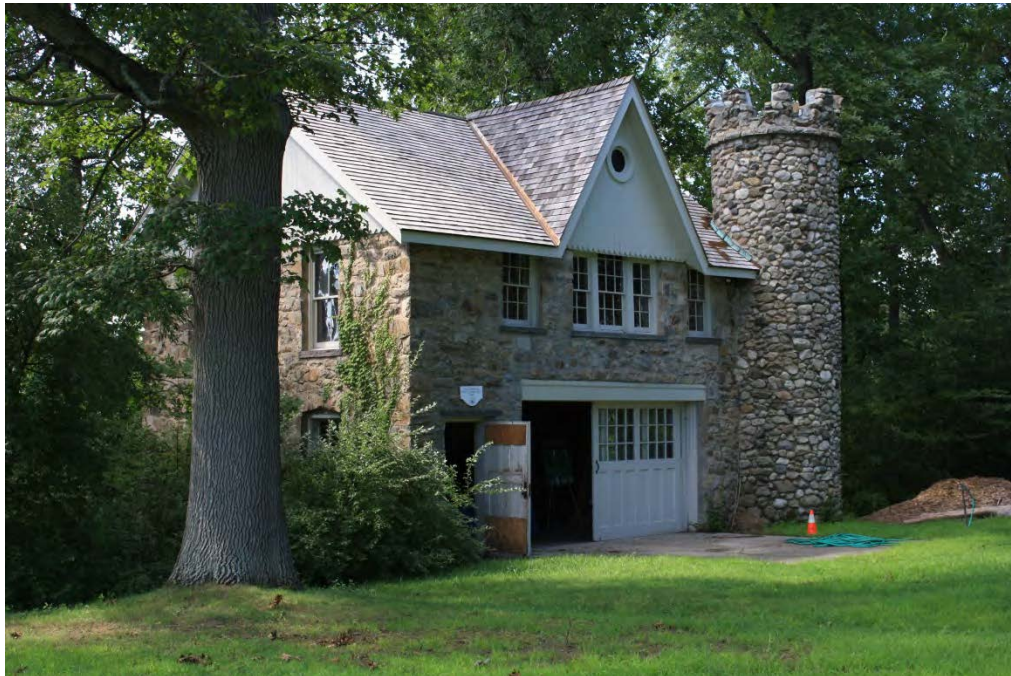
15. Southeast corner of carriage barn, camera facing northwest.
