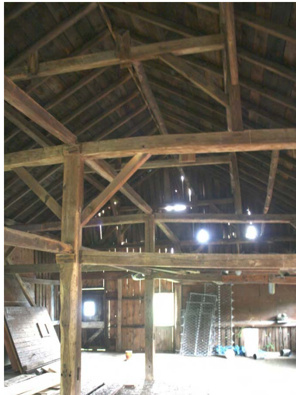
18. Interior view of upper level, Barn II, camera facing north.
