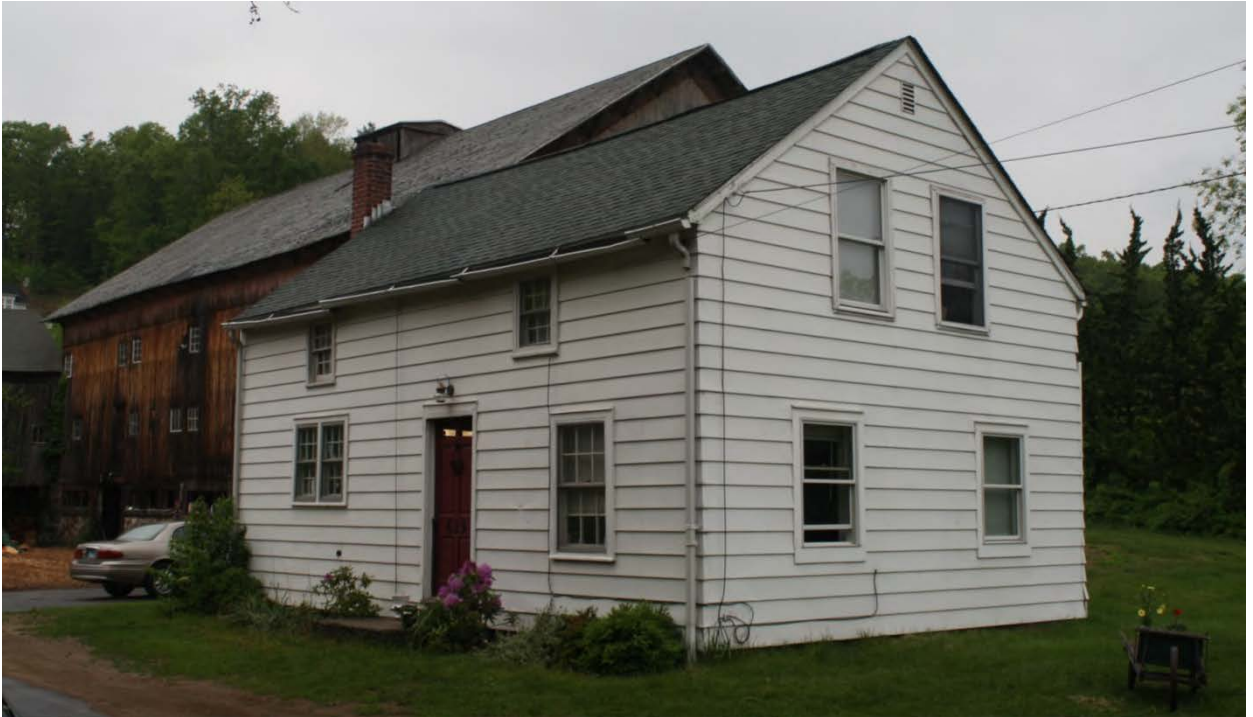
19. Southeast view of Barn III-House, camera facing northwest.
