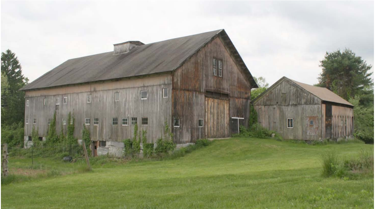
7. Northwest view of Barn I (left) and Barn II (right), camera facing southeast.
