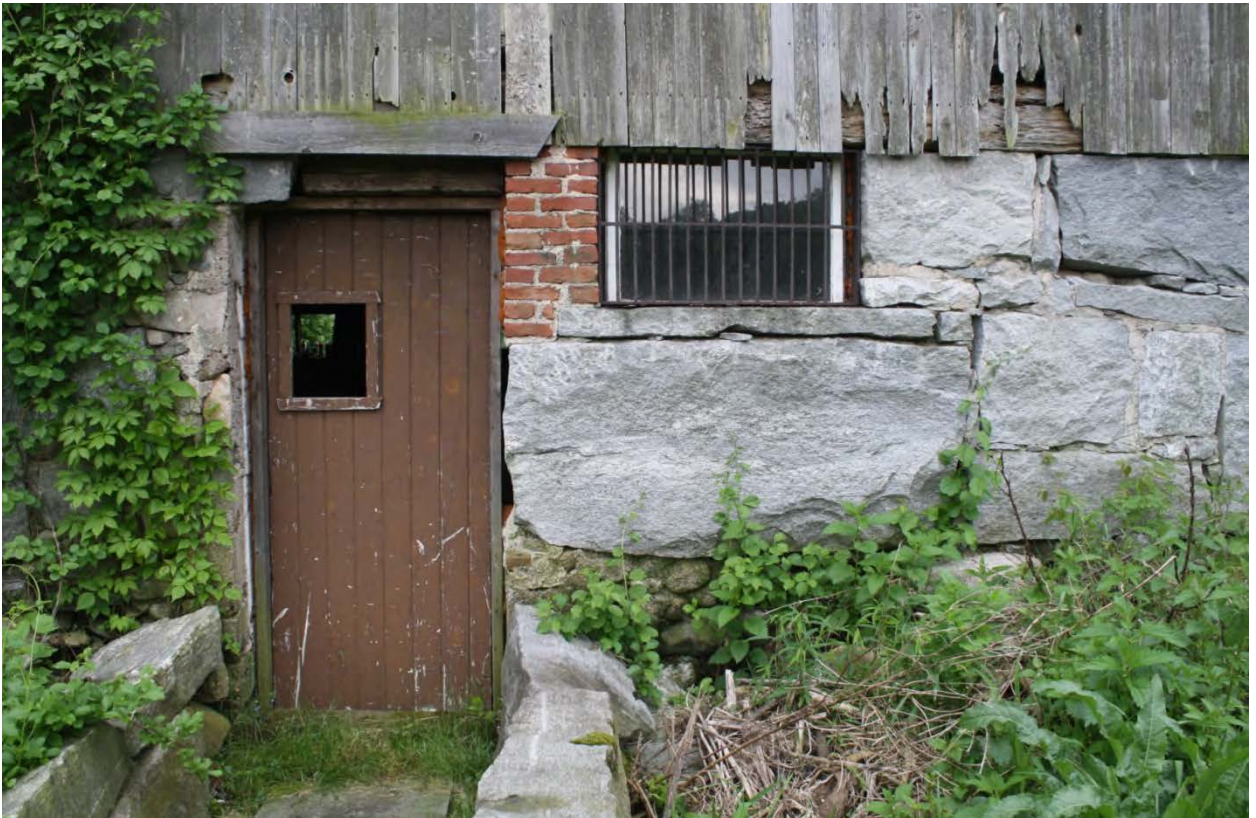
10. North detail view of Barn I stone foundation, camera facing south.
