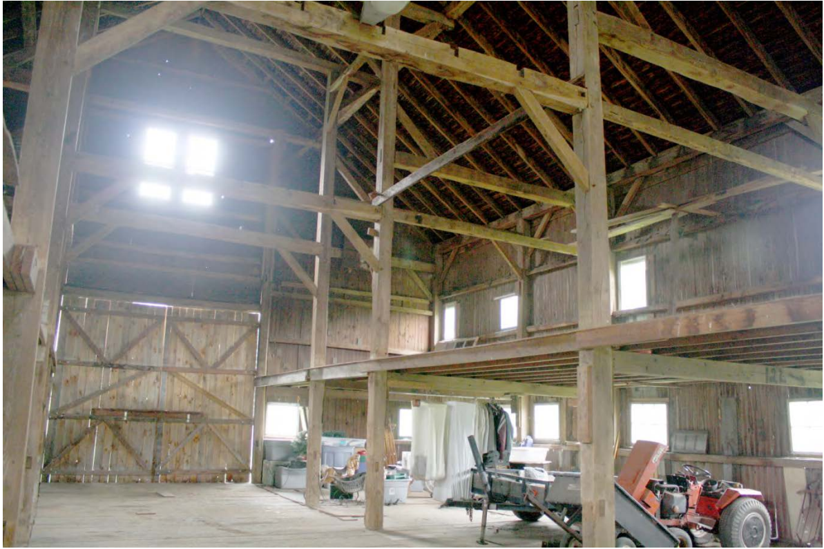
13. Interior view of Barn I main level, camera facing west.
