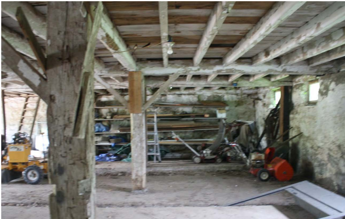
14. Interior view of Barn I, Basement level, camera facing west.
