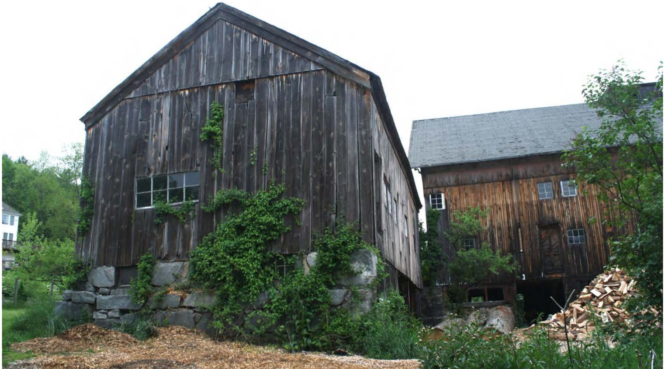
17. South view of Barn II, camera facing north.
