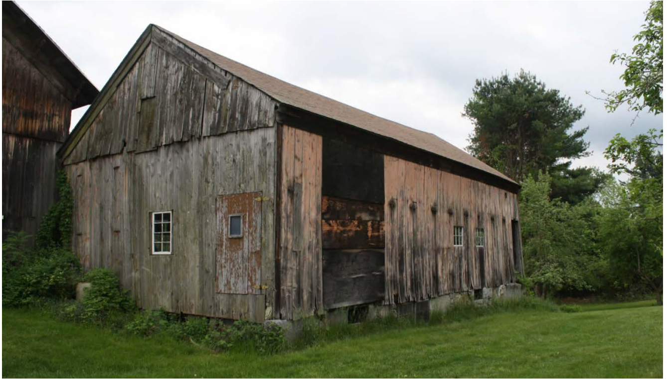
15. Northwest view of Barn II, camera facing southeast.
