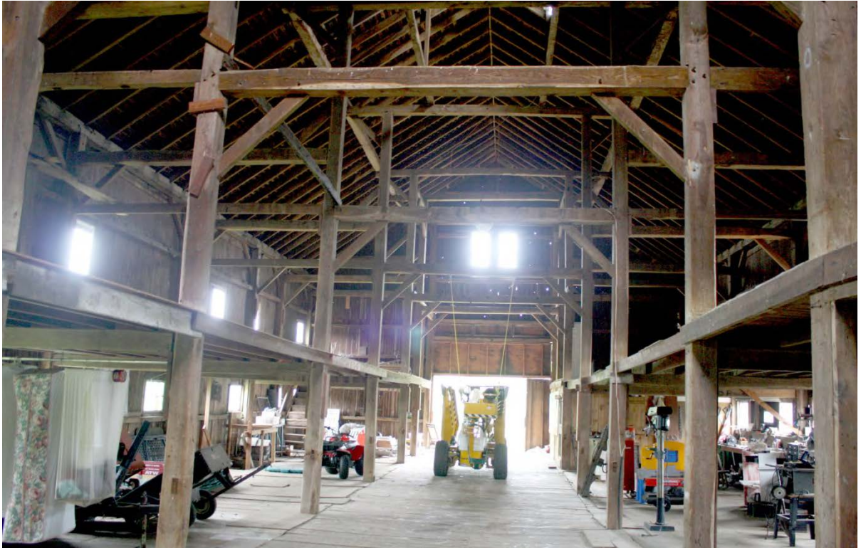
11. Interior view of Barn I main level, camera facing east.
