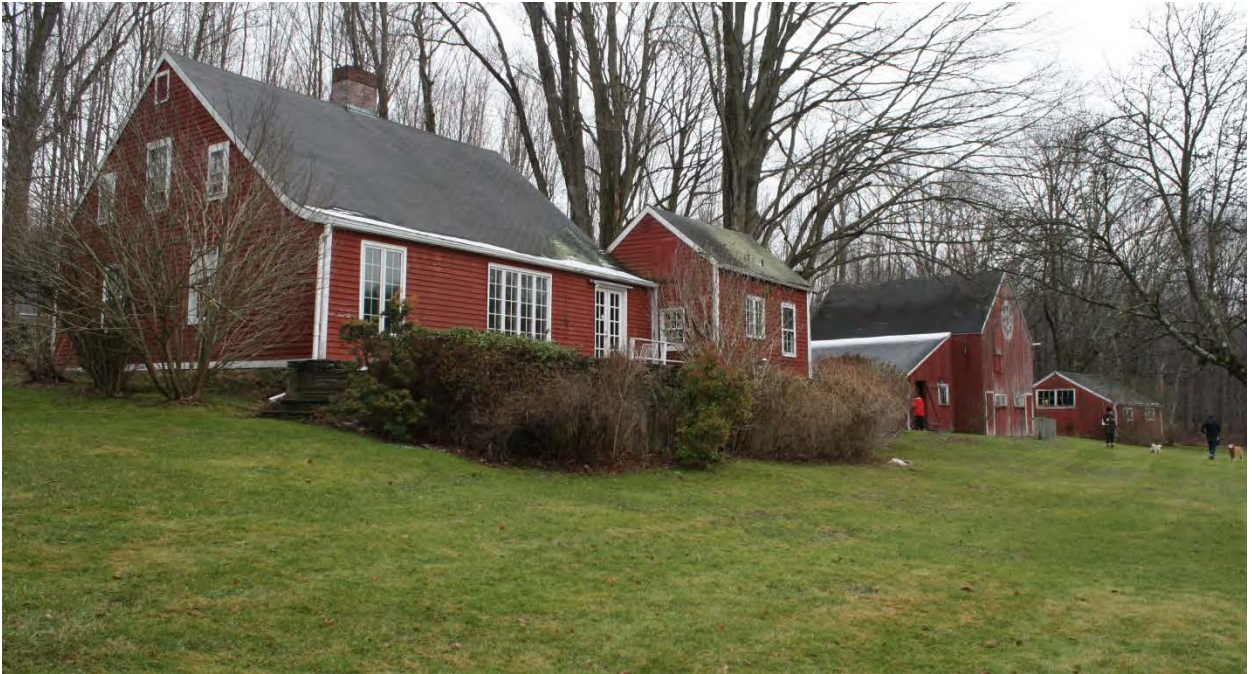
5. Northwest context view of 163 Carrington Road, Bethany, CT, camera facing southeast. From left to right: Farmhouse, Farmhouse kitchen addition, Barn I, Barn II.
