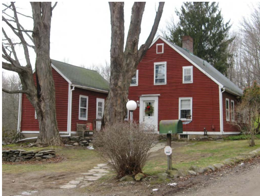
6. South and east elevations of Farmhouse and Farmhouse kitchen addition, camera facing north.
