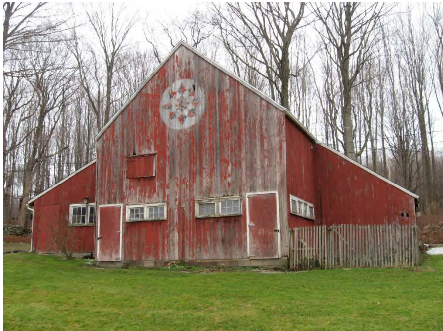
9. West and south elevations of Barn I, camera facing northeast. Note hay door and geometric detail in gable end.
