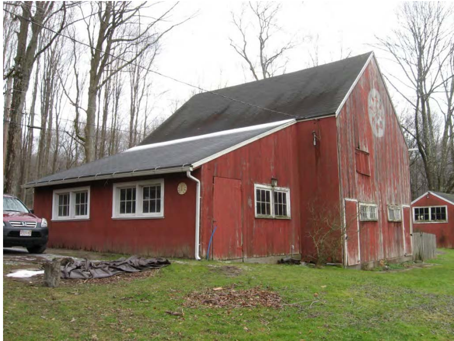
10. West and south elevations of Barn I, camera facing northeast.
