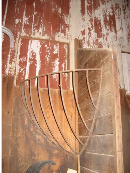
18. Interior view of Barn I north addition, showing horse stall hay catcher, camera facing south. Note hay door opening above.
