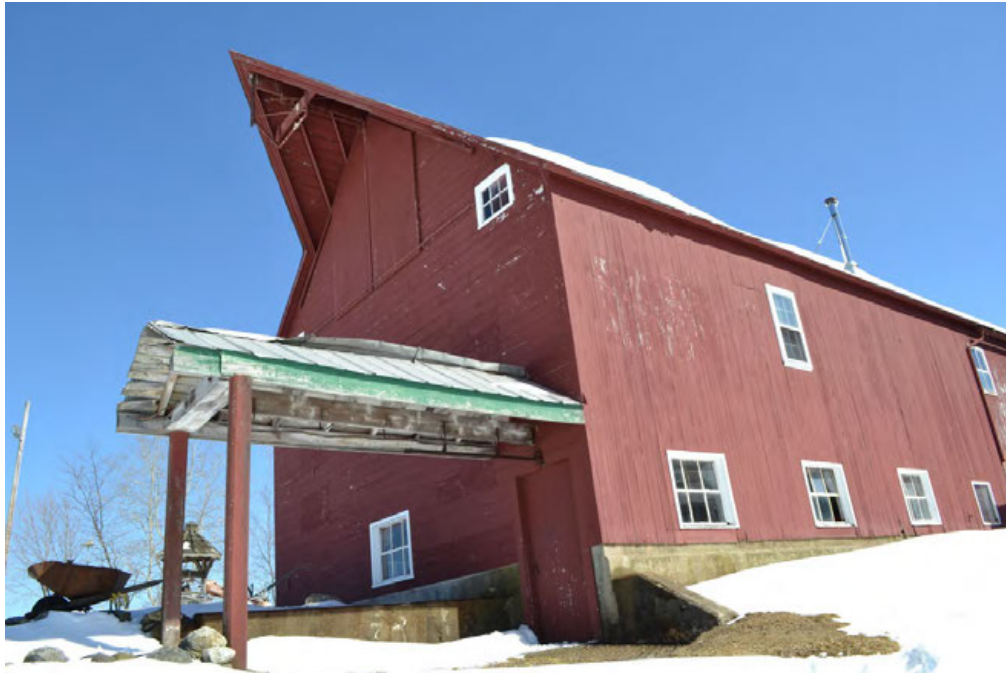
29. South eave-side and west gable-end of Barn I, camera facing northeast. Note covered manure trolley at middle left and projecting hood and hay track at upper left.
