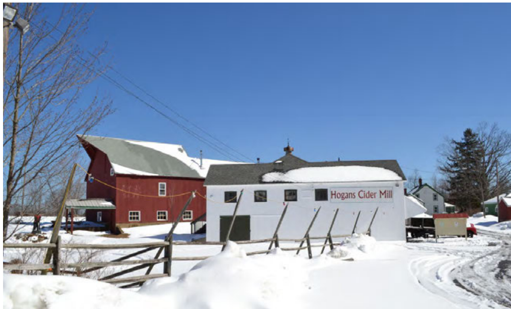
6. West context view of 522 Spielman Highway, Burlington, CT, camera facing east. From left to right, Barn I, Cider mill, Farmhouse, Garage I, Milk house.
