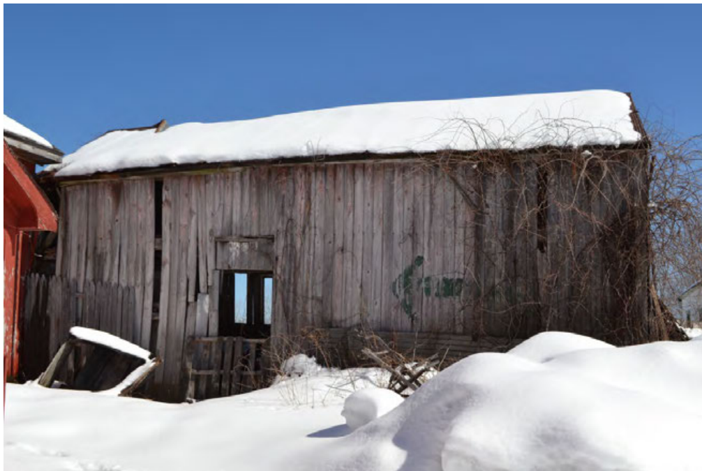
12. West eave-side of Barn II, camera facing east.
