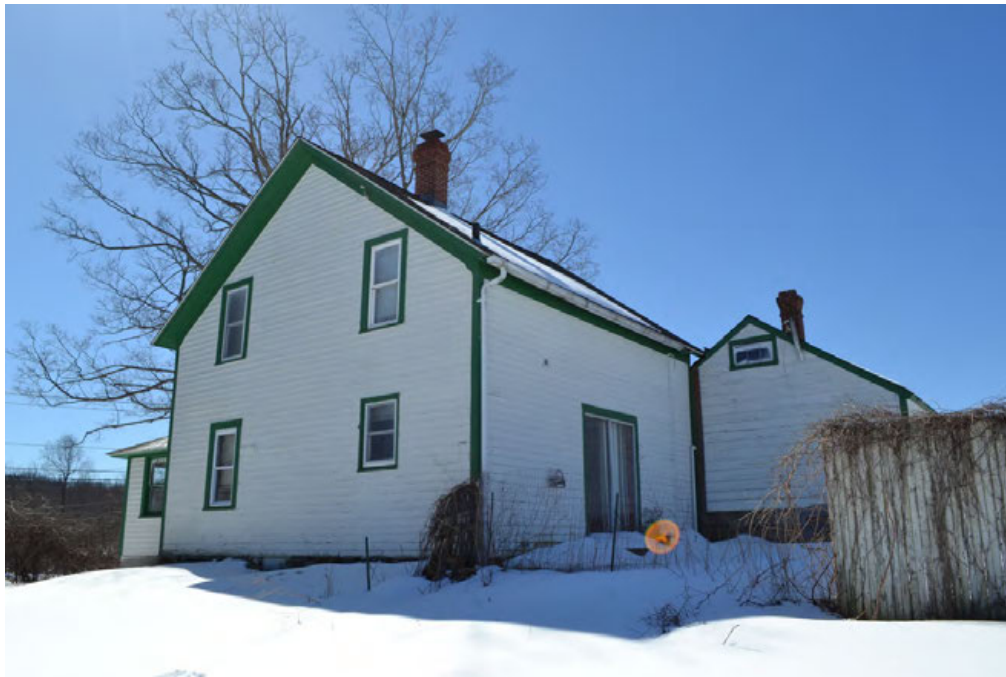
11. East gable-ends and north eave-sides of Farmhouse and side ell, camera facing southwest.
