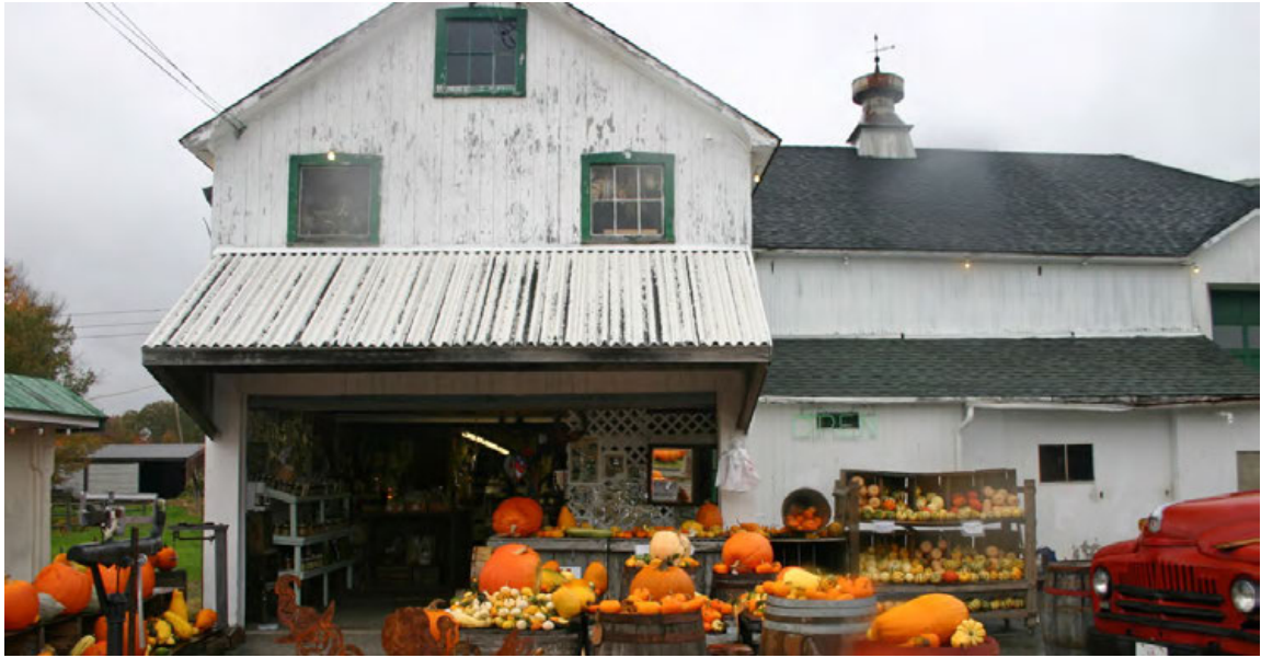
19. South gable-end and south eave-side of the Cider mill, camera facing north, showing entry to retail store.
