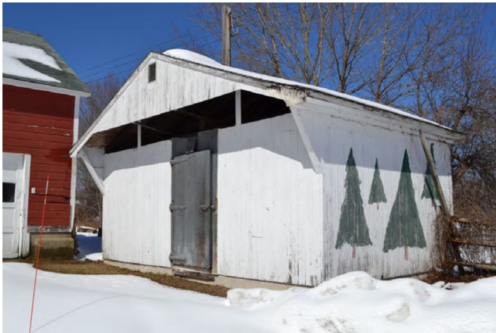
18. East eave-side and south gable-end of the Apple Storage Shed, camera facing northwest. Note insulated access door and overhanging roof.
