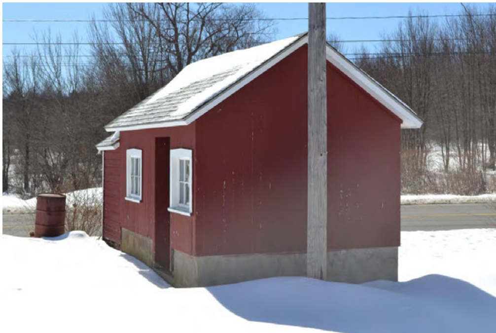
16. East eave-side and north gable-end of Milk house, camera facing southwest. Note addition on south gable-end.
