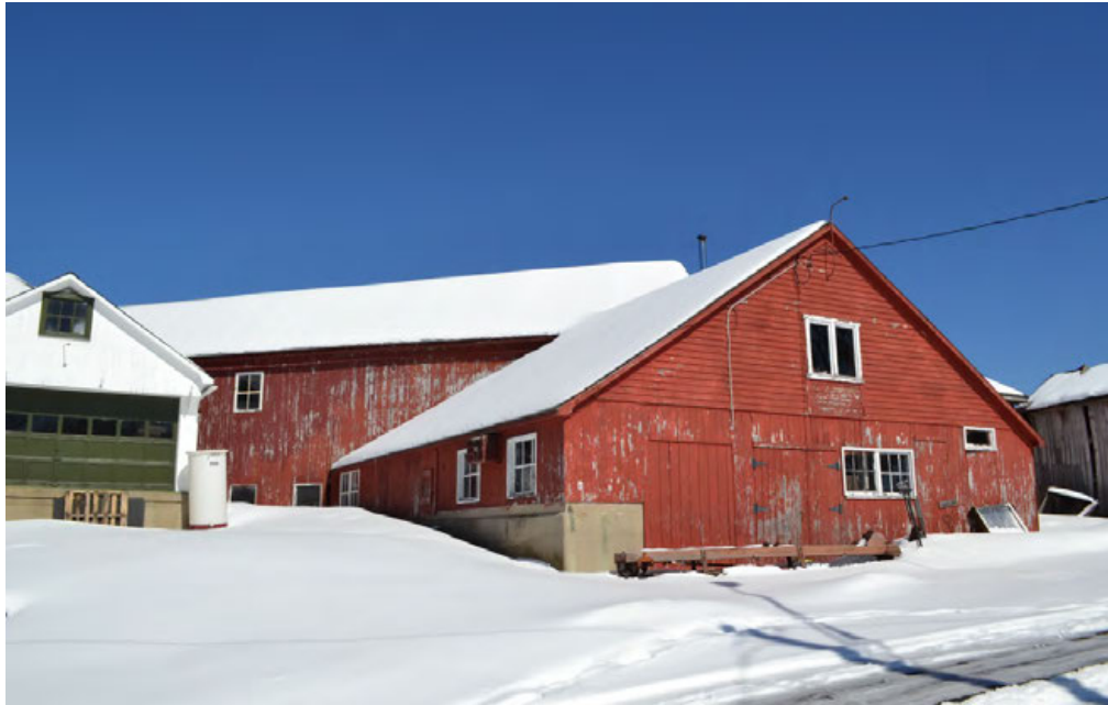
27. South gable-end and west eave-sides of Barn I, camera facing northeast.
