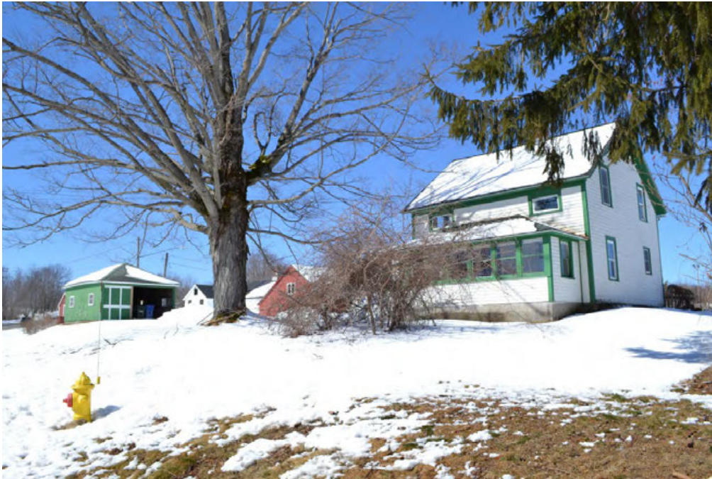
9. Southeast context view of 522 Spielman Highway, Burlington, CT, camera facing northwest. From left to right, Garage I, Cider mill, Barn I, Farmhouse.
