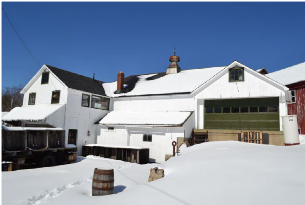
20. South gable-ends and south eave-side of the Cider mill, camera facing northwest.
