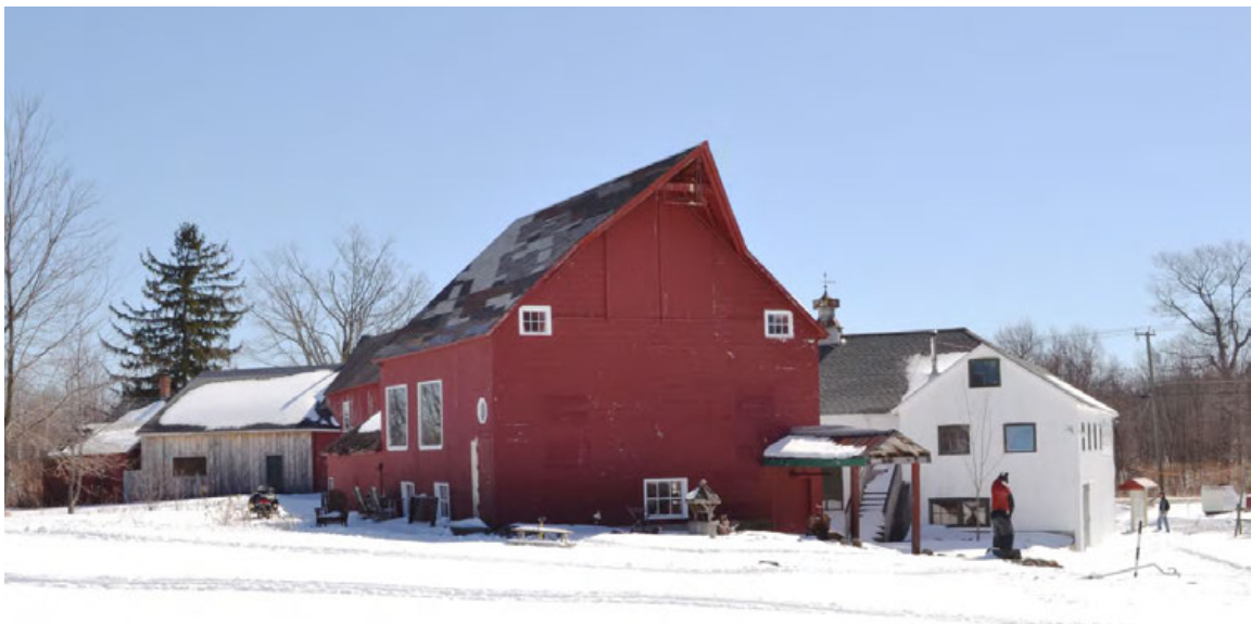
30. North eave-side and west gable-end of Barn I, camera facing east.
