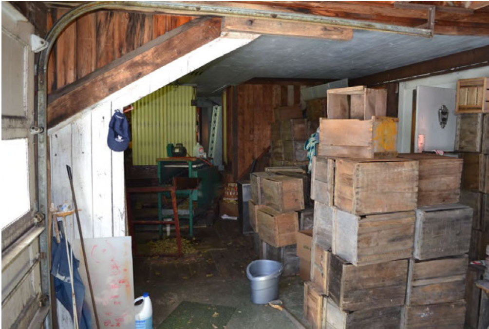
25. Interior of the Cider mill upper level, showing details of central block, camera facing west. Note eastern block roll-up garage-style door at far left, apple mill at center left, and refrigerated storage at far right.
