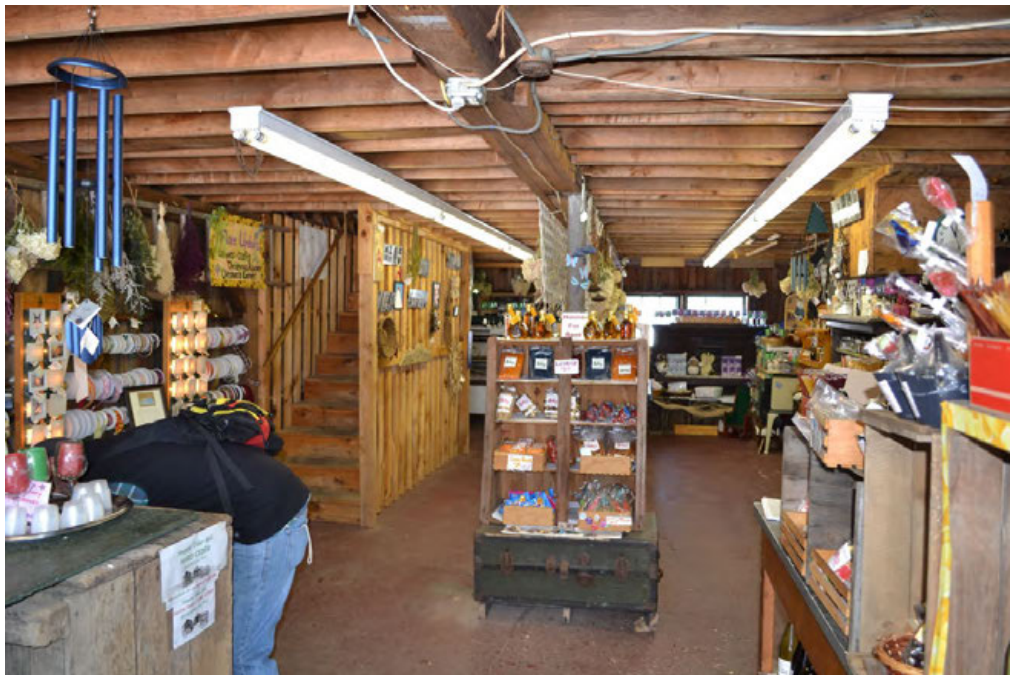
22. Interior of the Cider mill ground level, showing floor and framing details of western block, camera facing north. Note stair at left.
