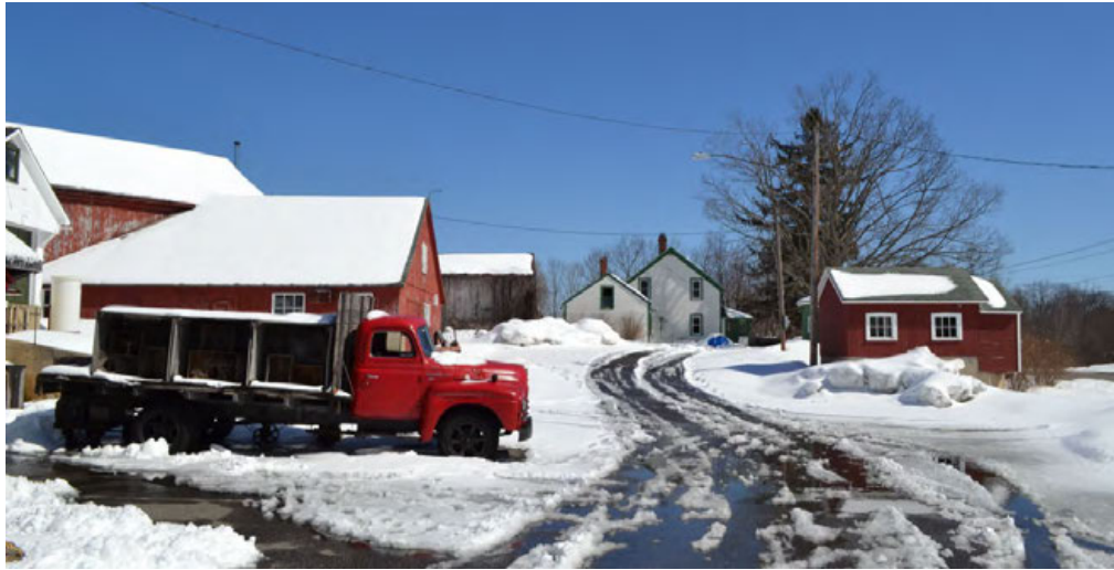
7. West context view of 522 Spielman Highway, Burlington, CT, camera facing east. From left to right, Cider mill, Barn I, Barn II, Farmhouse, Milk house.
