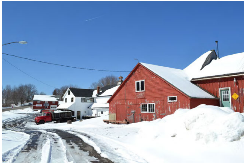
8. East context view of 522 Spielman Highway, Burlington, CT, camera facing west. From left to right, Garage II, Cider mill, Barn I.
