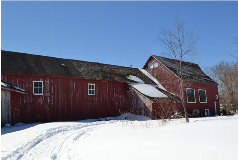
31. North eave-sides and east gable-ends of Barn I, camera facing southwest.
