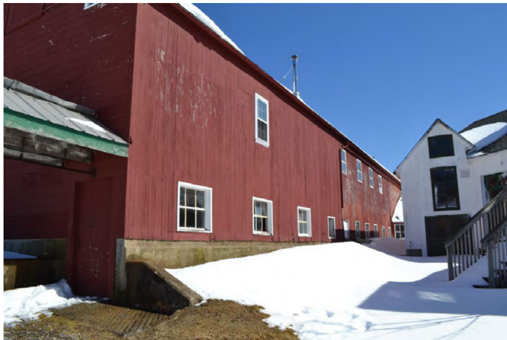
28. South eave-side and west gable-end of Barn I, camera facing northeast.
