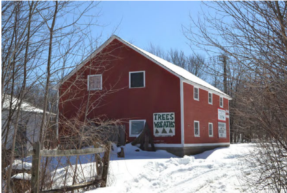
17. West eave-side and north gable-end of Garage II, camera facing south.
