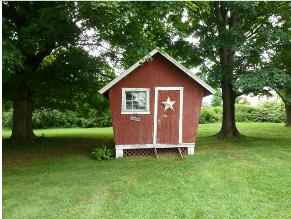
11. South gable-end of the Corn crib, camera facing north.
