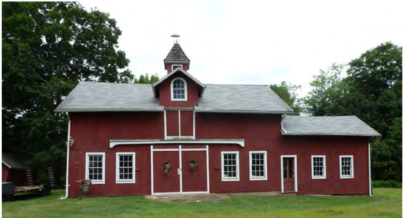
12. South eave-side (main façade) of the English barn and Addition I on the east, camera facing north.
