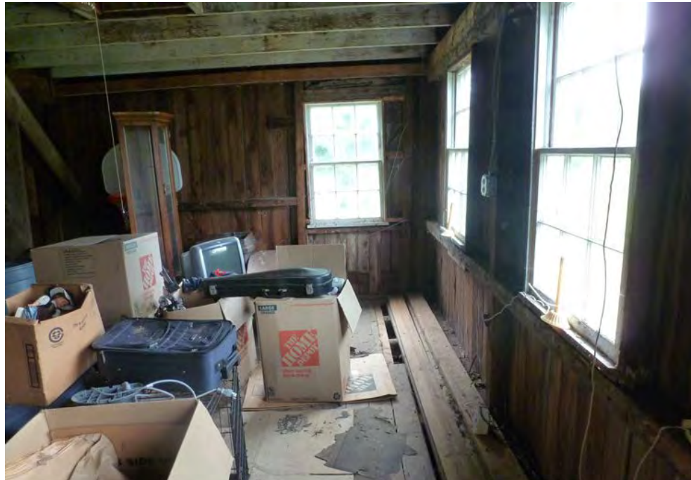
28. Interior view of the first floor of Addition I, camera facing east.
