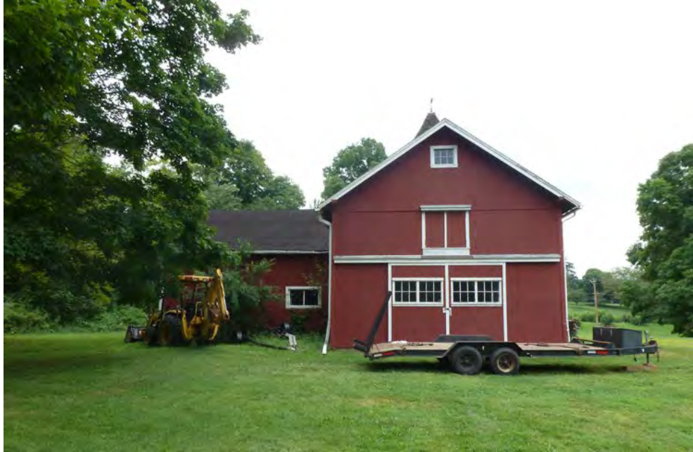
17. West eave-side of Addition III and west gable-end of the barn, camera facing east.
