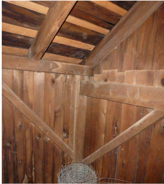
25. Interior view of the second floor northeast corner of the barn, note the post-and-beam framing. Camera facing northeast.
