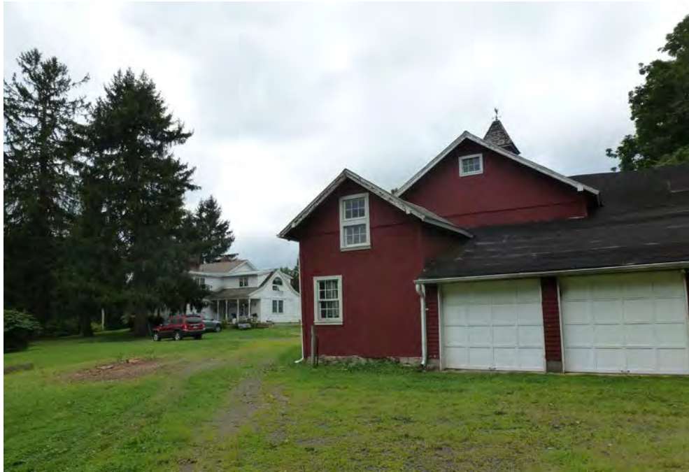
5. Northeast context view of Barn and Farmhouse, camera facing southwest.
