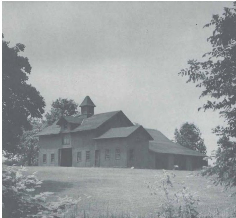
42. Southeast view of the barn and additions, c. 1979. Camera facing northwest. (Klamkin, p. 38).
