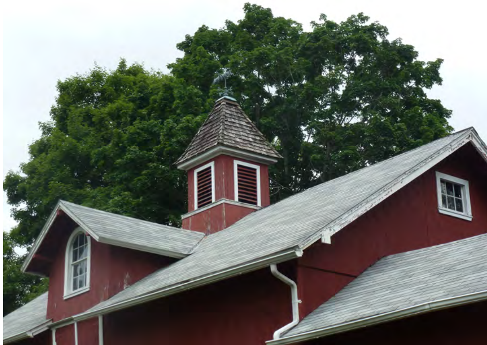
18. Detail view of the gable roof-dormer and the cupola, camera facing northwest.
