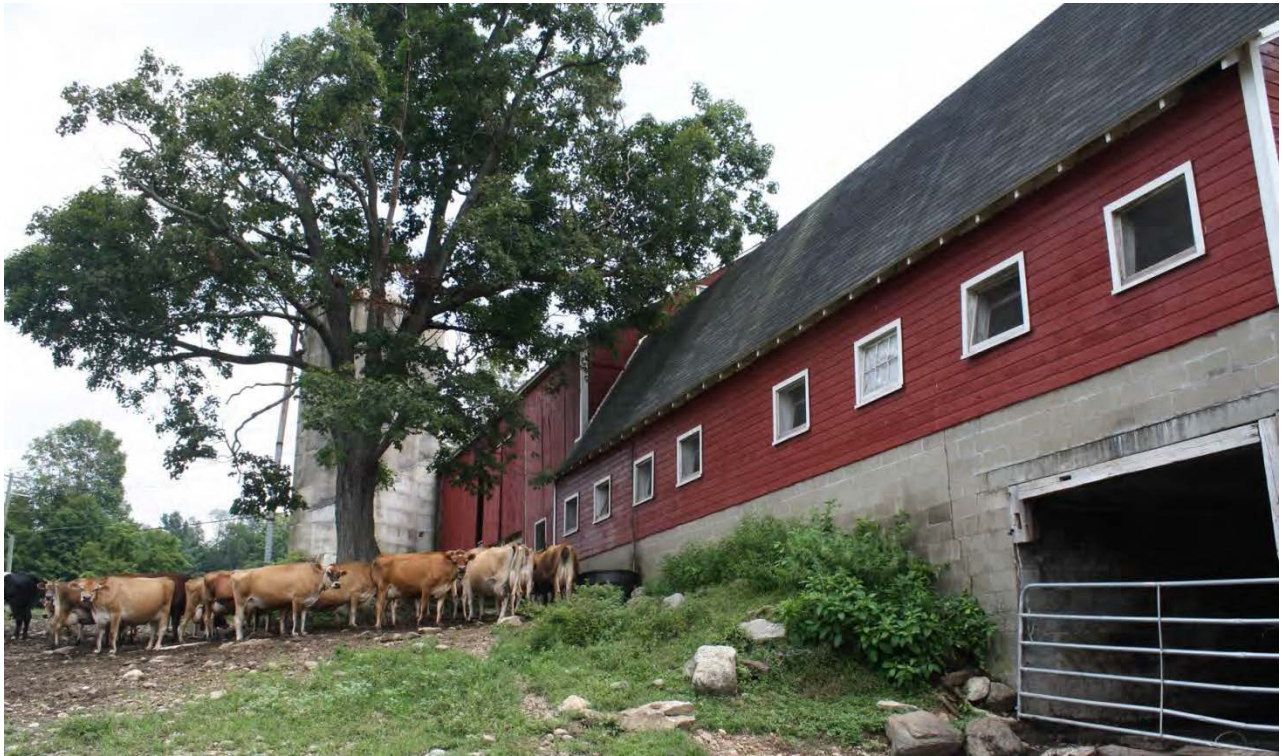
11. Southwest view of Barn I, camera facing northeast. The silo and main block are at left rear. In the foreground is Addition I (gambrel stable barn). At right is the manure-loading bay in the lower basement.
