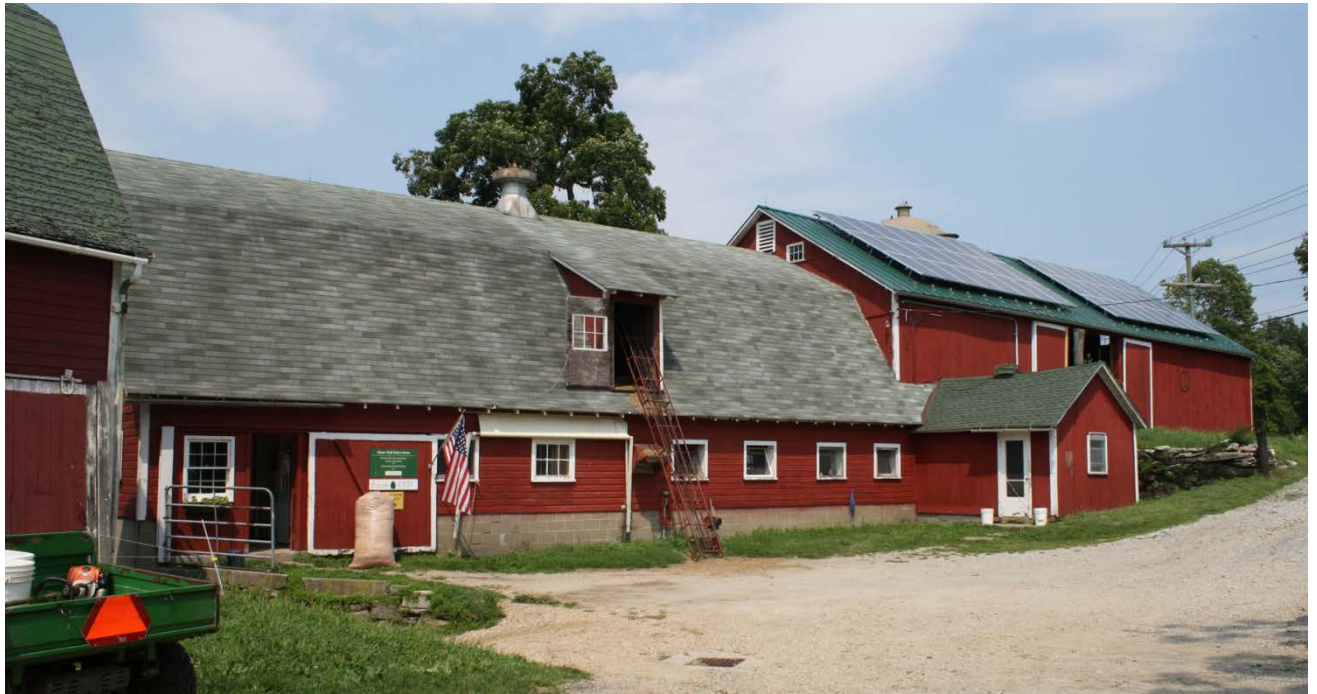
13. Southeast view of Barn I Addition I, camera facing northwest. Addition II (milk room) and main block at right.
