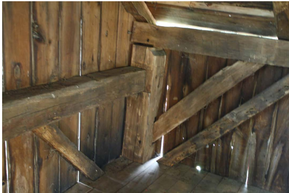
32. Interior view of Barn III, camera facing northwest, showing square rule framing and dropped girt.
