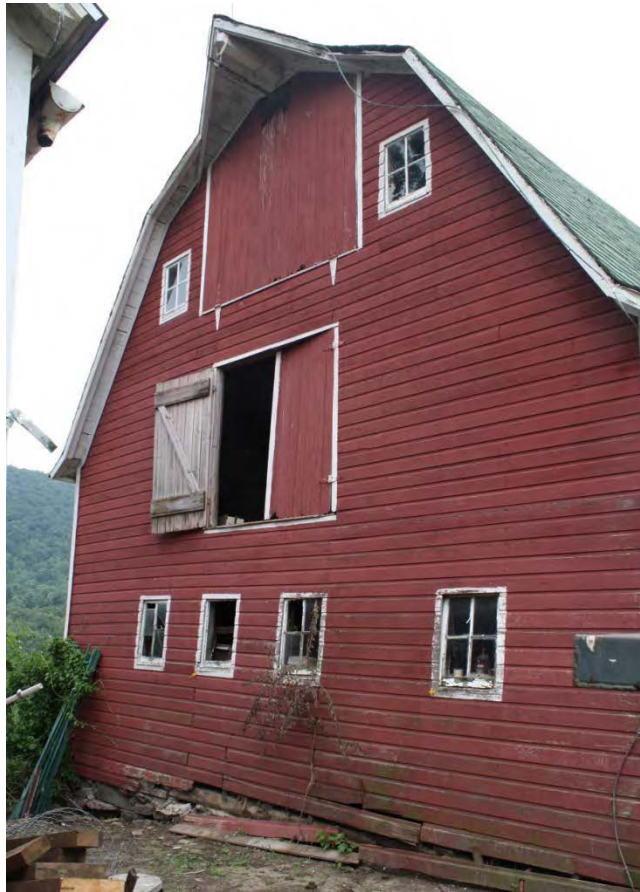
25. South view of Barn II, camera facing northwest. Note the out-swinging bottom-hinged upper hay door.
