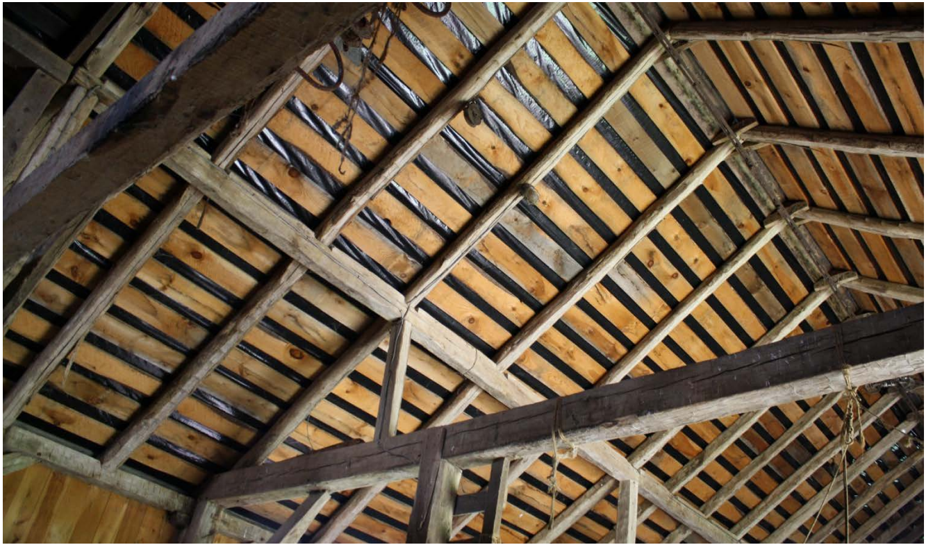
19. Interior view of Barn I main block, camera facing north, showing roof construction with purlin plate, hewn common rafters, and hay track. Purlin plates and queen posts are set closer to the outer walls than is typical.
