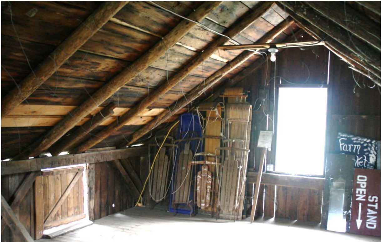
31. Interior view of Barn III, camera facing northeast, showing pole rafters and square rule framing.
