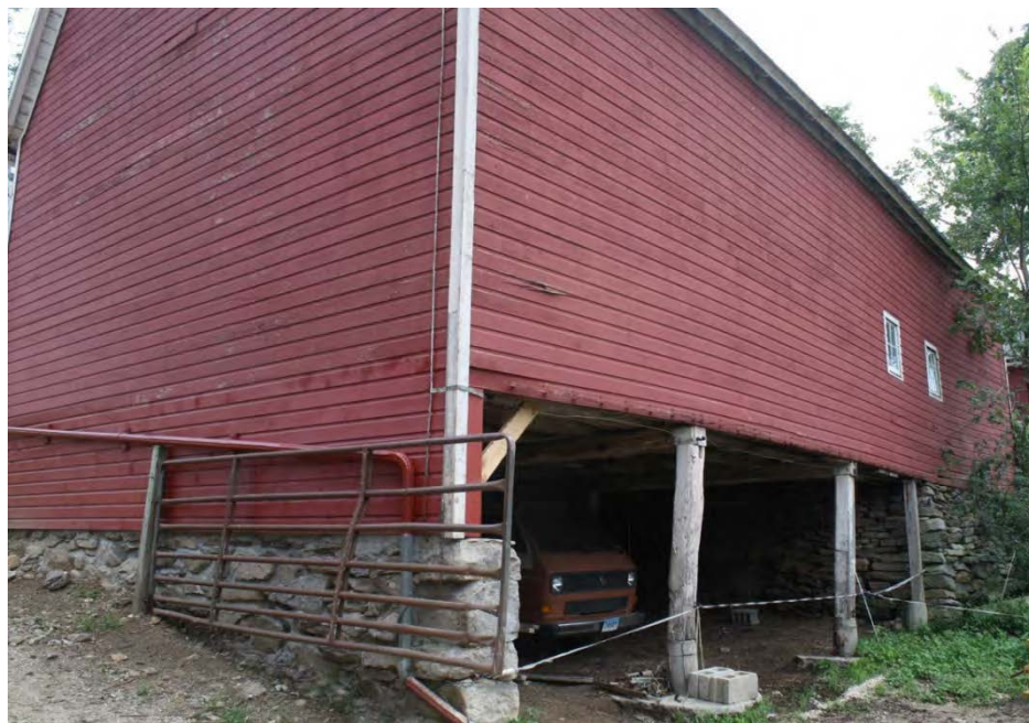
24. Northwest view of Barn II, camera facing southeast, showing banked north bays and fieldstone foundation of the south bay.
