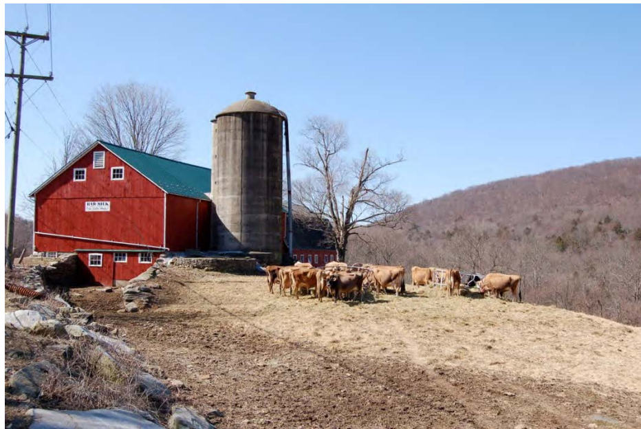
34. Northwest view of Barn I, camera facing southeast, with dairy herd. Note foundation of former silo.
