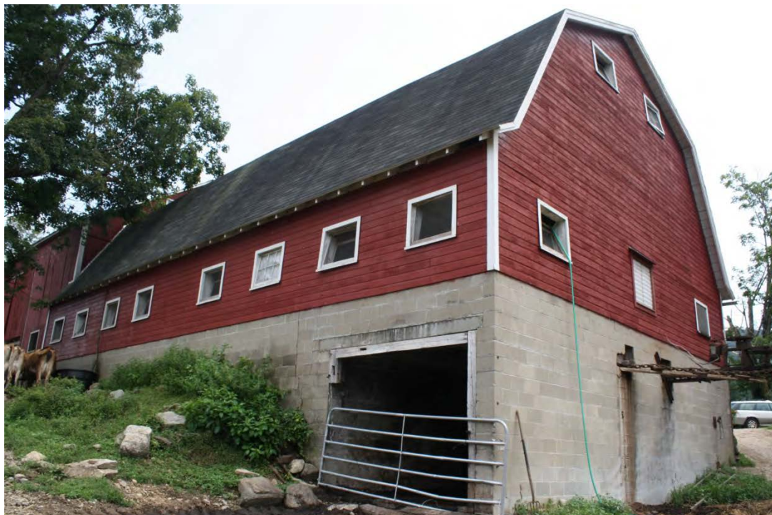
12. Southwest view of Barn I Addition I, camera facing northeast. Protruding from the south gable-end at right is the manure gutter scraping mechanism.
