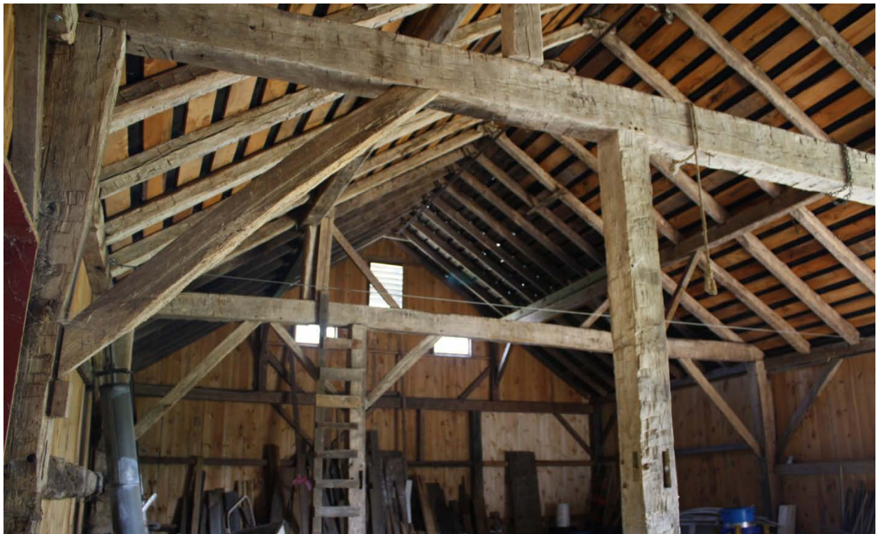
14. Interior view of Barn I main block, camera facing north from the center threshing bay, showing scribe rule framing of the central bays, and square rule framing of the north bay at rear.
