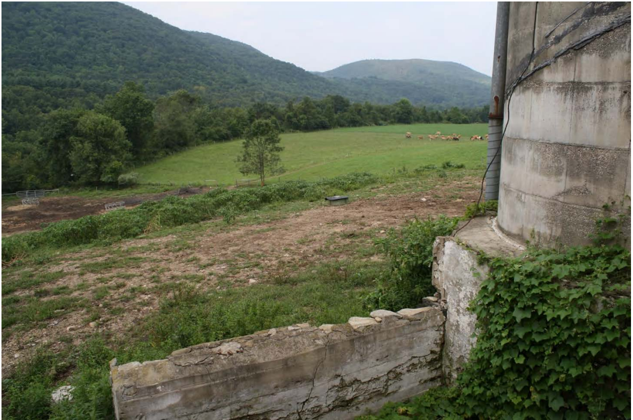
33. View of silo base and cow pasture, camera facing north. Housatonic River runs beyond the trees at left.
