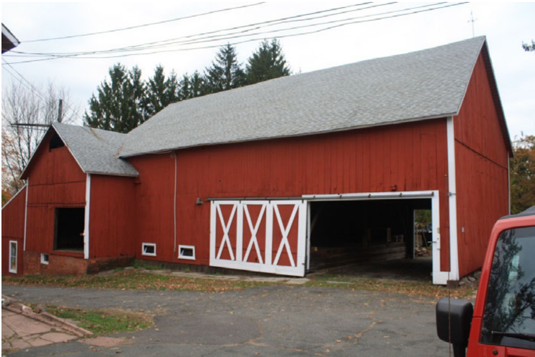
20. South view of the Barn, camera facing north. The original main block at left has a brick foundation.
