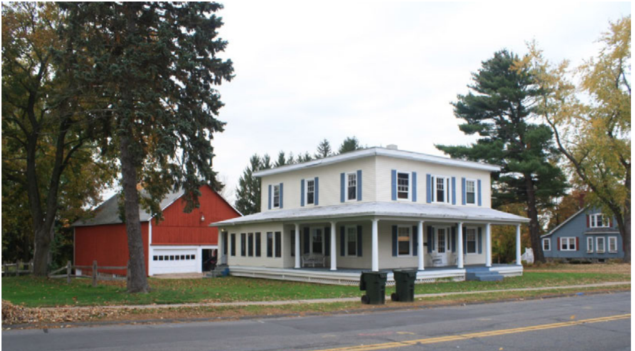
6. Southeast view of the Farmhouse and Tobacco shed behind, camera facing northwest.
