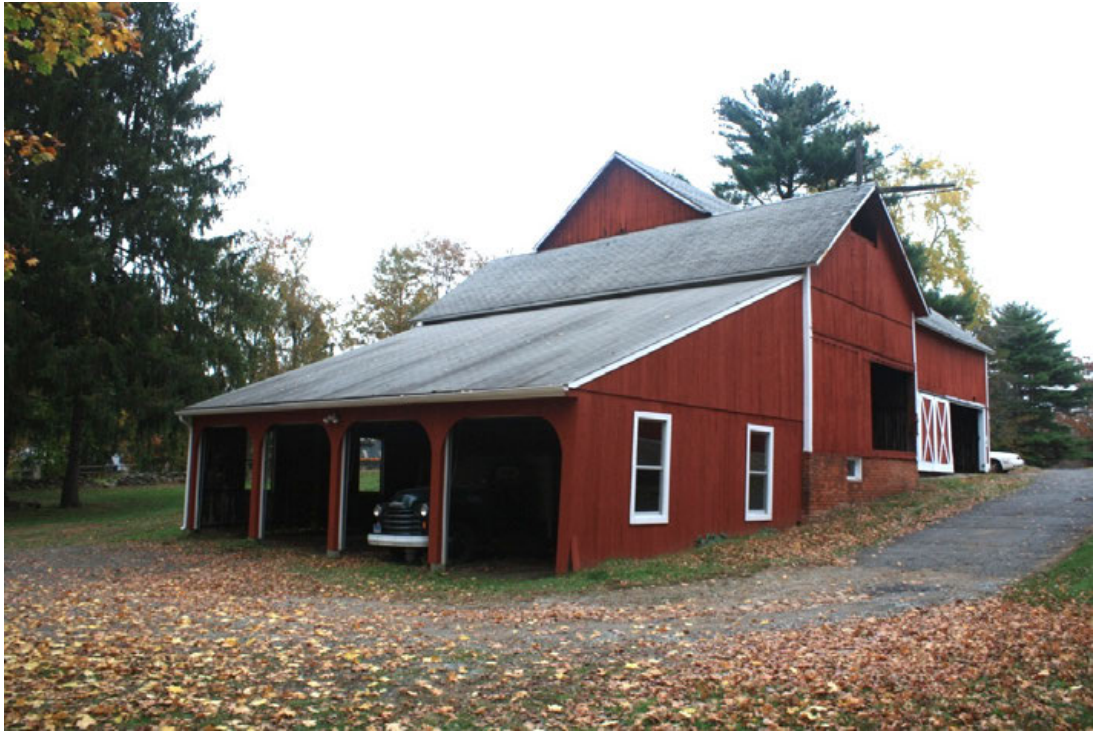
21. Southwest view of the Barn, camera facing northeast. Far left bay of the shed addition provided access to the basement dairy stable area.
