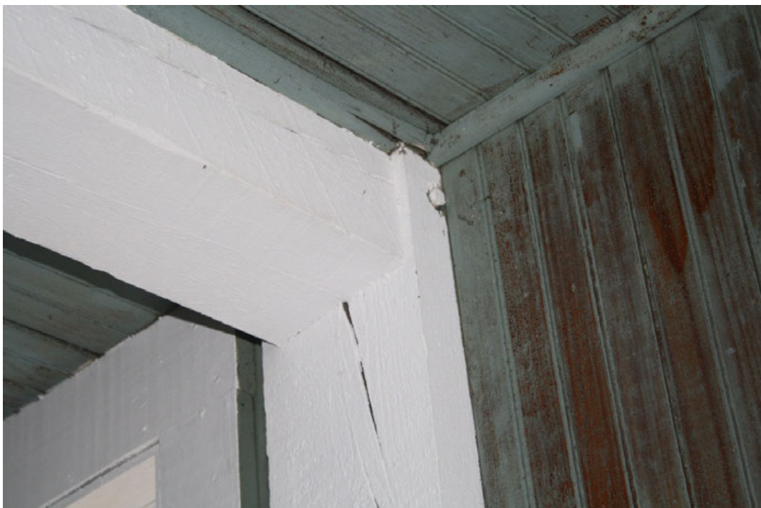
14. Detail of the interior of the Tobacco shed, square rule construction, camera facing northwest.
