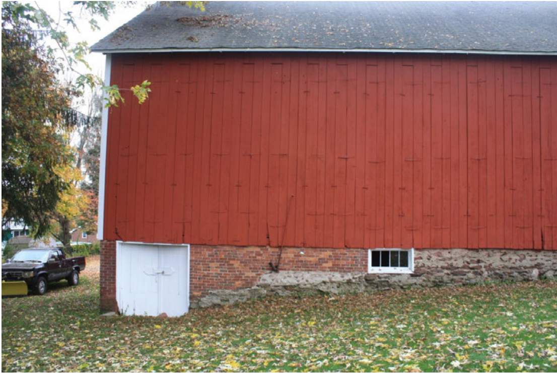
9. South eave-side of the Tobacco shed, camera facing north. Note the change in foundation materials.
