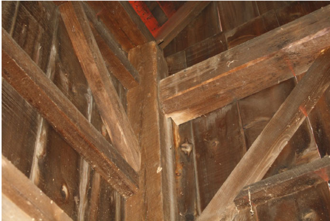
17. Detail of the interior of the Tobacco shed main level, square rule construction, camera facing southeast.
