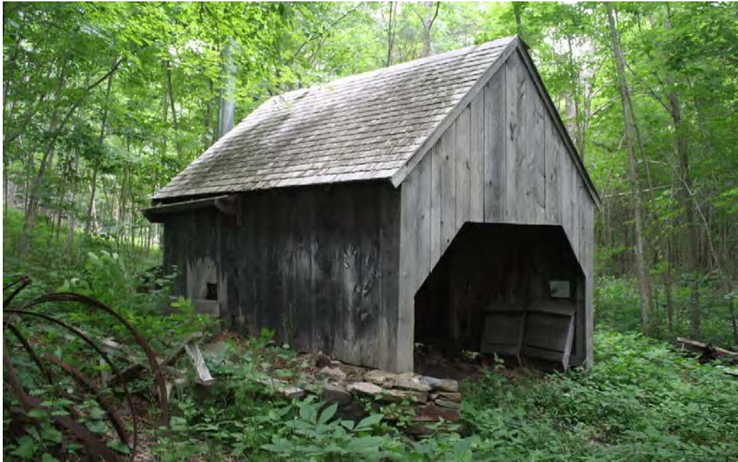
17. West view of Sugar house, camera facing east.
