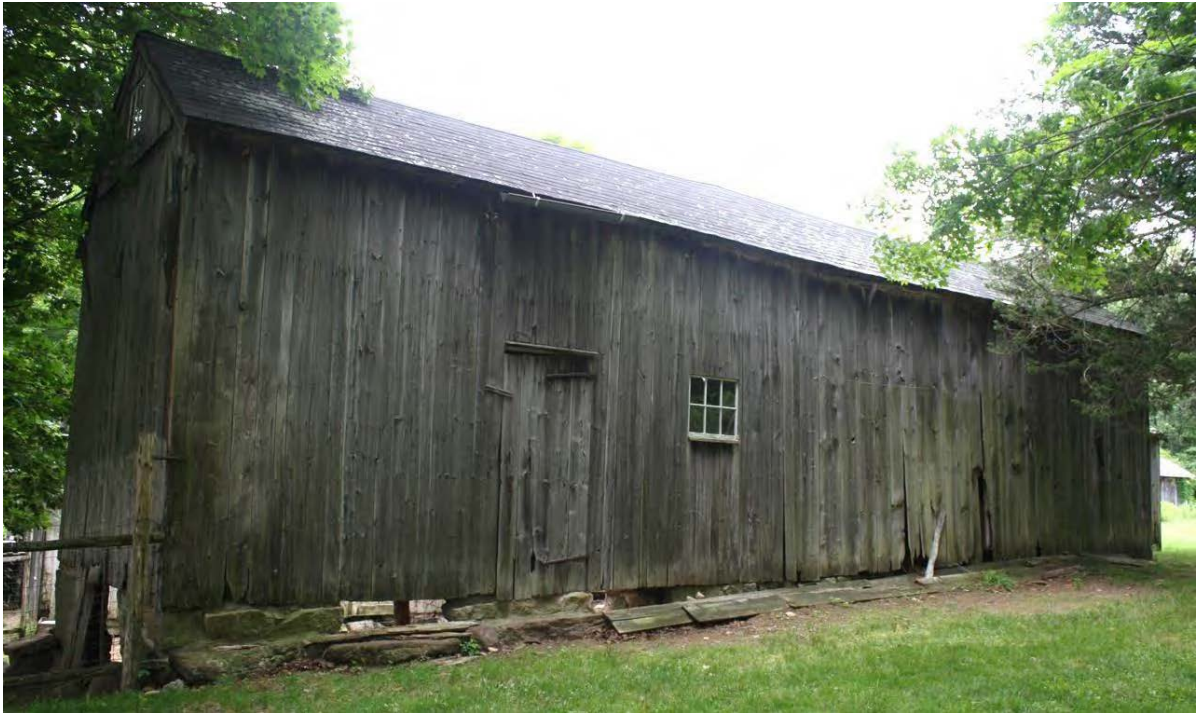
25. Southeast view of Barn II, camera facing northwest.
