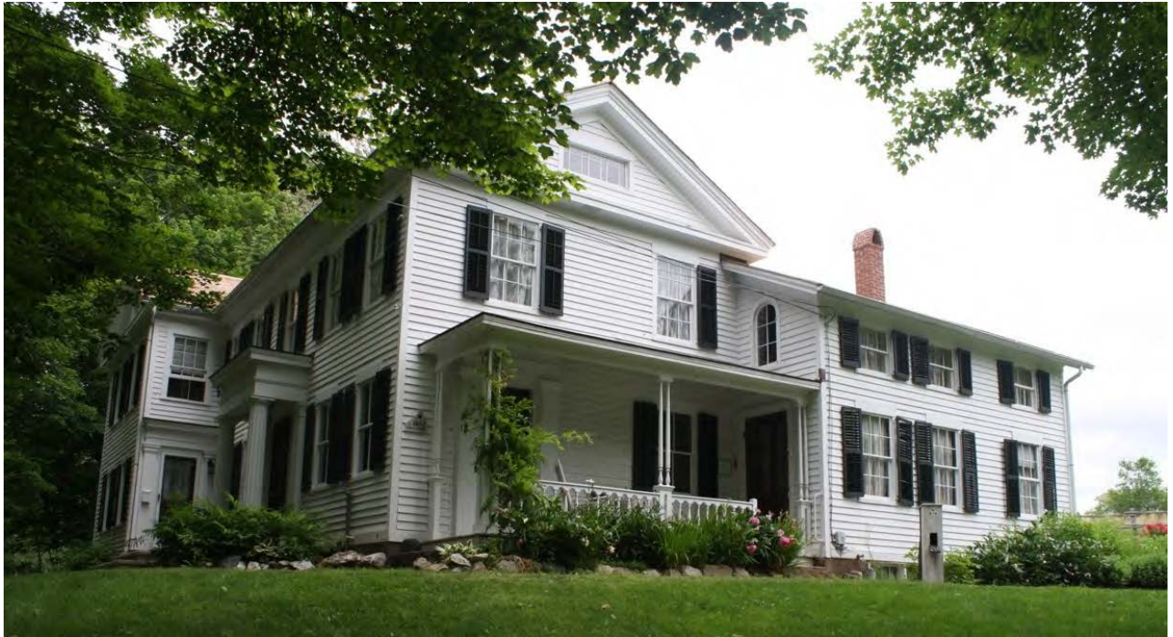
5. Southwest view of Farmhouse, camera facing northeast.
