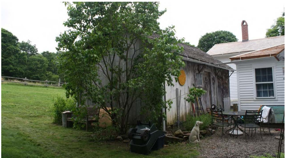
9. Northwest view of Shed III, camera facing southeast.
