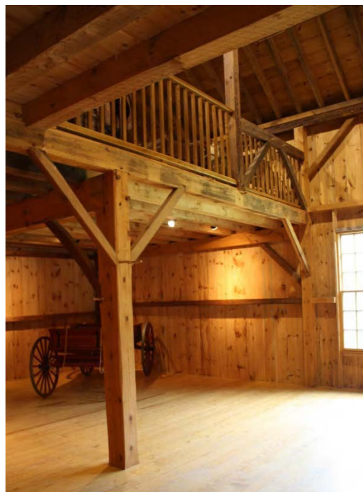
32. Interior view of Barn III main level, camera facing southeast.
