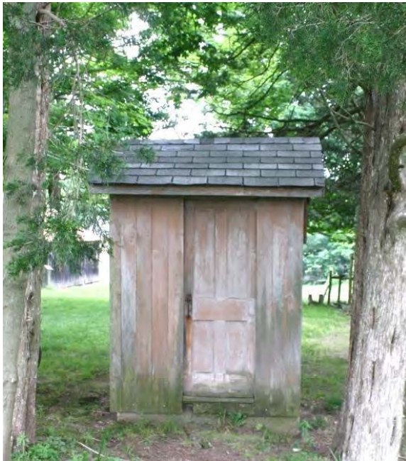
12. North view of Outhouse.
