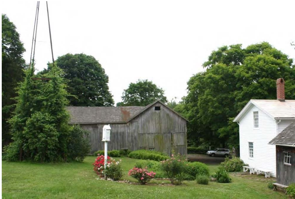
10. North view of Barn I with Windmill base at left and rear wing of Farmhouse at right, camera facing south.
