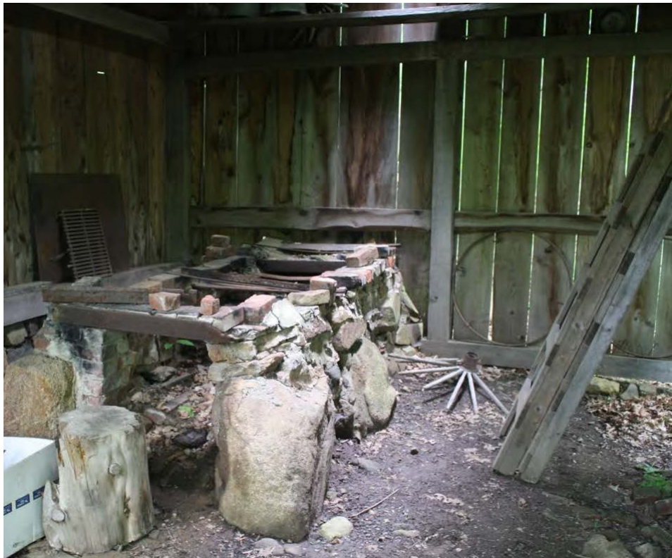
18. Interior view of Sugar house showing firebox, camera facing north
