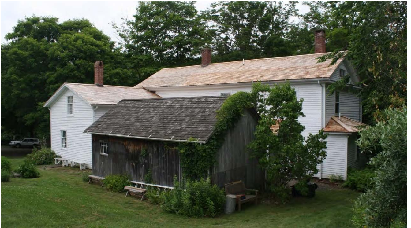
8. Northeast view of Farmhouse and Shed III, camera facing southwest.
