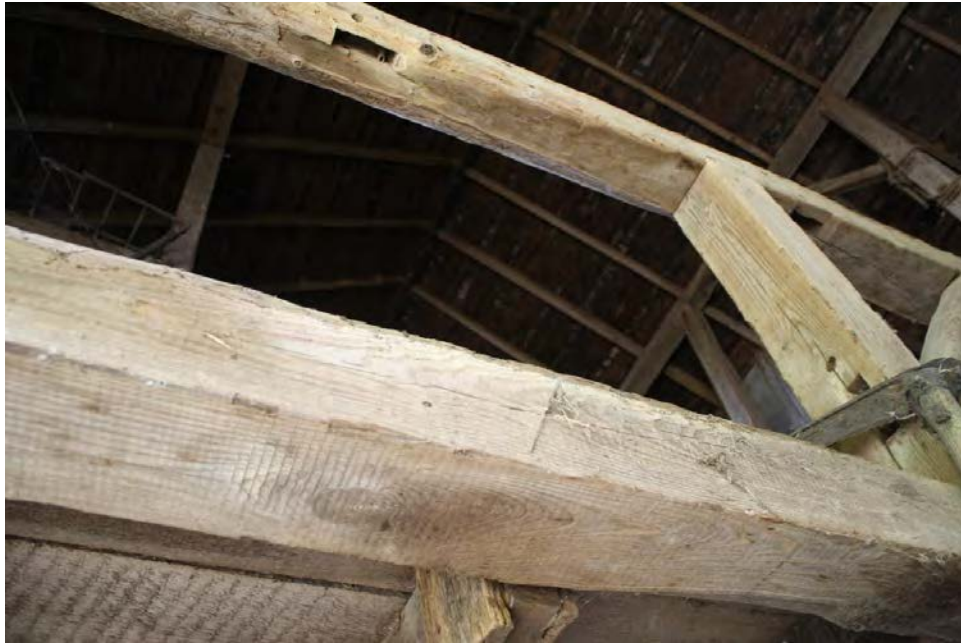
27. Interior view of Barn I, camera facing south from threshing bay. Note straight saw kerf marks on girt.
