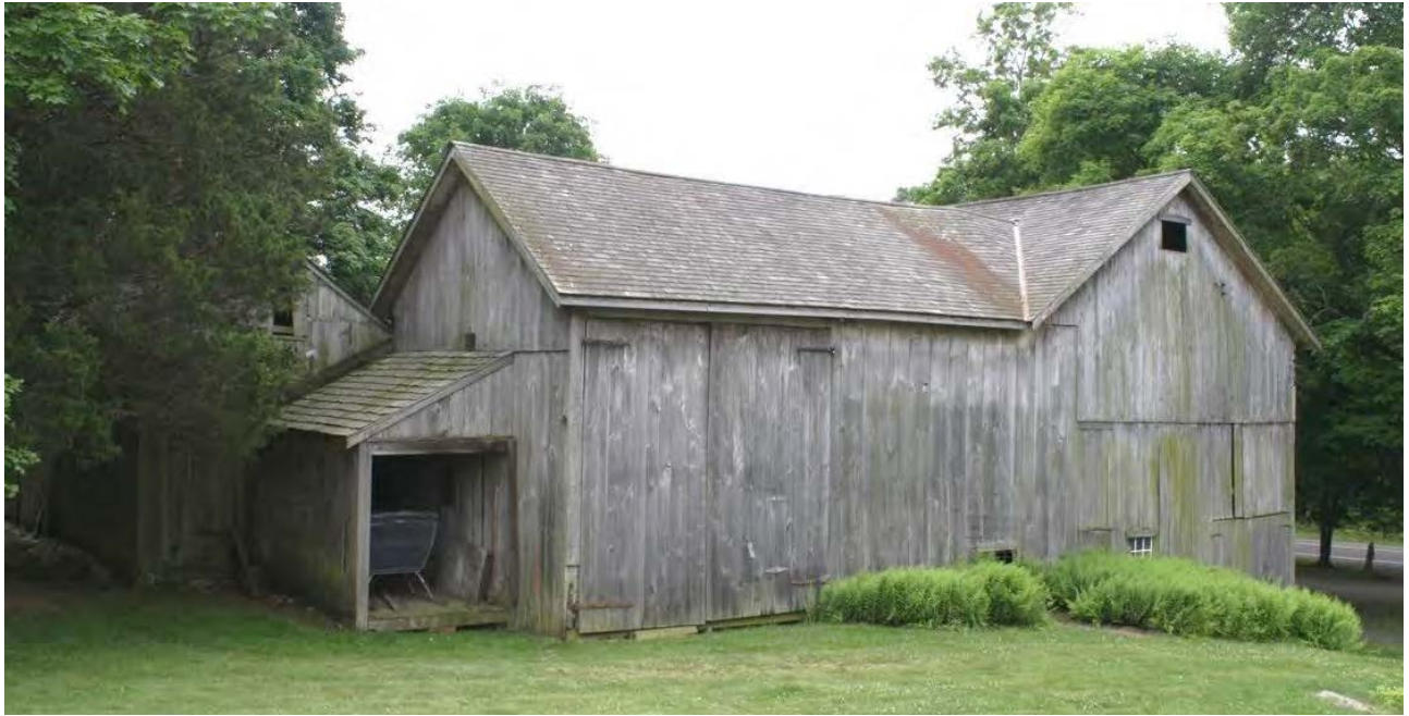
21. Northeast view of Barn I, camera facing southwest. Sleigh shed is at left.
