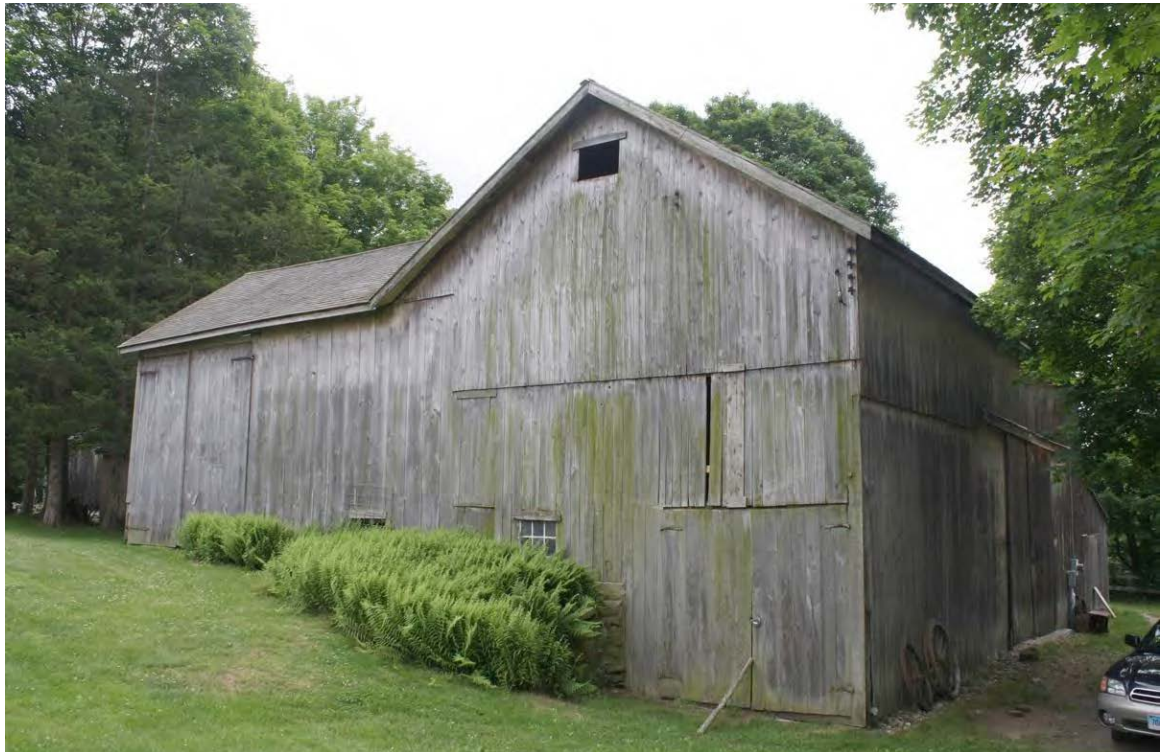
20. Northwest view of Barn I, camera facing southeast.
