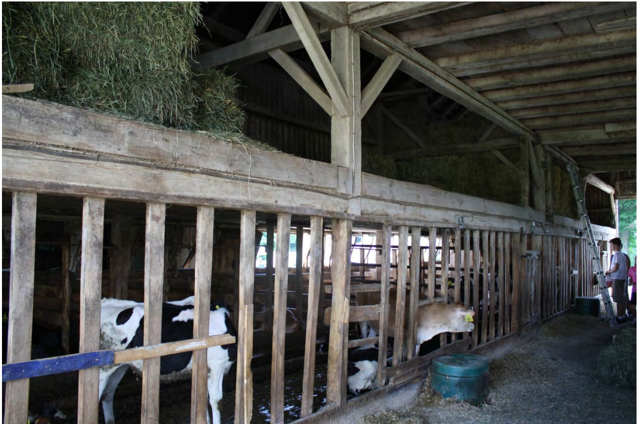
14. Interior view of Barn I, camera facing southwest, showing altered ground level stable area with truncated post timbers.
