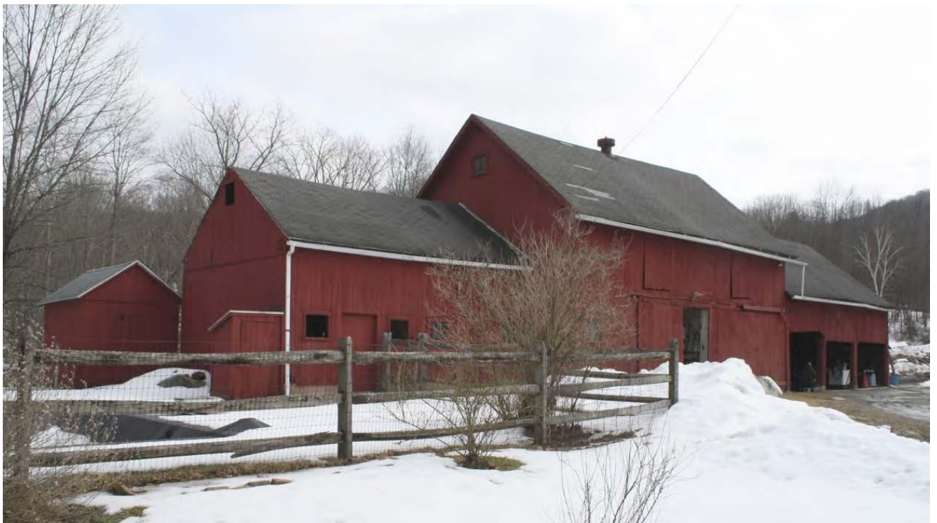
8. North view of Barn and Shed (at left), camera facing south.
