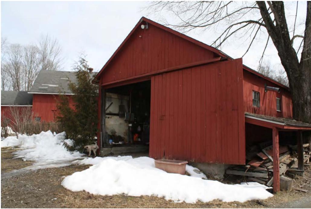
7. North view of Garage/workshop, camera facing south; Barn is visible at left rear.
