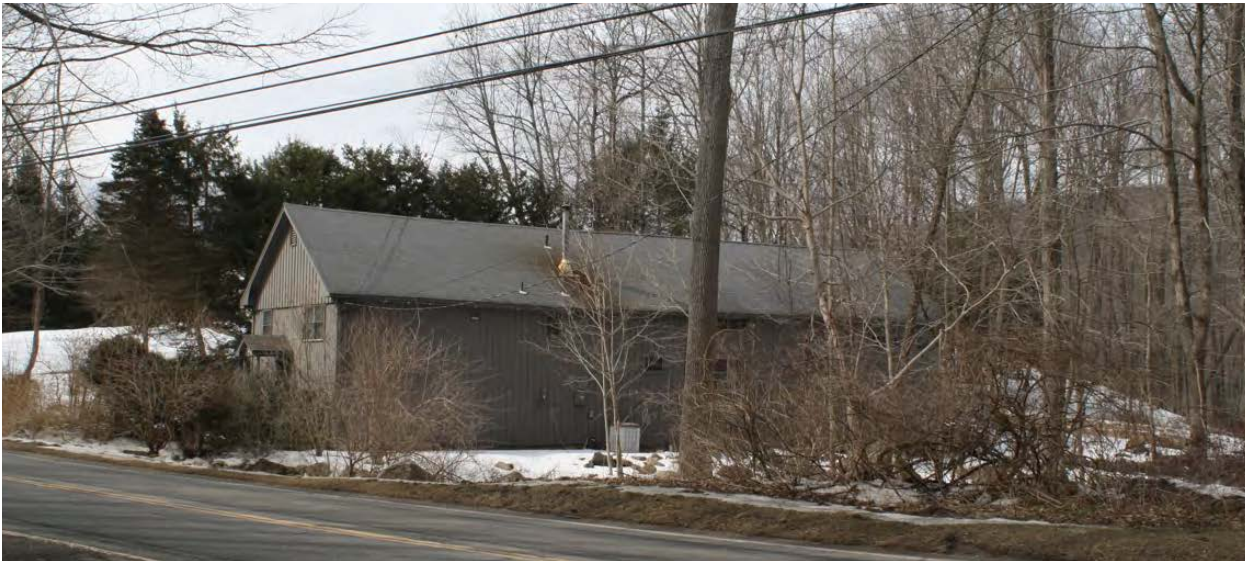
5. South view of former Tobacco barn, camera facing north; now converted to a residence under separate ownership.
