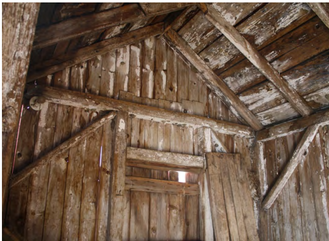
16. Interior view of Shed, camera facing west, showing timber framing.
