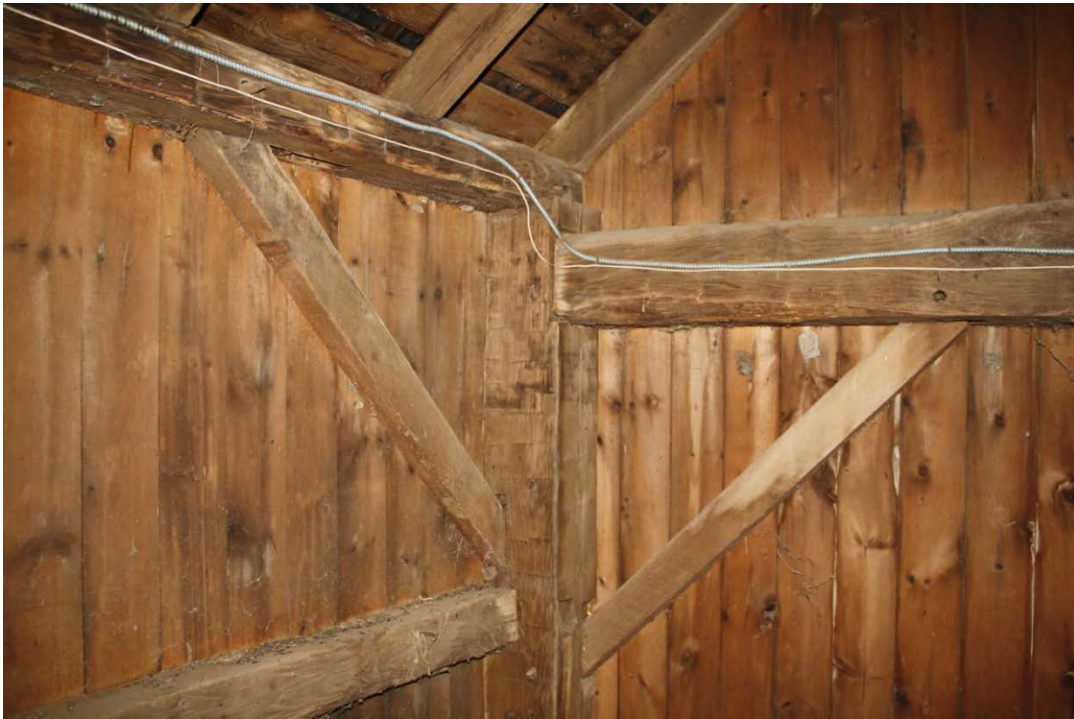
11. Interior view of Barn framing, camera facing north at northwest corner of loft level. Note hand-hewn timbers, dropped tie-girt detail.
