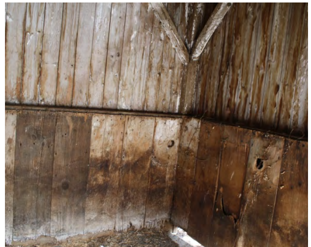
17. Interior view of Shed, camera facing northeast, showing board wainscoting.
