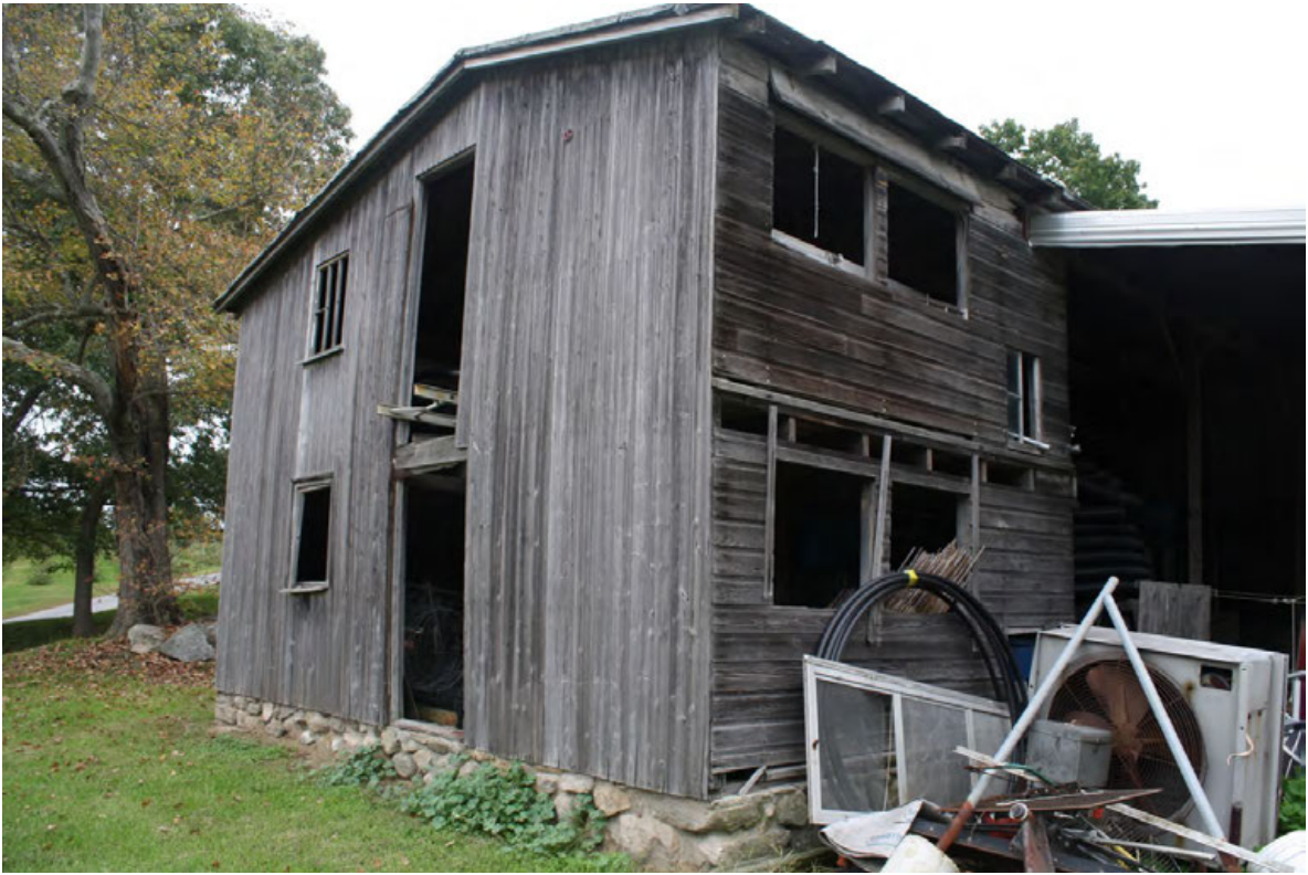
22. Southwest view of Coop II, camera facing northeast.
