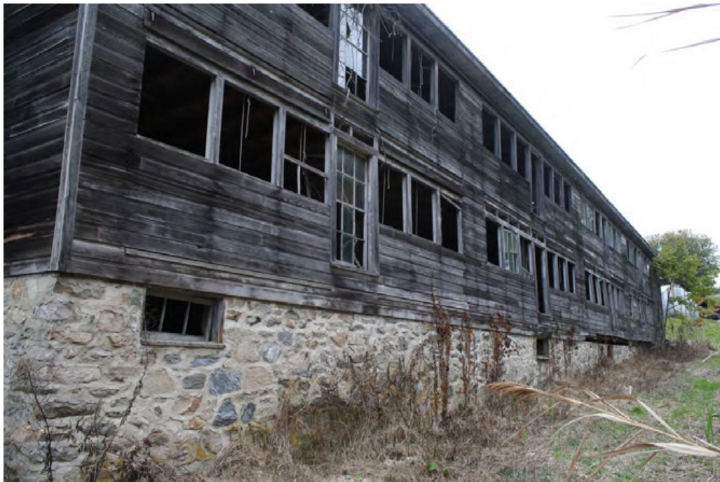
27. Southwest view of Coop III, south side; camera facing northeast.
