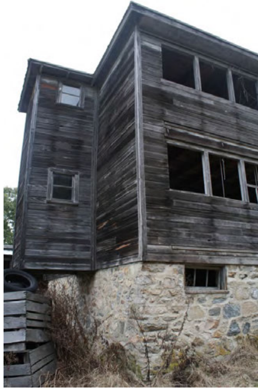
26. Southwest view of Coop III, west end; camera facing northeast.
