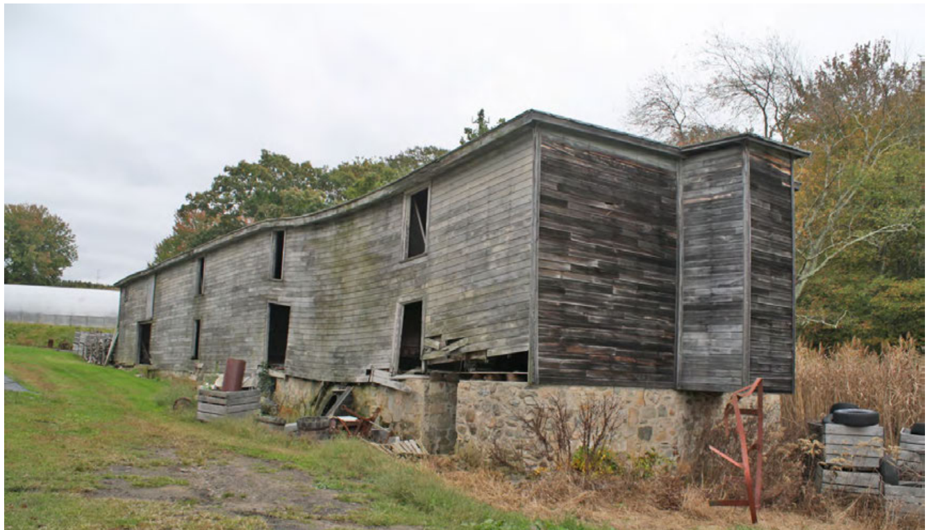
25. Northwest view of Barn II, camera facing southeast.
