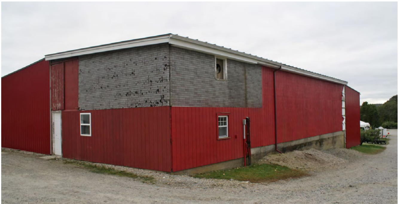
19. Northeast view of Coop I / Apple storage barn, camera facing southwest.
