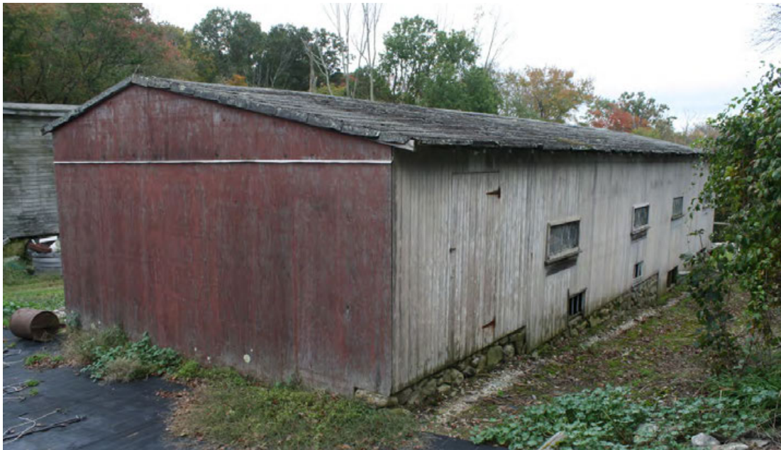
23. Northeast view of Coop II, camera facing southwest.
