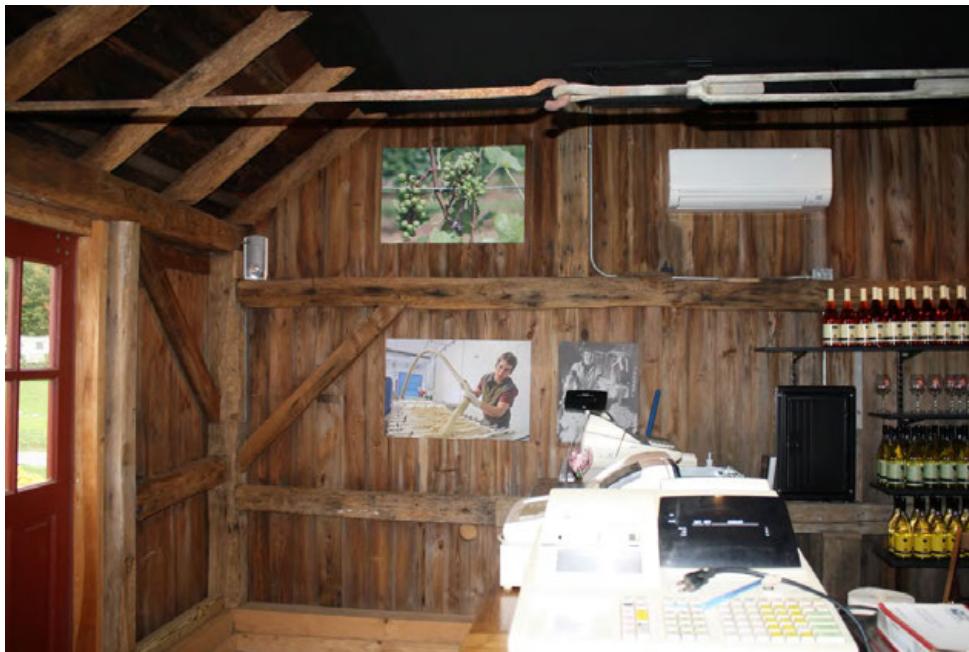
13. Interior view of Barn I, camera facing south.
