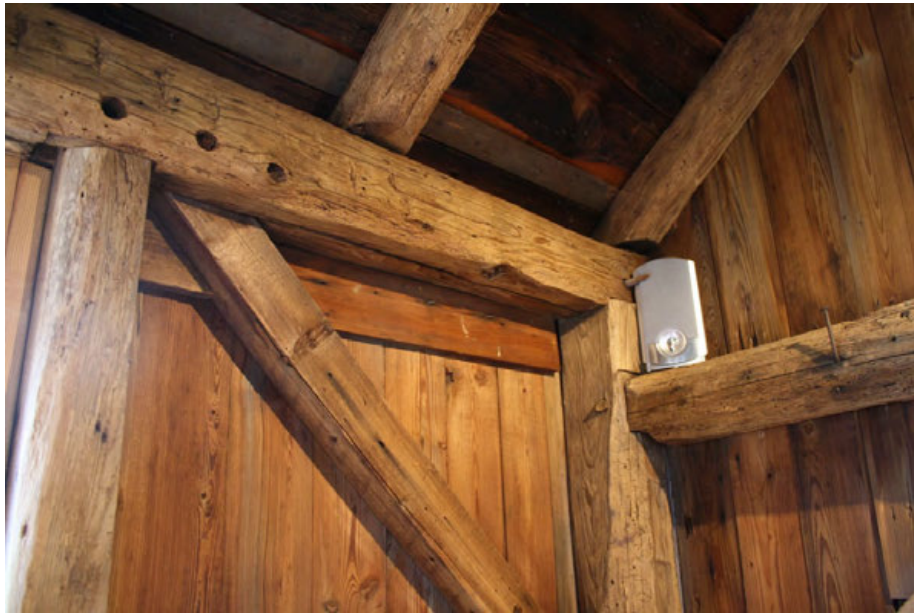
14. Interior detail view of Barn I framing, camera facing southeast.
