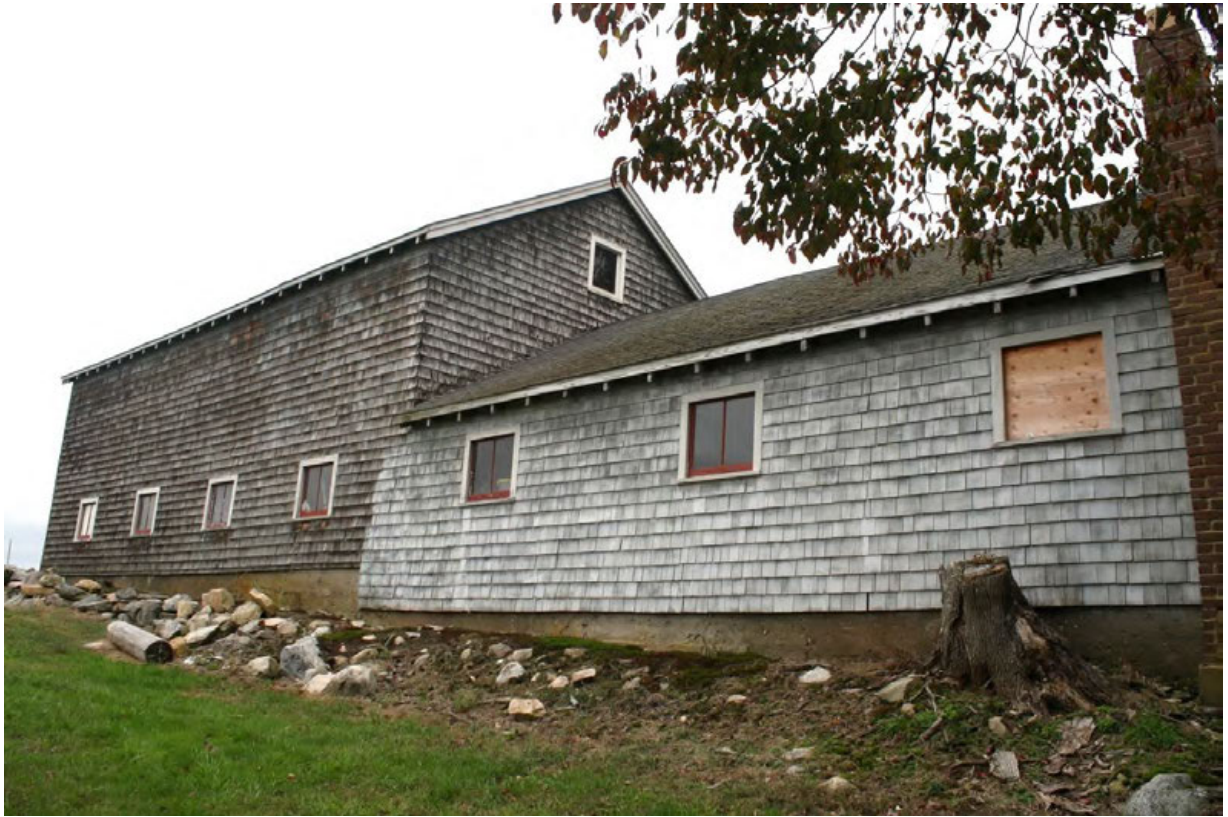
16. Southwest view of Barn II, camera facing northeast.
