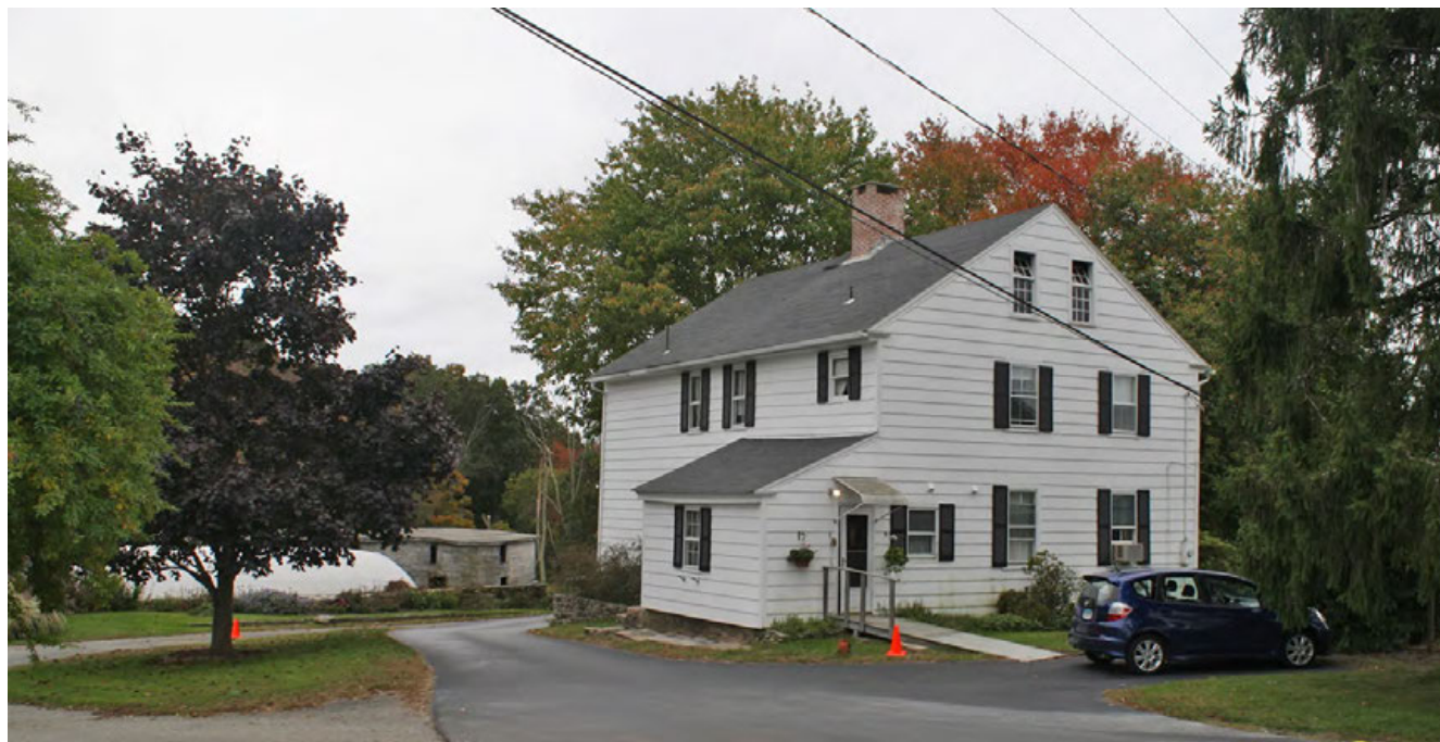
7. Northeast view of Farmhouse, camera facing southwest; Coop III at left rear. Note extant six-over-nine sash in attic windows, 19 th -century two-over-two sash at lower floors.
