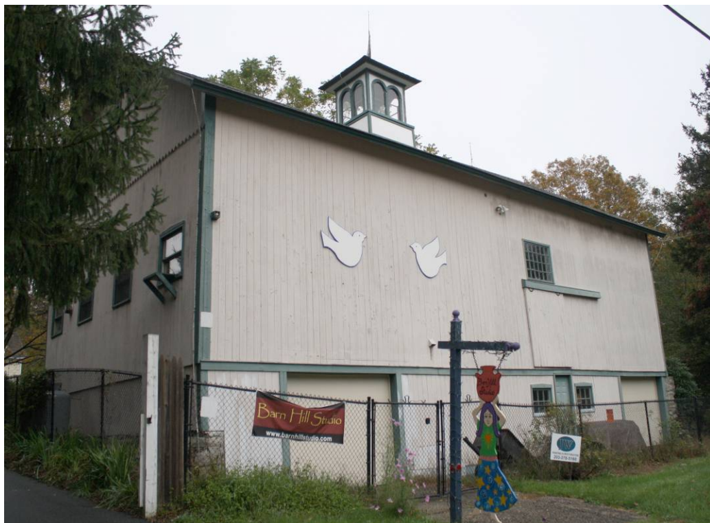
7. Southwest view, camera facing northeast.
