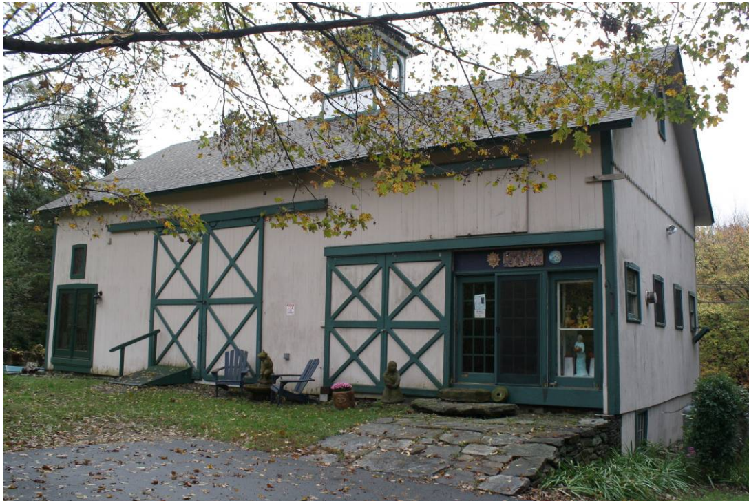
6. Northwest view, camera facing southeast.
