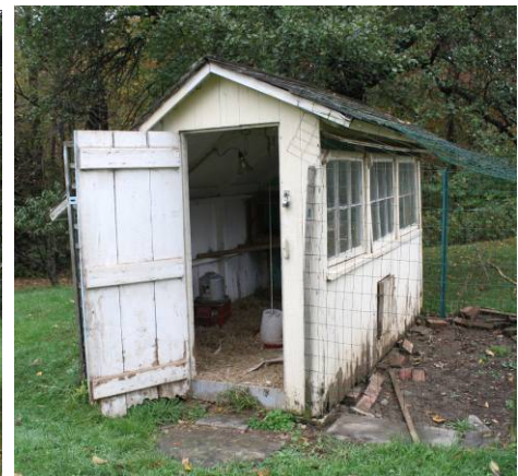
9b. Southwest view of coop.
