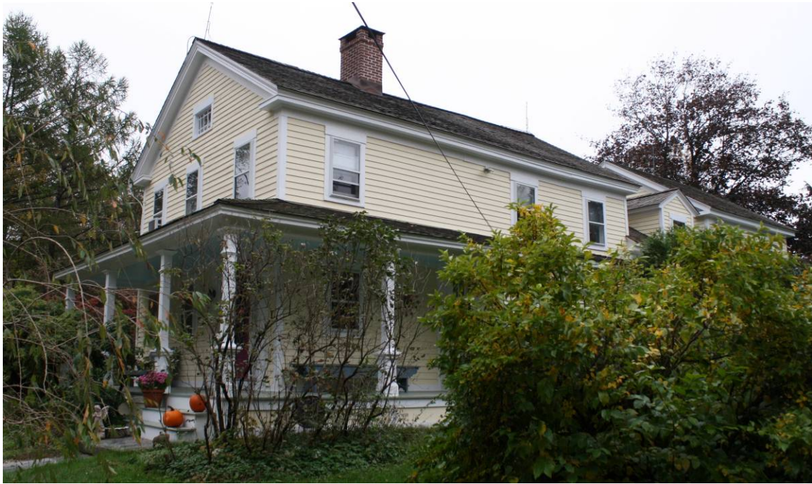
10. Northwest view of farmhouse, camera facing southeast.
