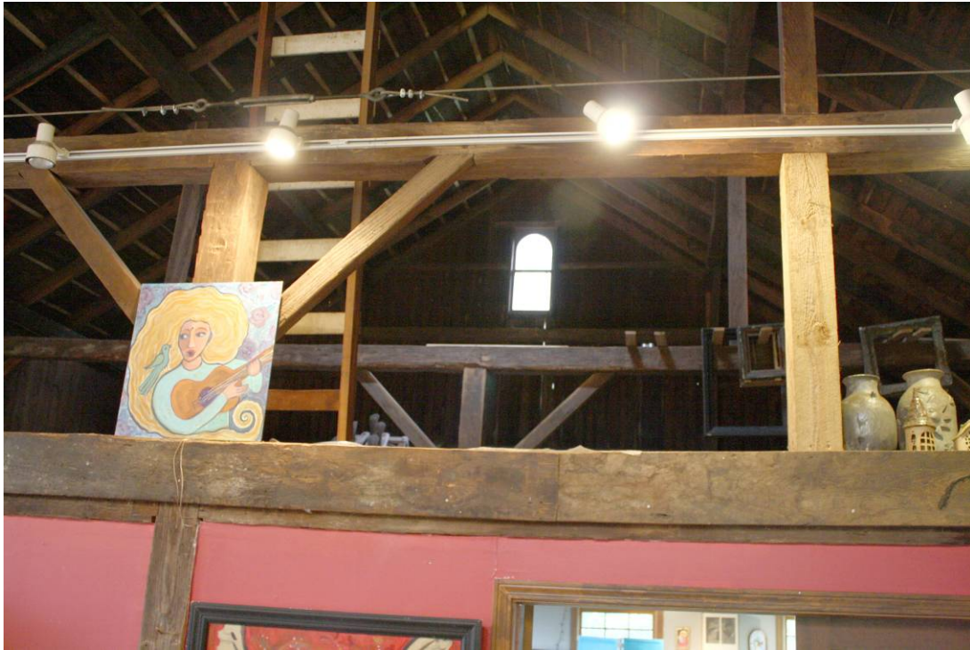
14. Interior of loft level, camera facing west.
