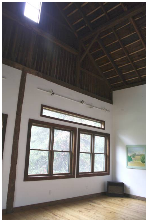
13a. Interior view of southeast corner.
