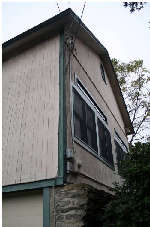
12b. Southeast corner detail, camera facing north.
