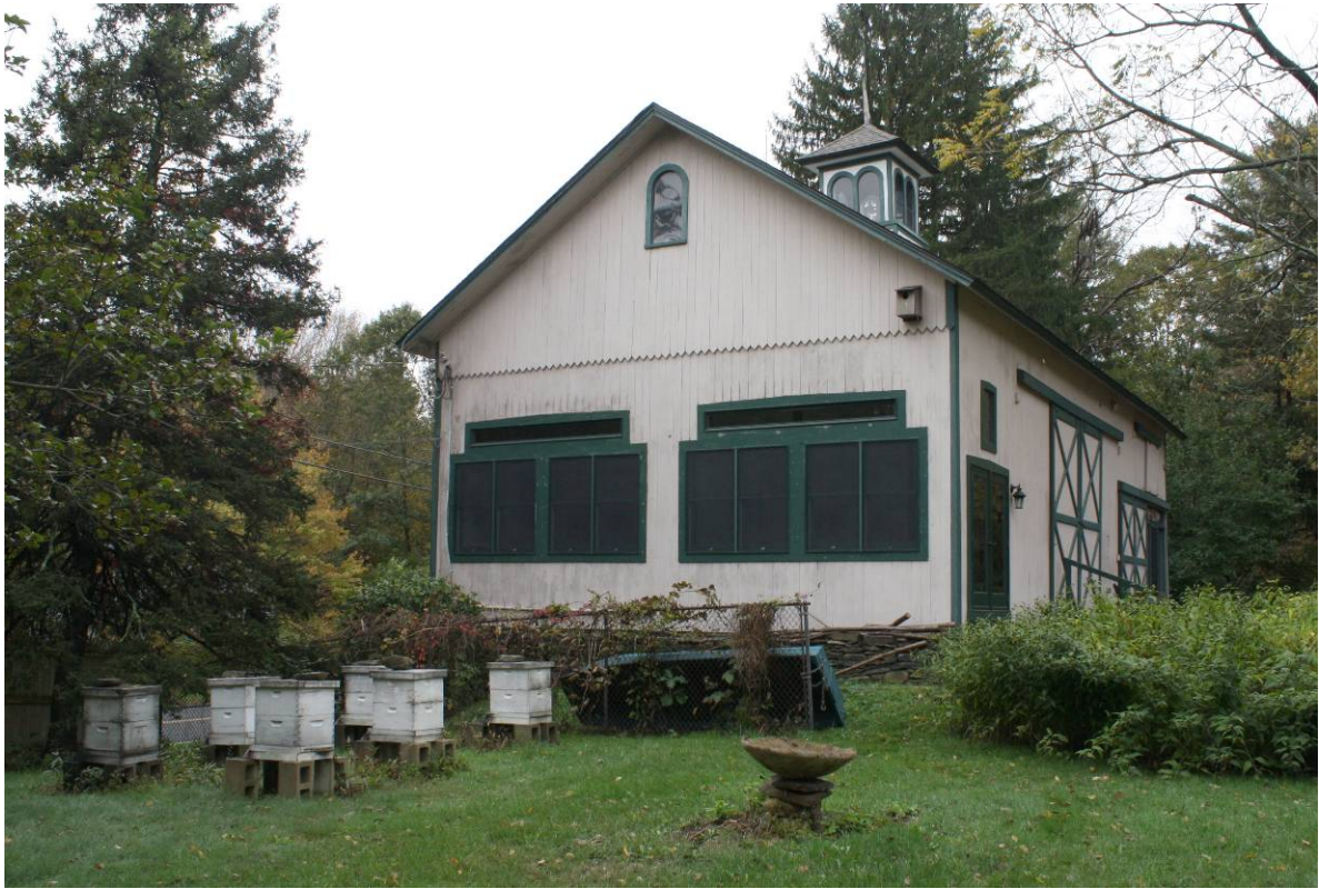
8. Northeast view, camera facing southwest.
