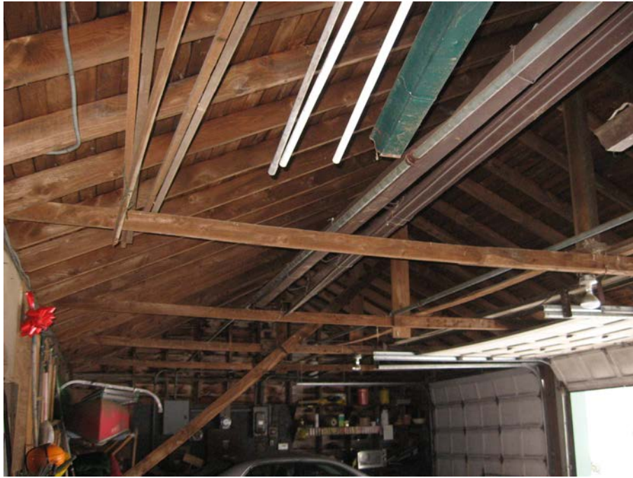
21. Interior view of Addition I, showing garage details, camera facing northeast.
