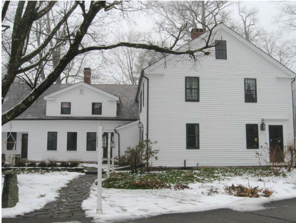
7. East gable-end of Farmhouse, camera facing west. Note rear ell details.
