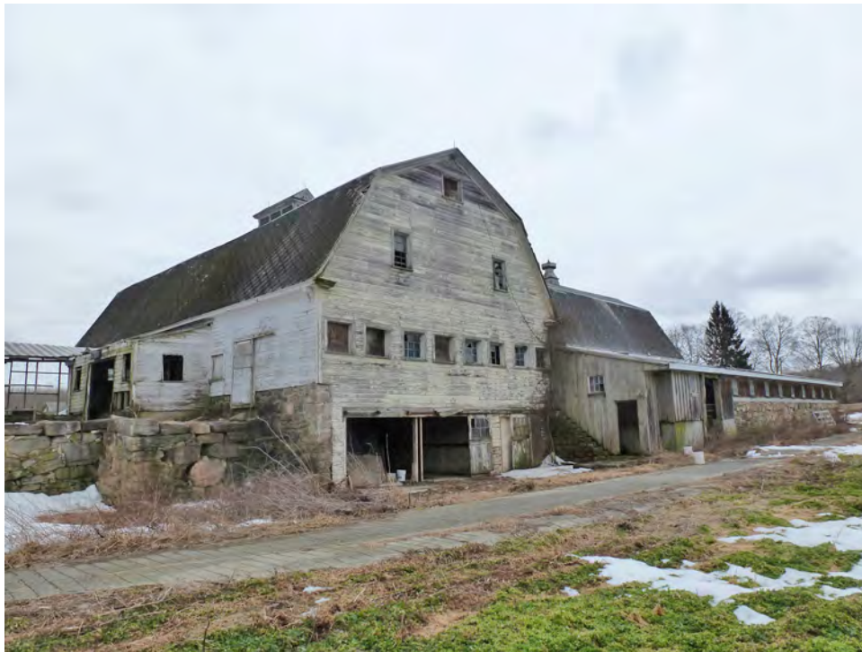
17. North eave-side and west gable-end of the north section of Barn I. Camera facing southeast. Note the partial banked basement.
