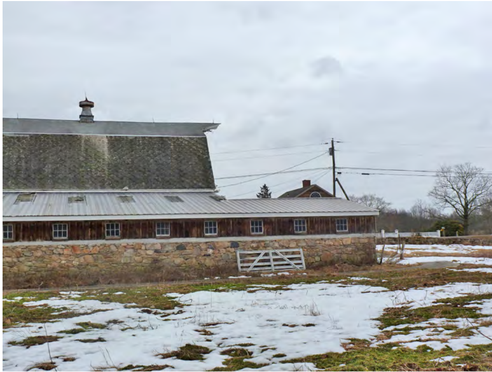
7. West view of Barn I (on the left) and the house (in the distance behind Barn I). Camera facing east.
