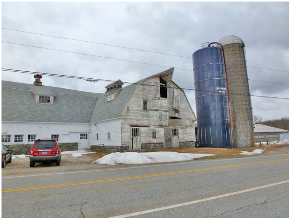
12. South eave-side and east gable-end of the north section of Barn I. Camera facing northwest.
