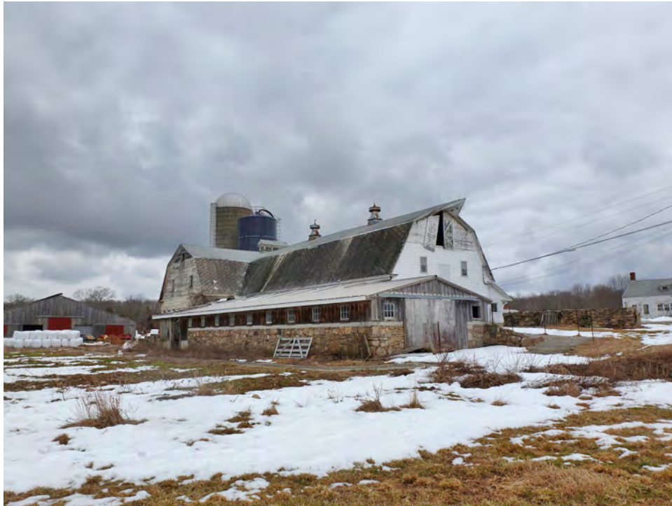
5. Southwest context view of Barn II (on the left), Barn I (in the middle) with its added west dairy stable wing, and a corner of Barn III (on the right). Camera facing northeast.
