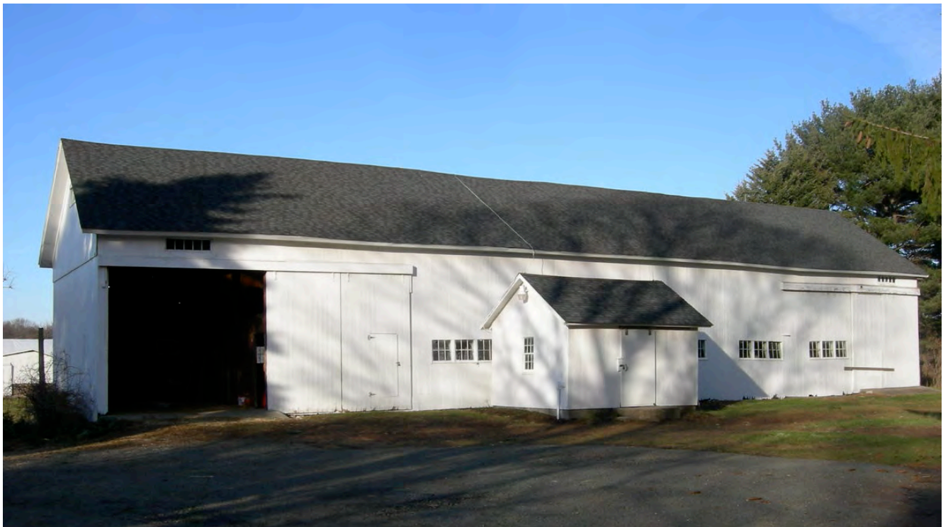
7. South view of Barn, camera facing north. Milk room is at center.
