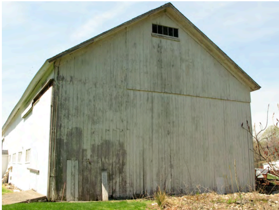
9. East view of Barn, camera facing west (Gould photo).
