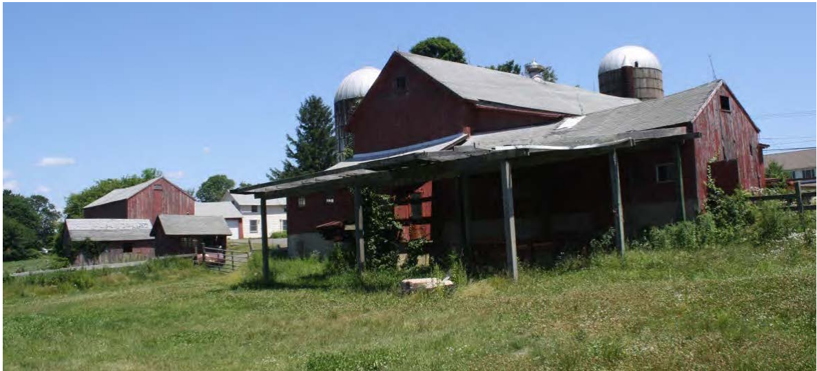
13. Southwest view of Barn I, Addition II, III and leanto, with corn crib, shed, Barn II and house in background.
