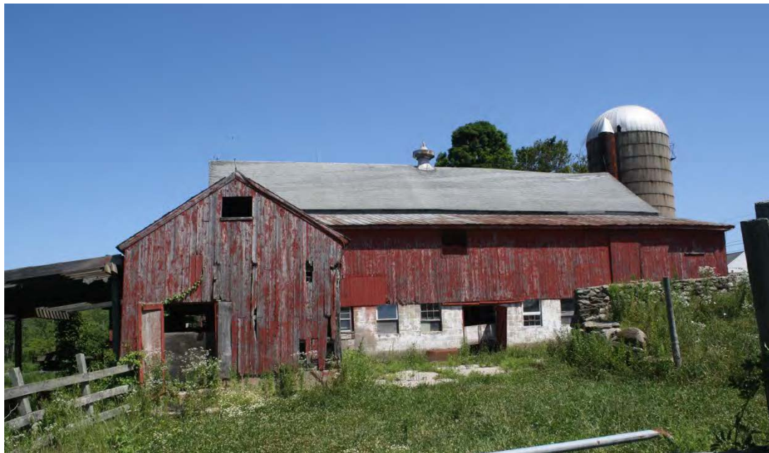
12. South view of Addition II and I, camera facing north.
