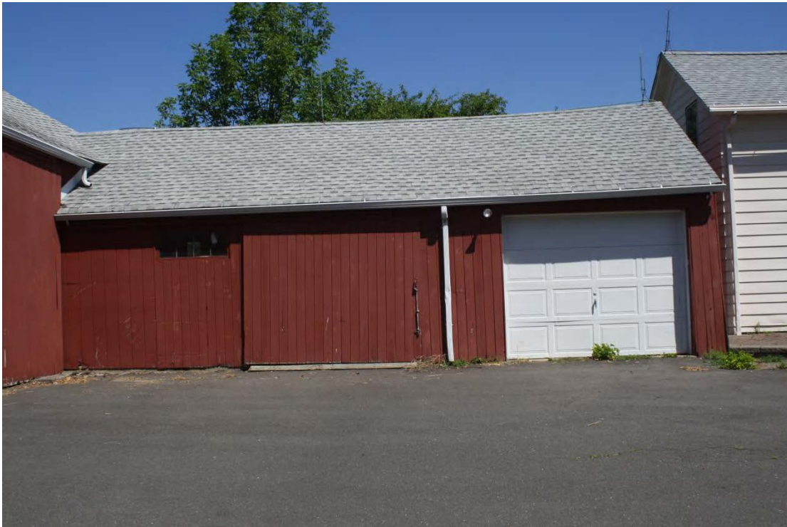
26. South view of Carriage barn addition, camera facing north.
