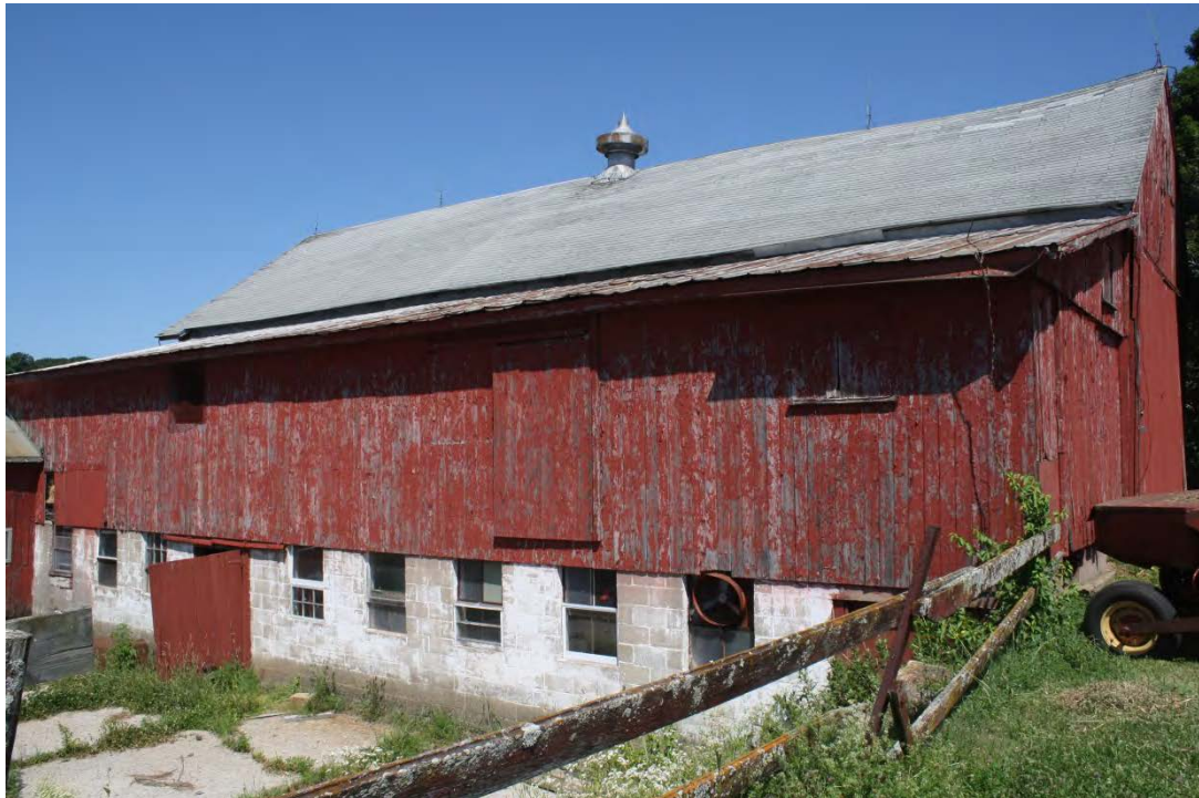
10. South side view of Addition I, camera facing northwest.
