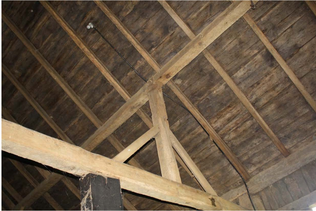
19. Detail of interior, queen trusses and purlin plates in Barn I, camera facing southeast.
