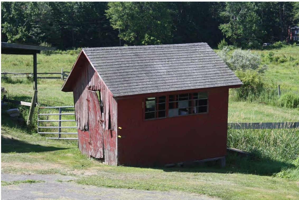
6. Northeast view of Corn crib, camera facing southwest.
