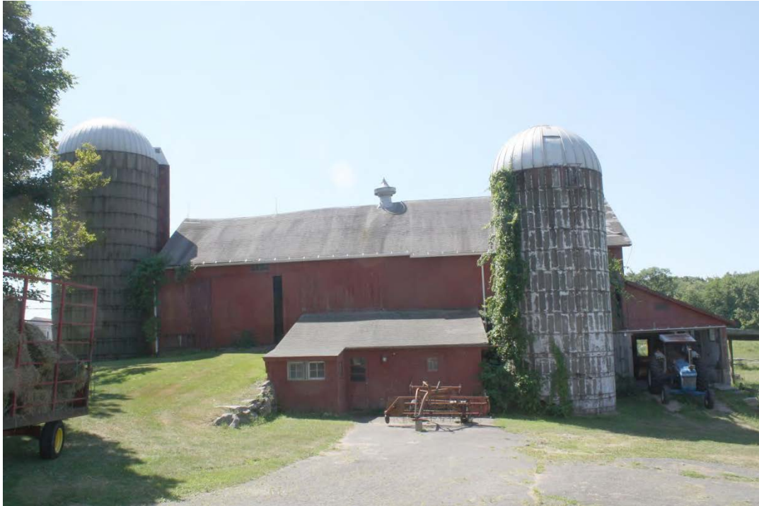
17. North view of Barn I, Addition III and IV, with silos, camera facing south.
