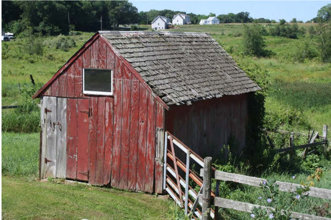
7. Northeast view of Shed, camera facing southwest.
