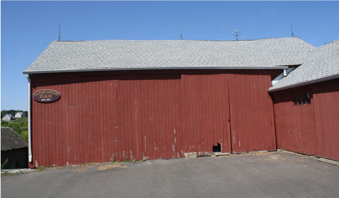
25. East view of east-eave side of Barn II, camera facing west.
