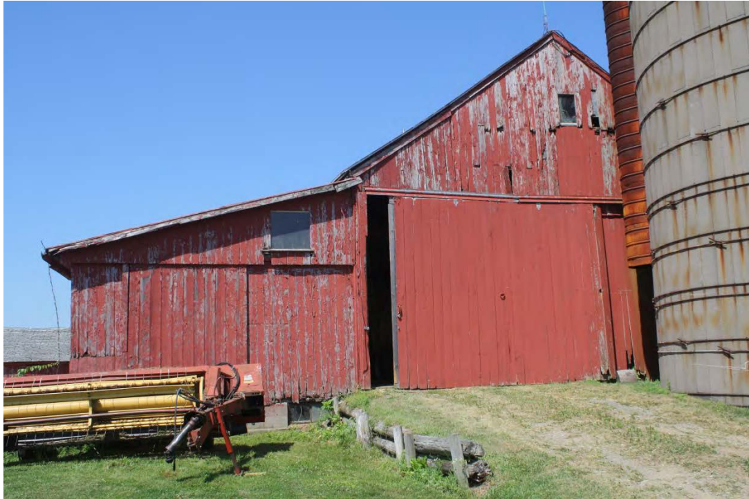
9. East gable-end view of Barn I, Addition I and Silo, camera facing west.
