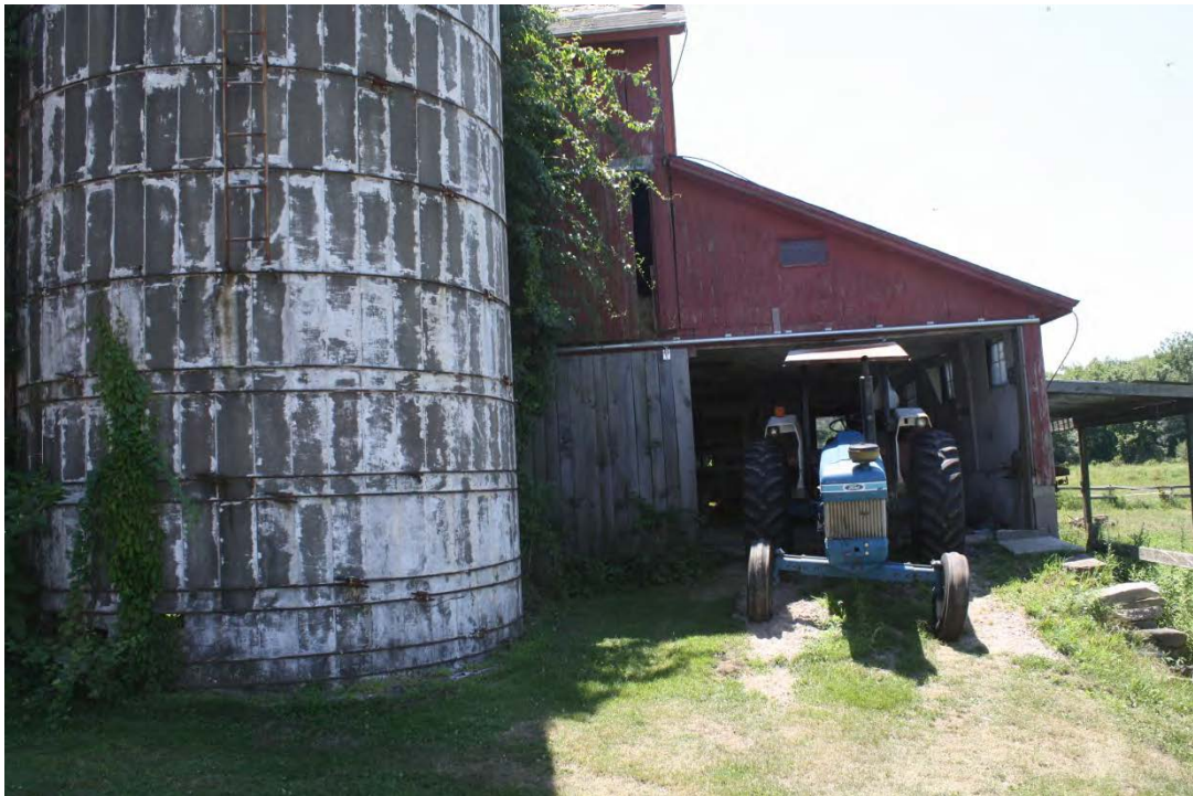
16. North view of Addition III and concrete tile stave Silo, camera facing south.
