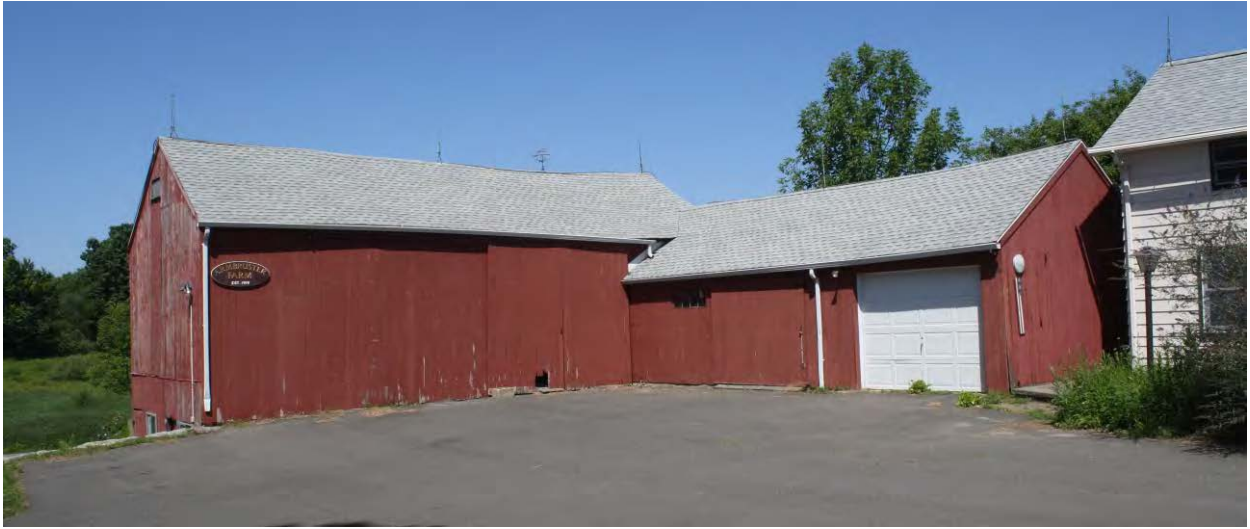
5. Southeast view of Barn II and Carriage barn addition, camera facing northwest.
