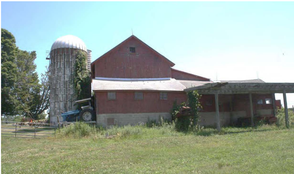
14. West view of Barn I, Silo, Addition II, III and lean-to, camera facing east.
