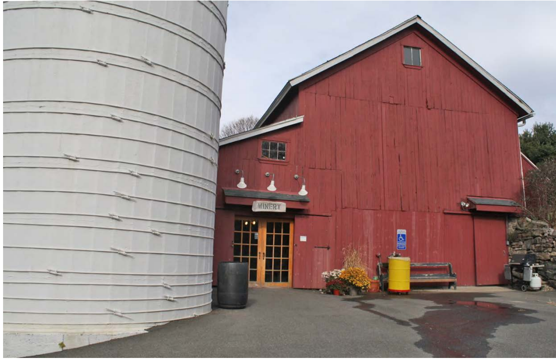
9. South view of the Main barn and Silo, camera facing north.
