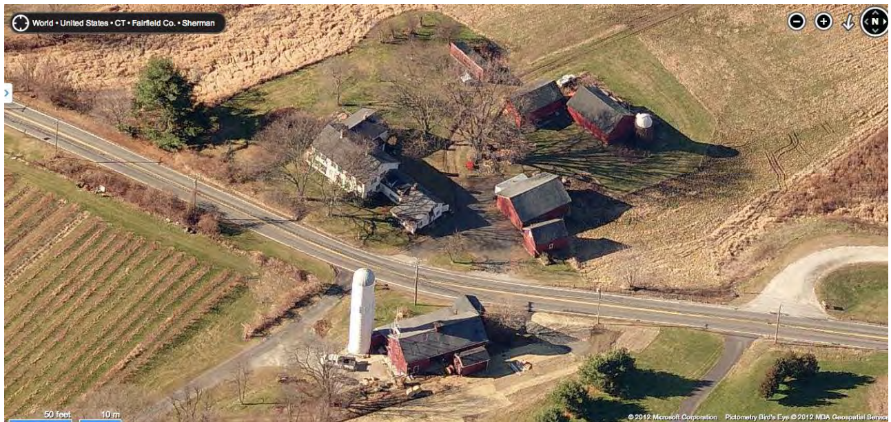
2. East view – aerial “bird’s-eye” map of 32 Route 37 East, Sherman CT – http://www.bing.com/maps accessed 11/13/2012. South of (below) the road is the White Silo Farm barn and silo. North of (above) the road is the Albert Barnes house and the other barns of the Osborns’ Upland Pastures Farm.
