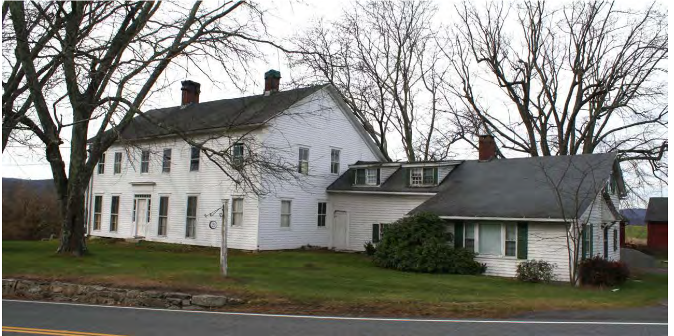
5. Southeast view of 29 Route 37 East, the Albert Barnes House, camera facing northwest.
