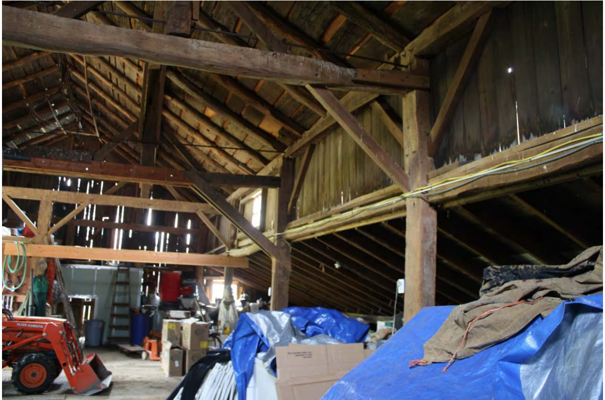
15. Interior view, camera facing south. Note the shed roof framing of the western addition at right.
