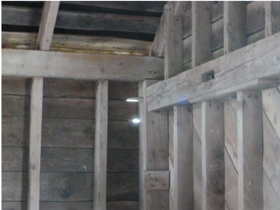
16. Interior view of the northwest corner of the barn. Note the mortise and tenon joint with tree nails typically found in post-and-beam frames. Camera facing northwest.
