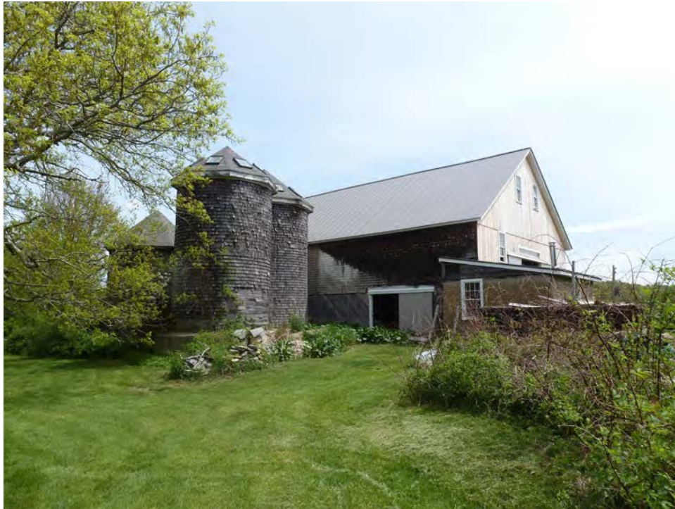
5. Southwest context view of the Silos and the Barn. Camera facing northeast.
