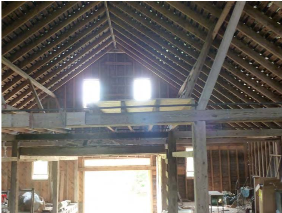
14. Interior view of the Barn, camera facing south.
