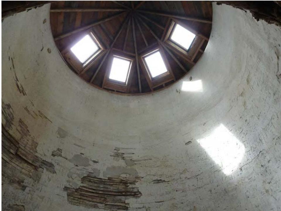
19. Interior view of one of the wood shingled silos. Note the bent wood lathe and plaster finish.
