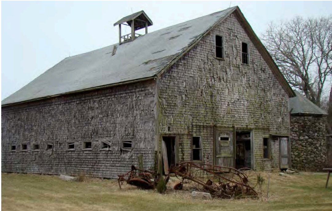
21. Northeast view of the Barn in 2007, prior to restoration work.
