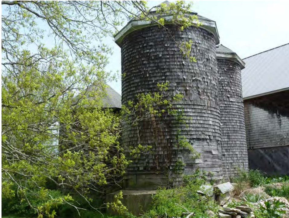
7. Southwest view of the three silos. Note the two wood shingled Silos II and I in the foreground and the stone Silo II in the background behind the trees. Camera facing northeast.
