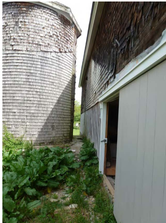
10. West eave-side of the Barn and Silo I. Camera facing north.
