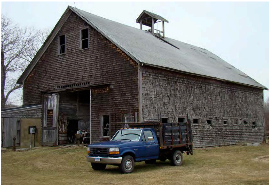
20. Southeast view of the Barn in 2007, prior to restoration work.
