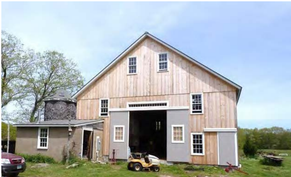
8. South gable-end of the barn, east and south sides of the addition. Camera facing north.
