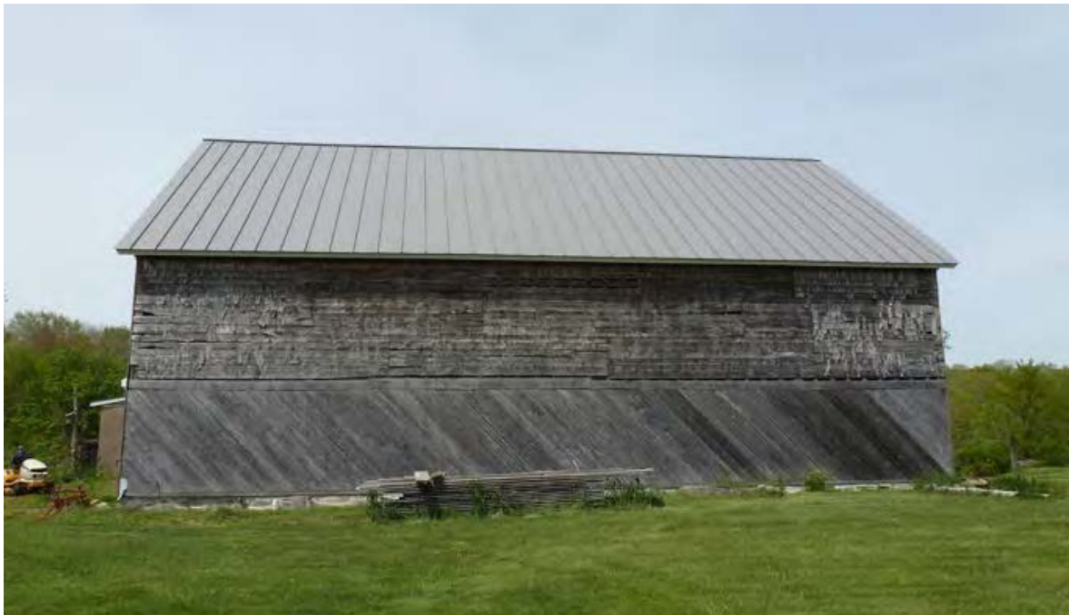
12. East eave-side of the barn. Camera facing west.
