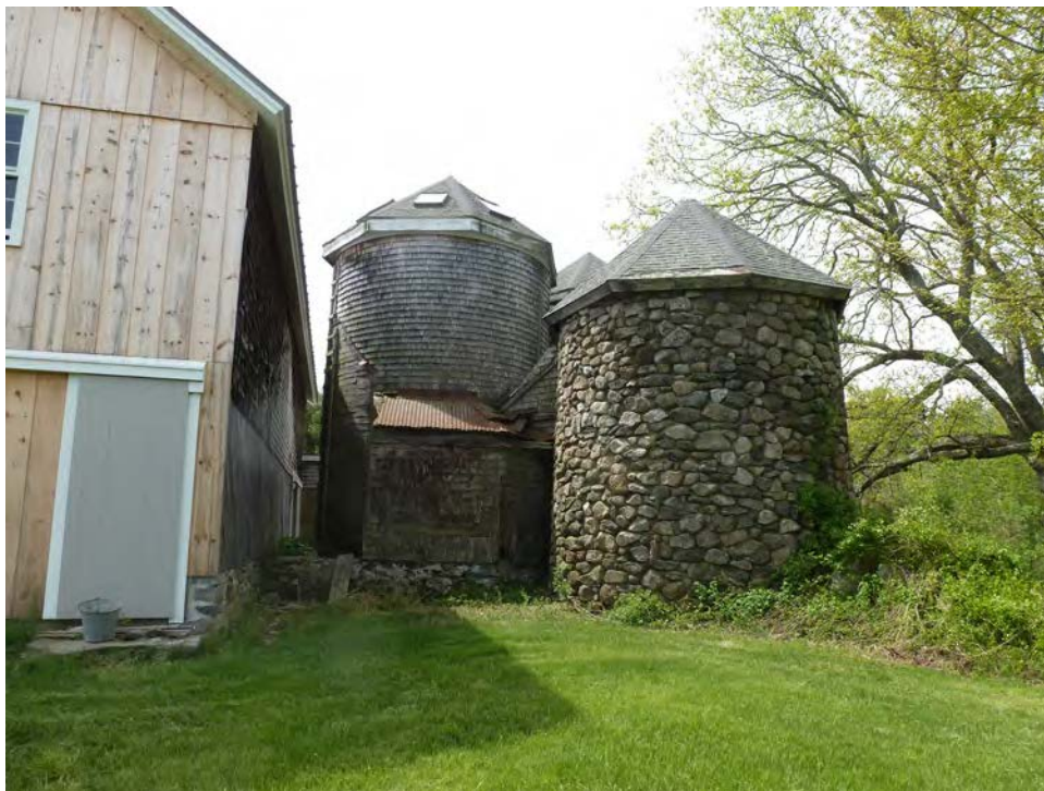
6. North view of the silos. Note the stone Silo III in the foreground and wood shingled Silo I in the background. Camera facing south.
