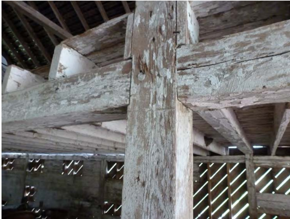
17. Detail of the post-and-beam frame with mortise and tenon joints. Note the whitewash indicating former dairy use. Camera facing east.
