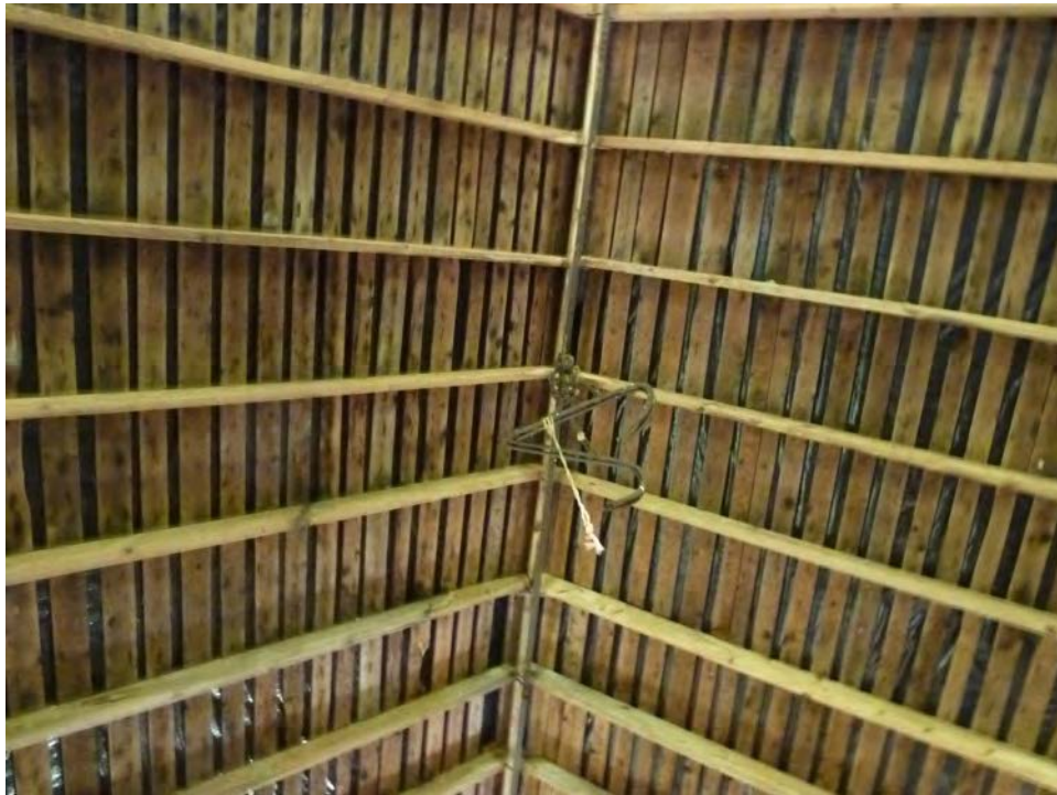
18. Interior view of the roof framing. Note the common rafters meeting at the peak with a ridge-board, narrow spaced deck boards, the hay fork, and the hay track.
