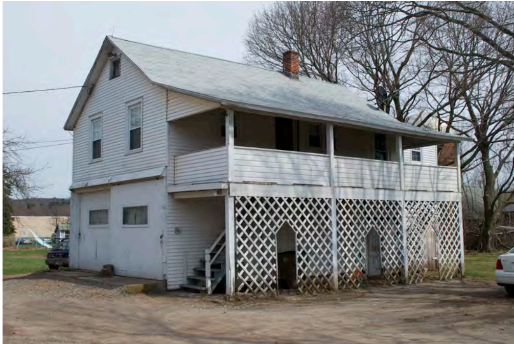
18. Northwest view of Farmhand housing, camera facing southeast. Note sliding doors on north gable-end lower level.
