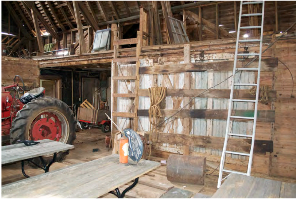
28. Interior of Barn main block, showing sliding door between main block and rear ell, camera facing southeast. Storage area behind wall at right, workshop at far left.
