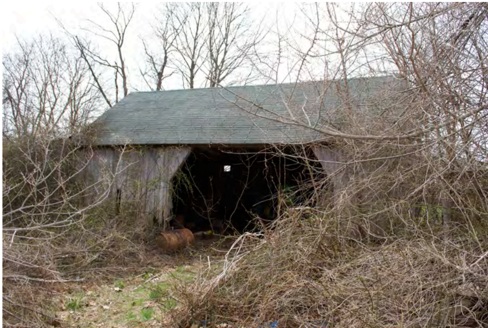
19. East eave-side of Wagon shed, camera facing southwest.
