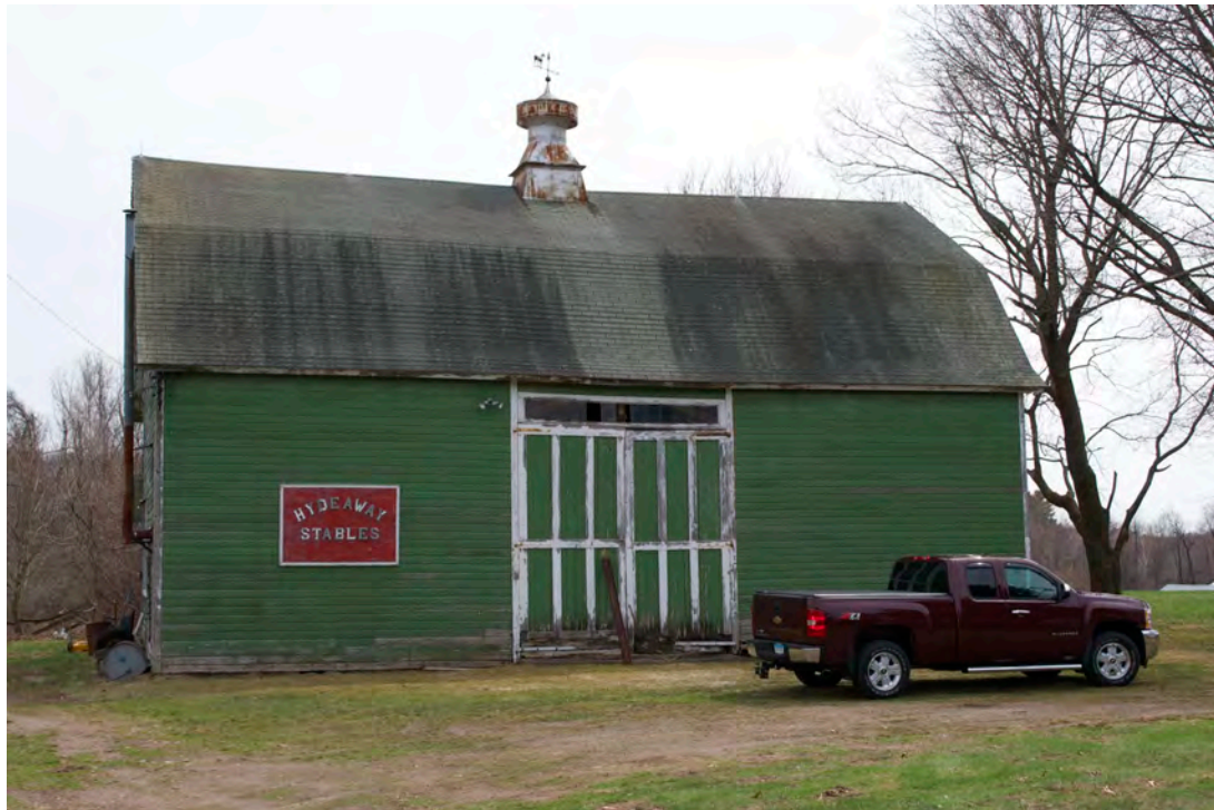
21. North view of Barn, camera facing southwest.
