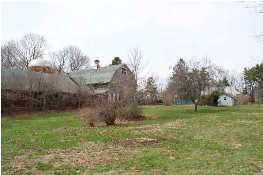
11. Southeast context view of Gunther Farm, camera facing northwest. From left to right, Barn, Pool and Pump House, Farmhouse I at rear right, Silo at rear left.
