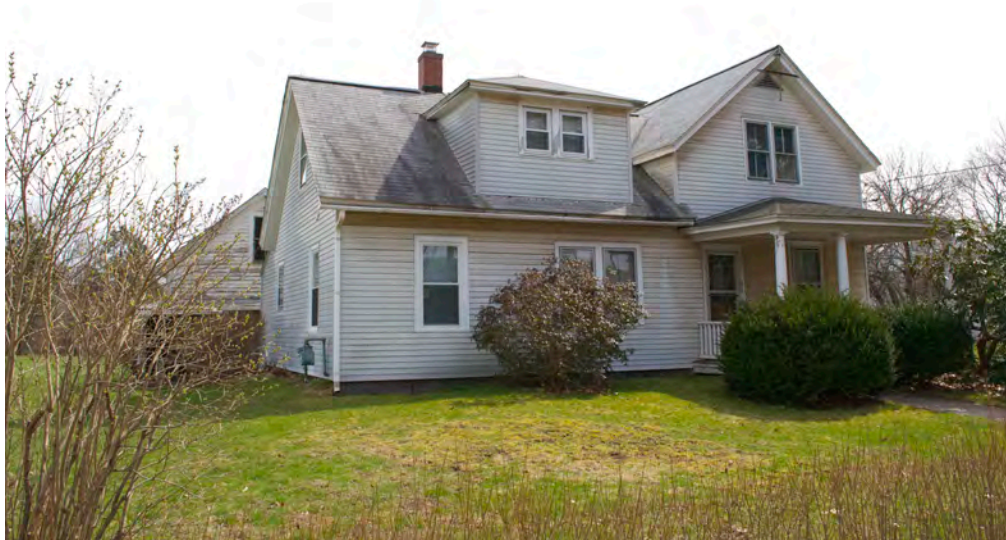
12. North and east view of Farmhouse I, camera facing southwest. Note Garage at left rear.
