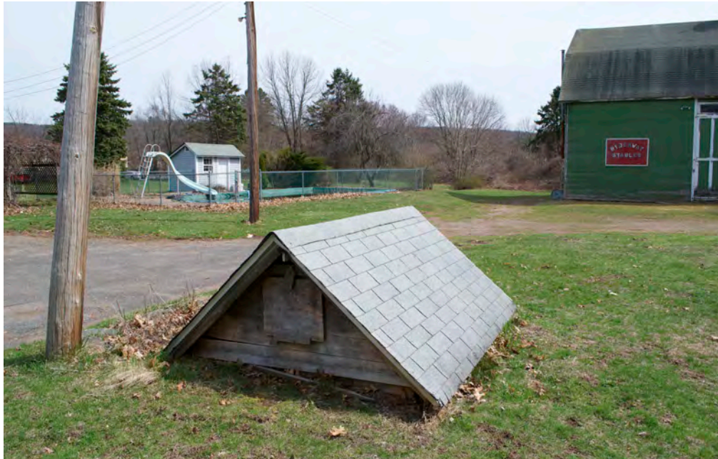
16. North gable-end and west eave-side of Wellhouse, camera facing southeast. Note Pool at left, Barn at right.
