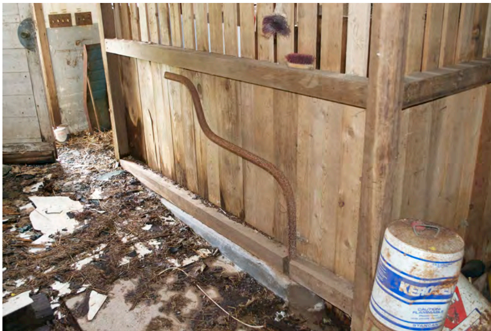
31. Interior of Barn rear ell, showing surviving stanchion detail, camera facing southeast. Note east eave-side entry at left.
