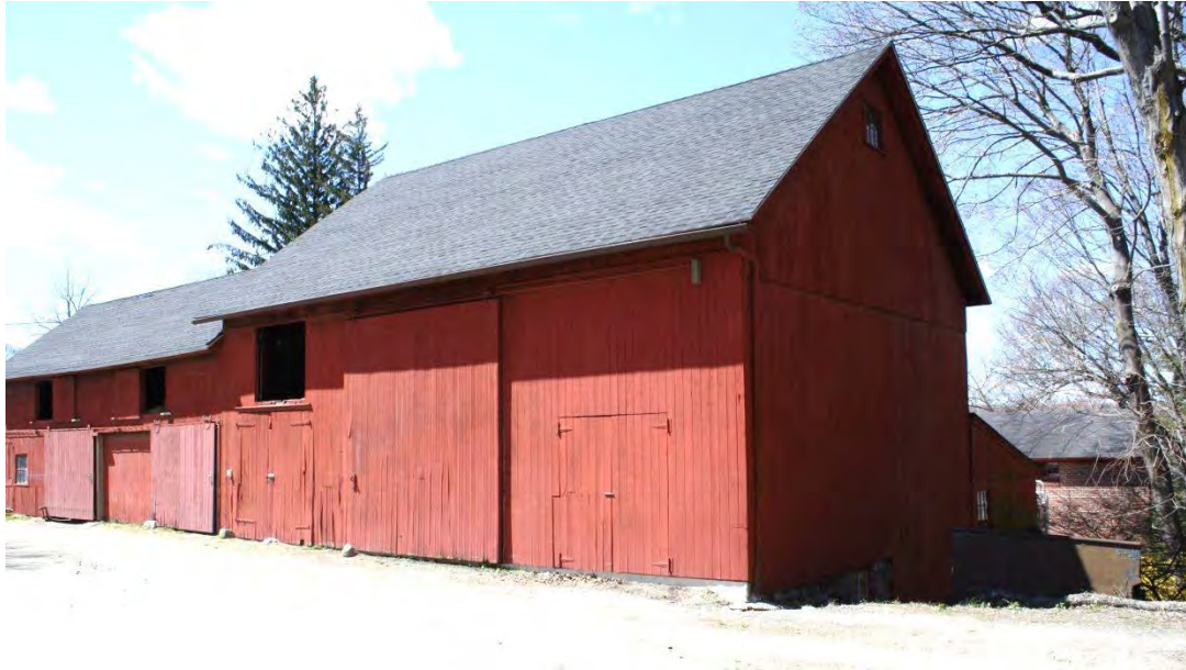
7. Northeast view of Barn I, camera facing southwest. Barn II is at left.
