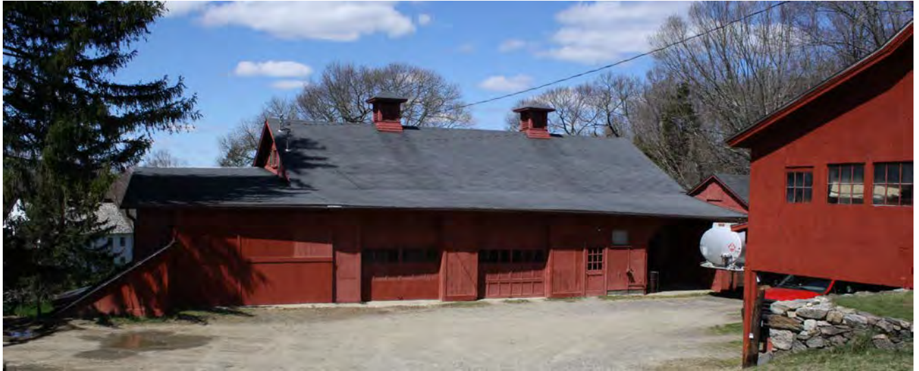
17. East view of Barn III showing Addition II, across the east façade, Addition III at left, and Addition I at right behind the fuel truck. Note cupolas on the ridge.
