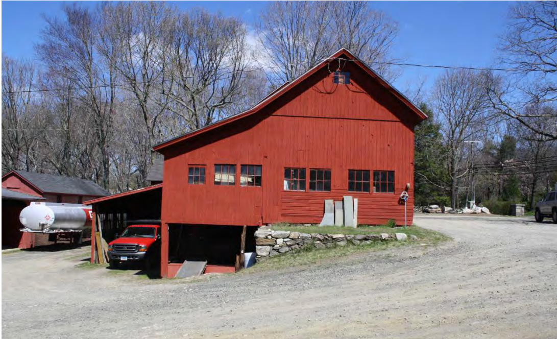
11. View of south gable-end of Barn II, camera facing north.
