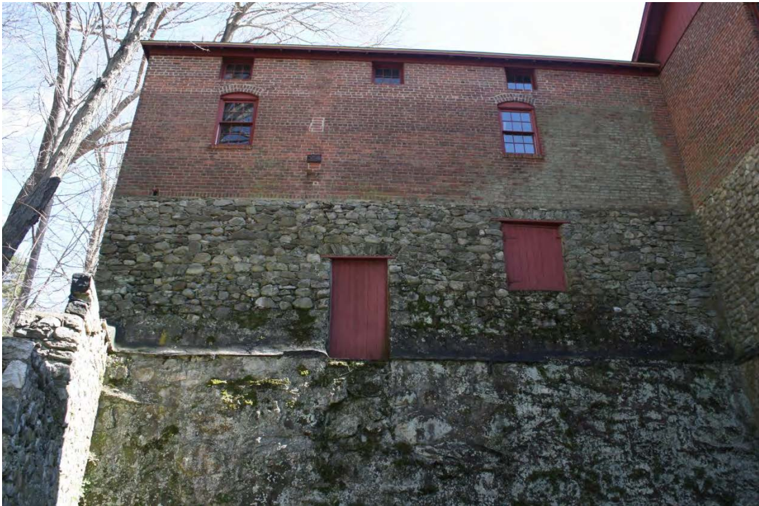
26. West view of Addition I, camera facing east.
