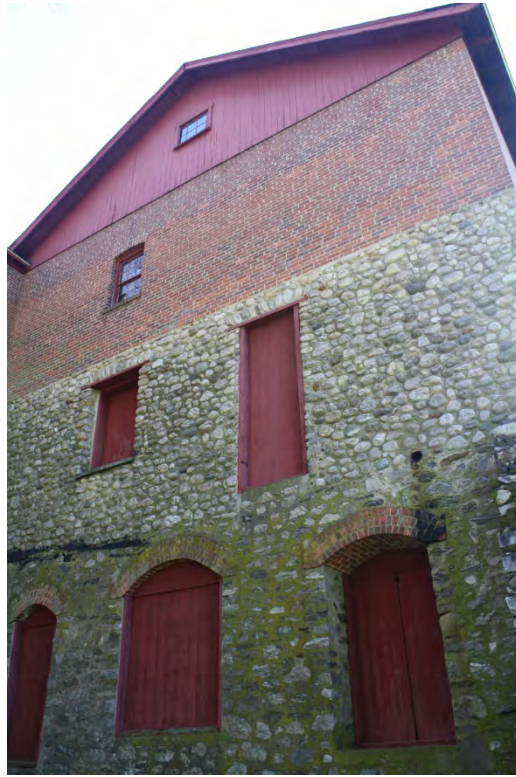
25. North view of Barn III, camera facing south.
