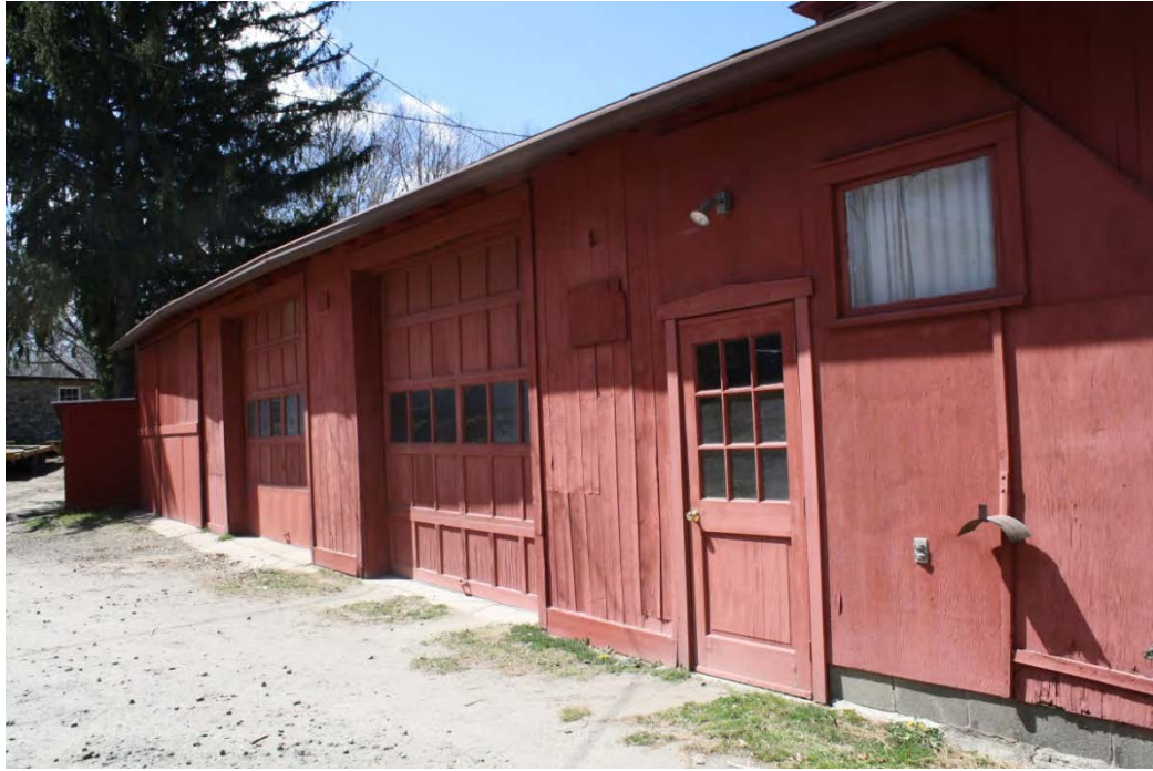
19. East view of Addition II of Barn III, camera facing southwest.
