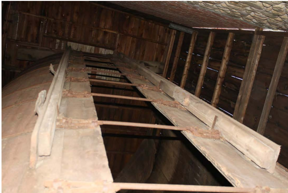
33. Detail of wood stave silo inside Addition III, camera facing up.
