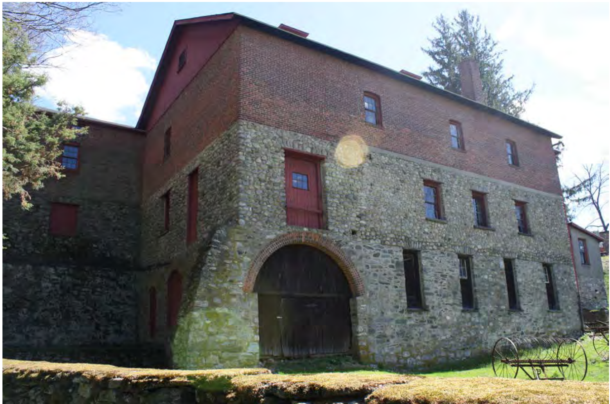
24. Northwest view of Barn III, camera facing southeast.
