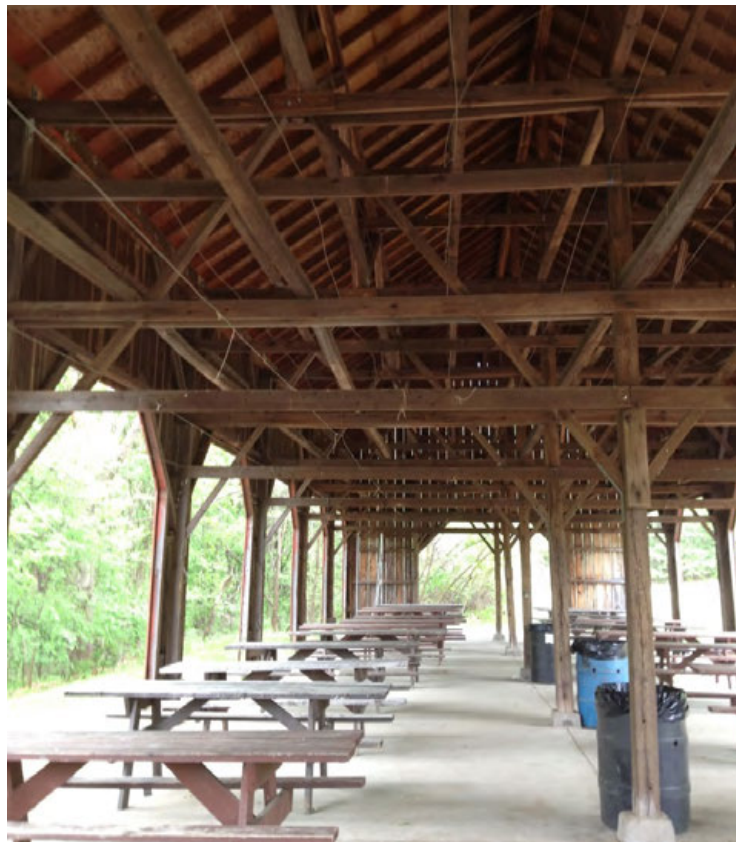
17. Interior view of Picnic pavilion, camera facing south.
