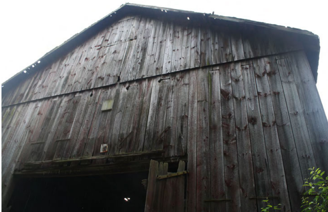
32. North view of Field barn IV, camera facing south.
