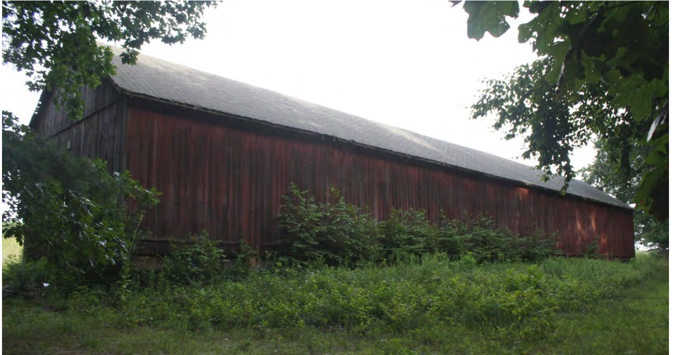
33. Northwest view of Field barn IV, camera facing southeast.
