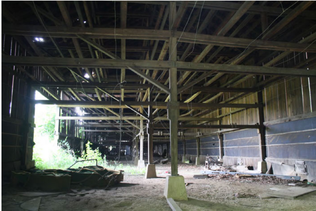
31. Interior view of Field barn IV, camera facing south.
