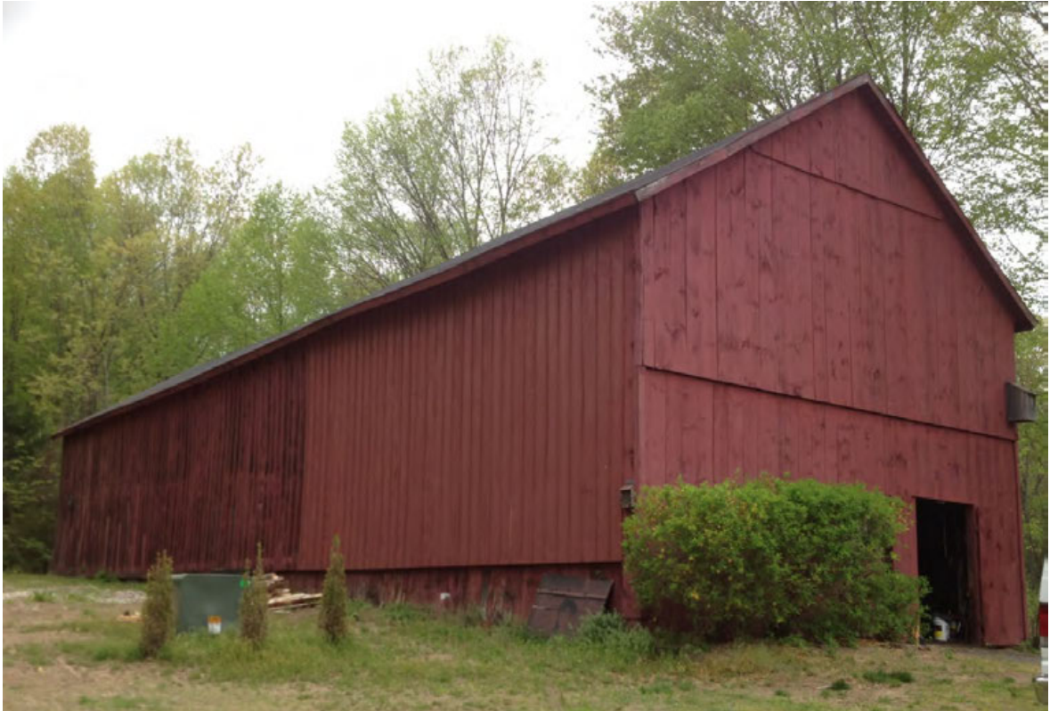
19. Southeast view of Maintenance shed, camera facing northwest.
