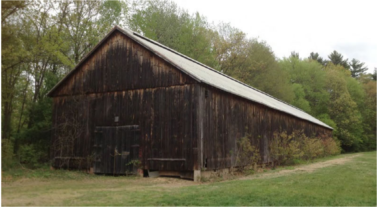
23. Southwest view of Field barn I (Tobacco shed), camera facing northeast. Note the metal roof with continuous ridge ventilator.
