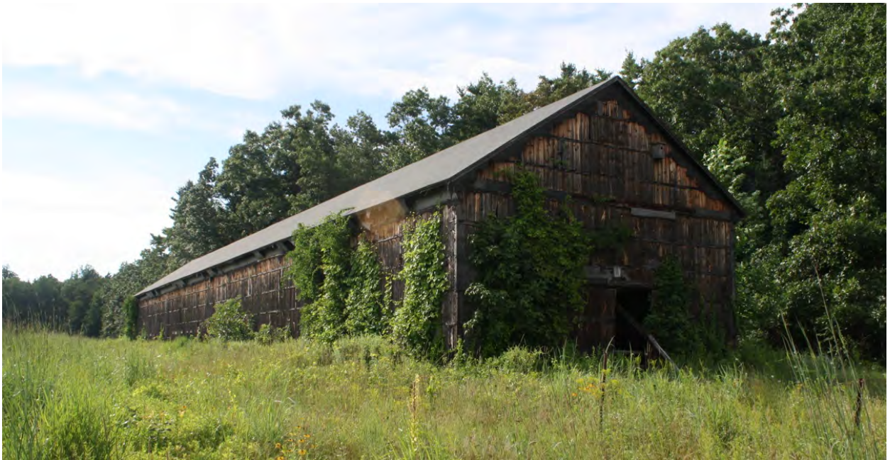
28. Southeast view of Field barn III, camera facing northwest.
