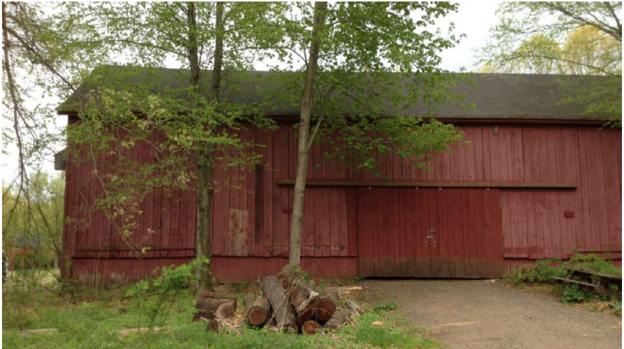
19. North view of Maintenance shed, camera facing south.
