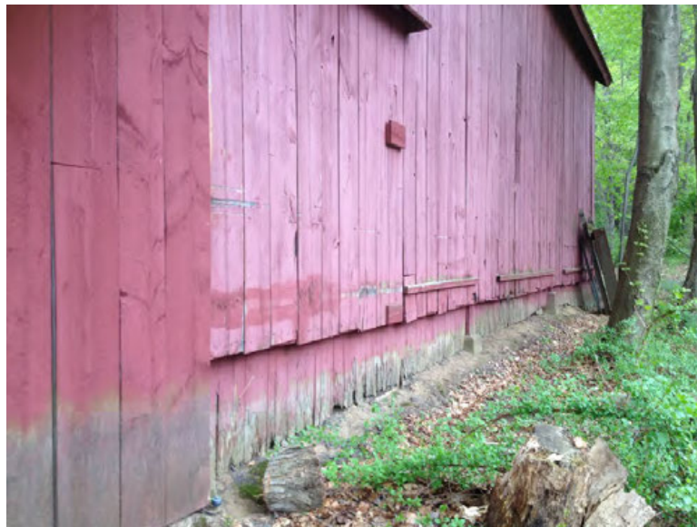
20. North detail view of Maintenance shed, camera facing southwest.
