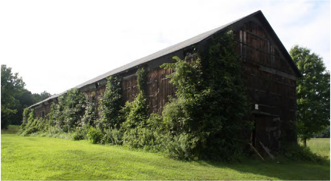
25. Southeast view of Field barn II, camera facing northwest.
