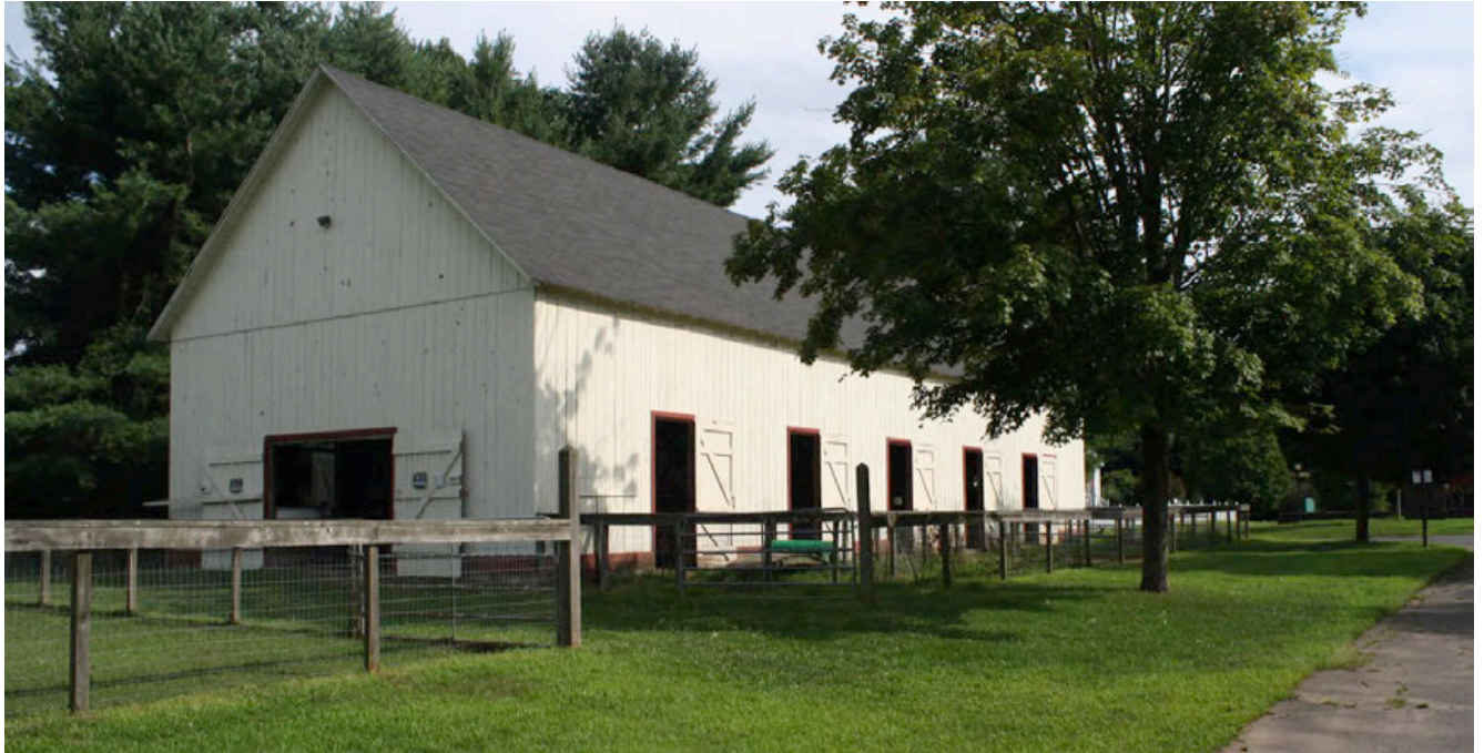
21. Northwest view of Animal barn, camera facing southeast.
