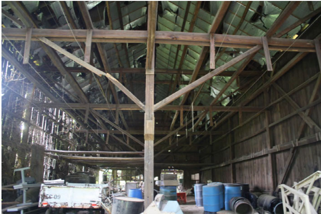
27. Interior view of Field barn II, camera facing west.
