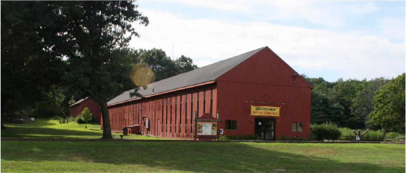
18. Southeast view of Nature center, camera facing northwest.
