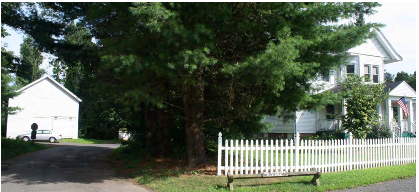
7. West view of Farmhouse with Horse barn at left rear, camera facing east.
