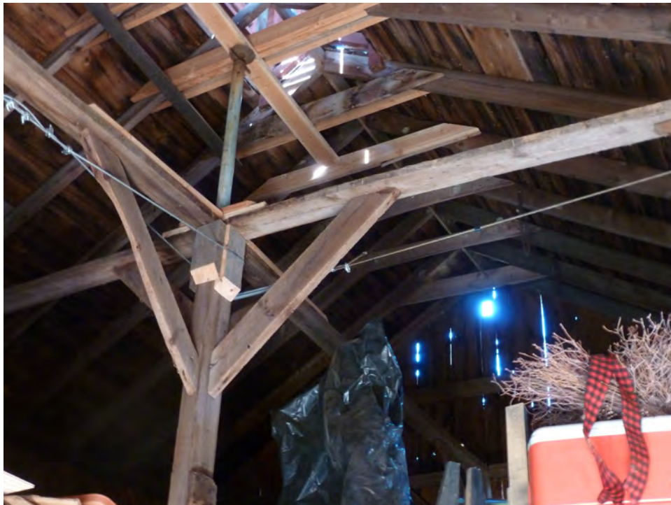
18. Interior view of the north gable-end of the Barn. Note the nailed timber framing. Camera facing north.
