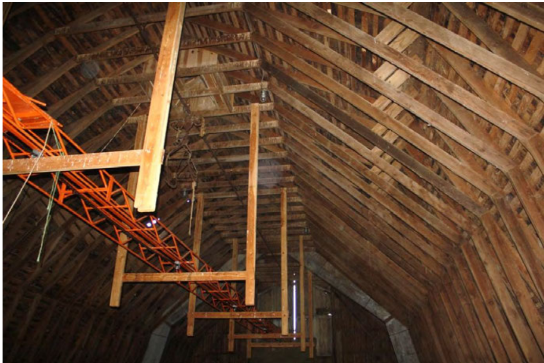
31. Interior detail view of attic loft, camera facing south.
