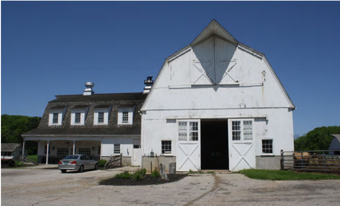
15. South gable-end of barn and addition, camera facing north. Note original diagonal sliding hay doors.
