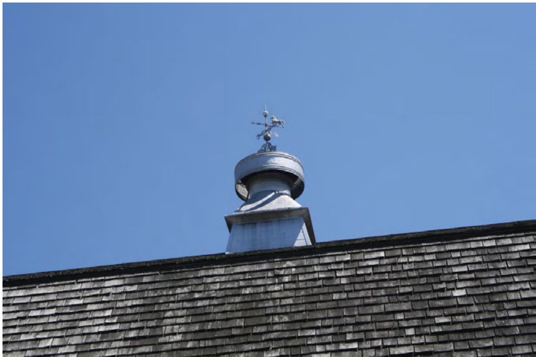
24. Detail of barn metal ventilator, camera facing east.
