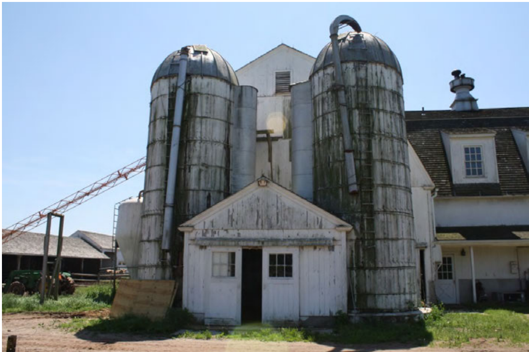
18. North gable-end of barn and silos, camera facing south.
