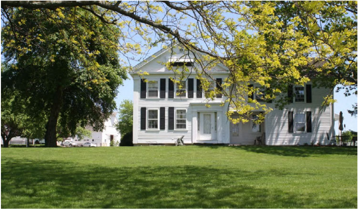
5. West view of Jabez Loomis White house, camera facing east. Note barn on left behind house.
