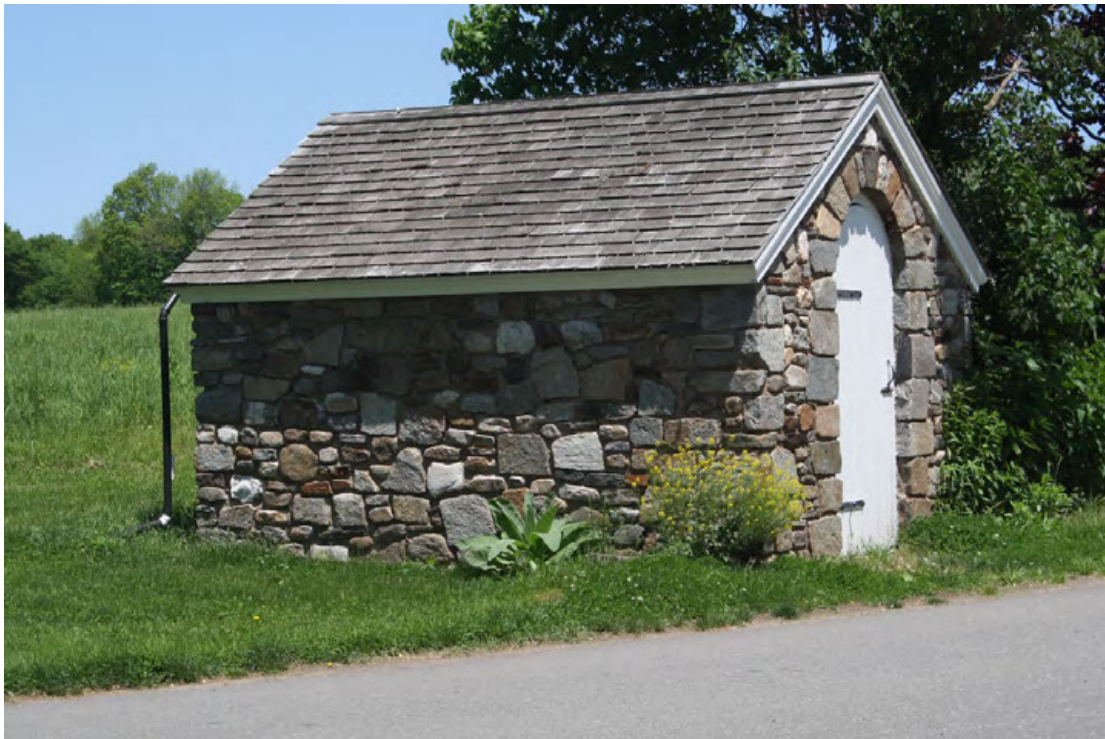
12. Stone shed, camera facing north.
