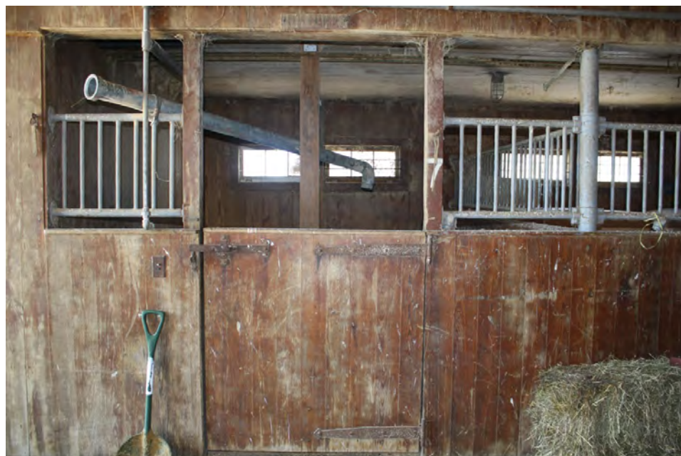
26. Detail of interior box stall, camera facing west.
