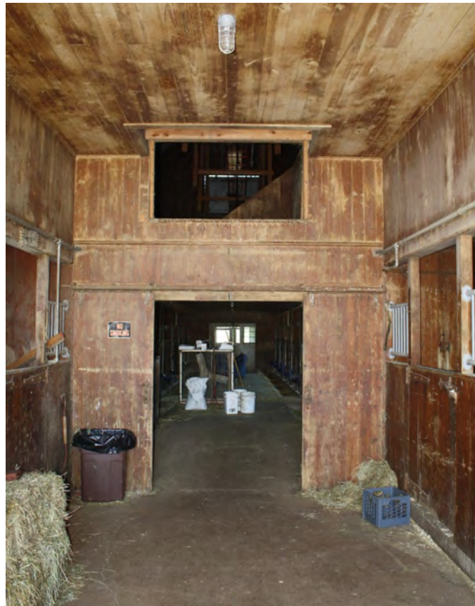
25. Interior of barn entry, camera facing north.
