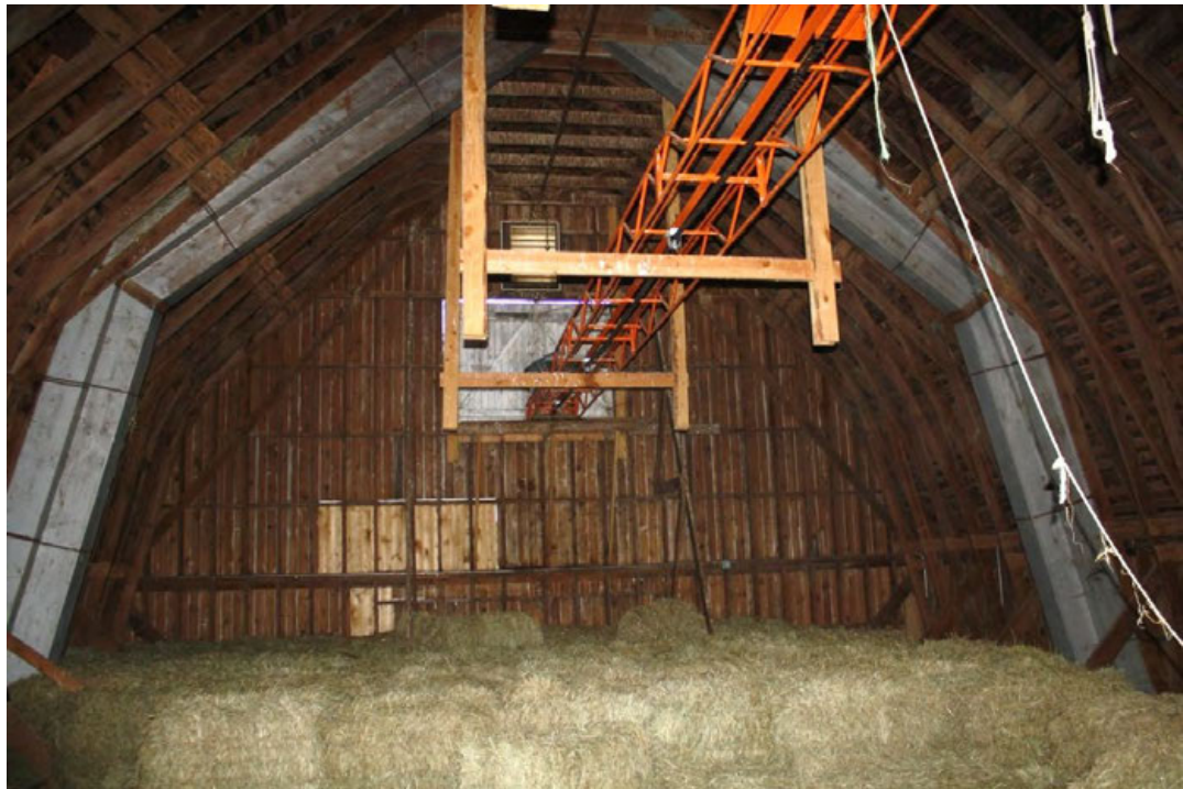
30. Interior detail view of attic loft, camera facing north.
