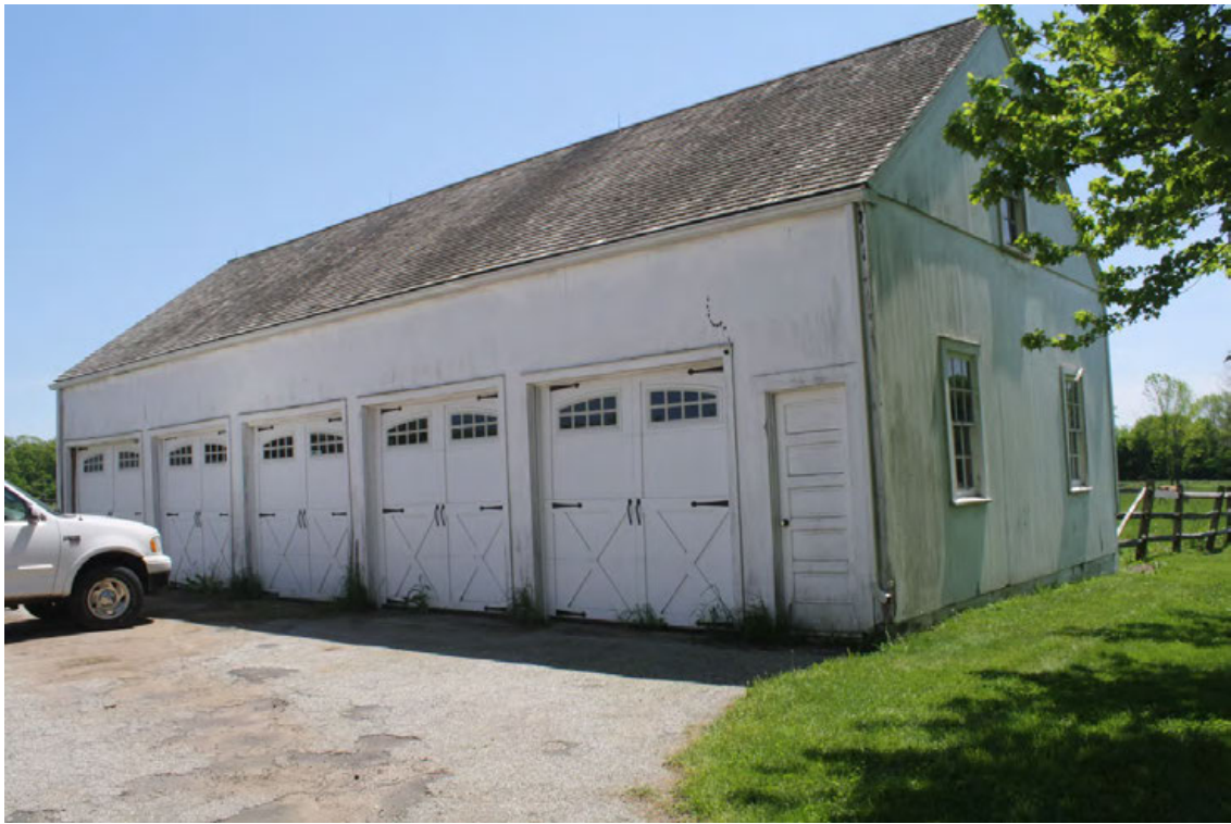
13. North eave-side of the five-bay garage, camera facing south.
