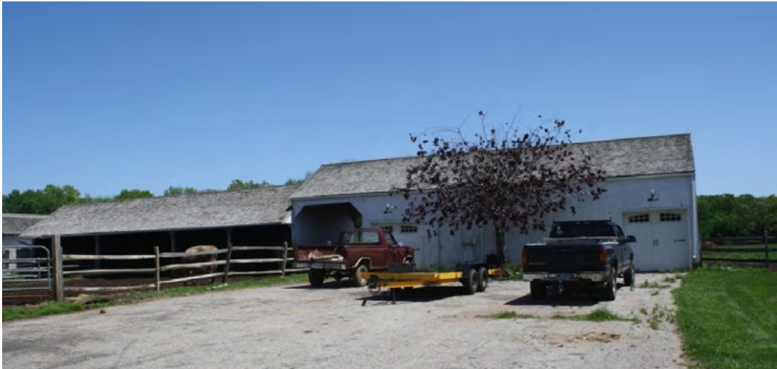
9. East side of sheds to the east of the barn. The south shed is for apple storage and the north section has a four bay for wagons, now used for storage and farming equipment.
