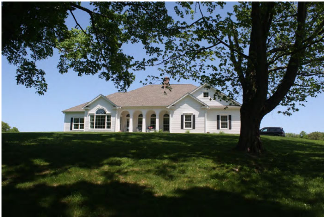
32. West view of modern house built in 2011, camera facing east.
