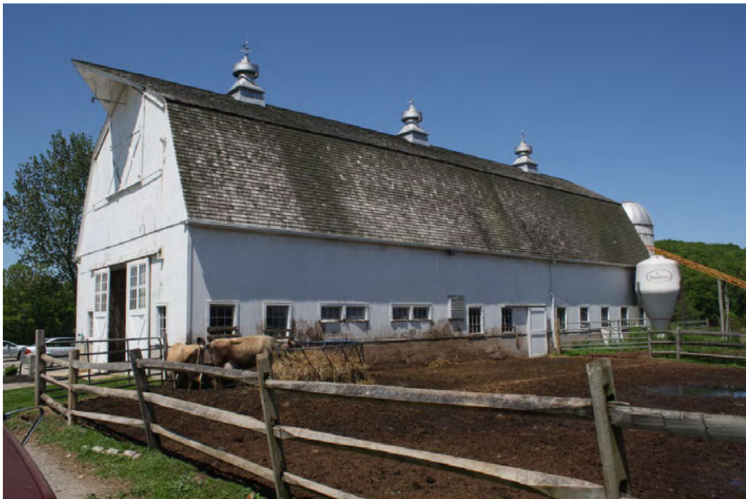
16. Southeast corner of barn, camera facing northwest.
