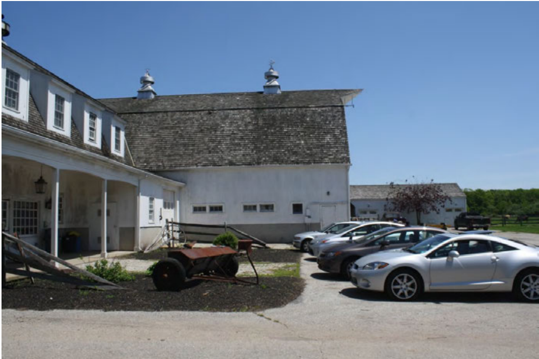
23. West eave-side of barn, camera facing east.
