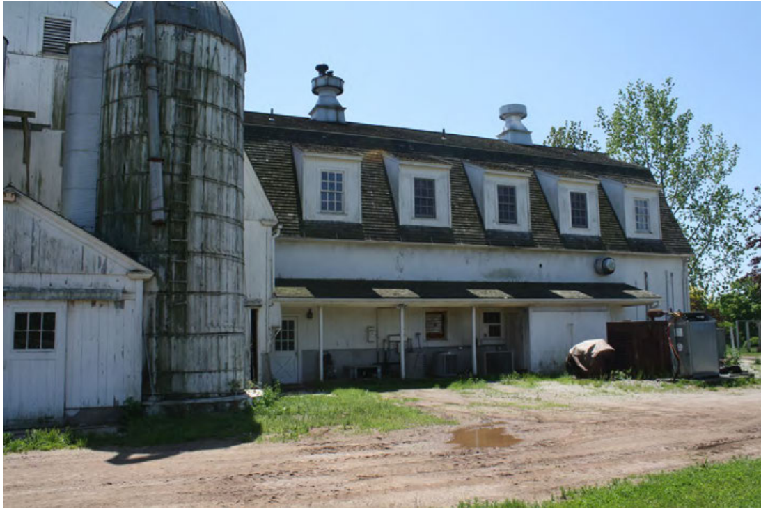
19. North eave-side of addition, camera facing south.
