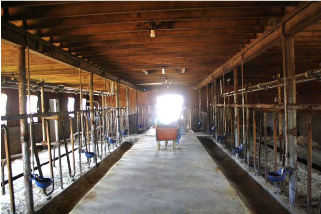
27. Interior of dairy stable with stanchions and center aisle, camera facing south.
