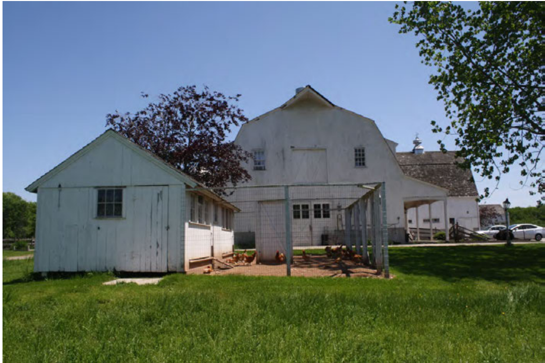
21. East gable-end of addition and Hen house, camera facing east.
