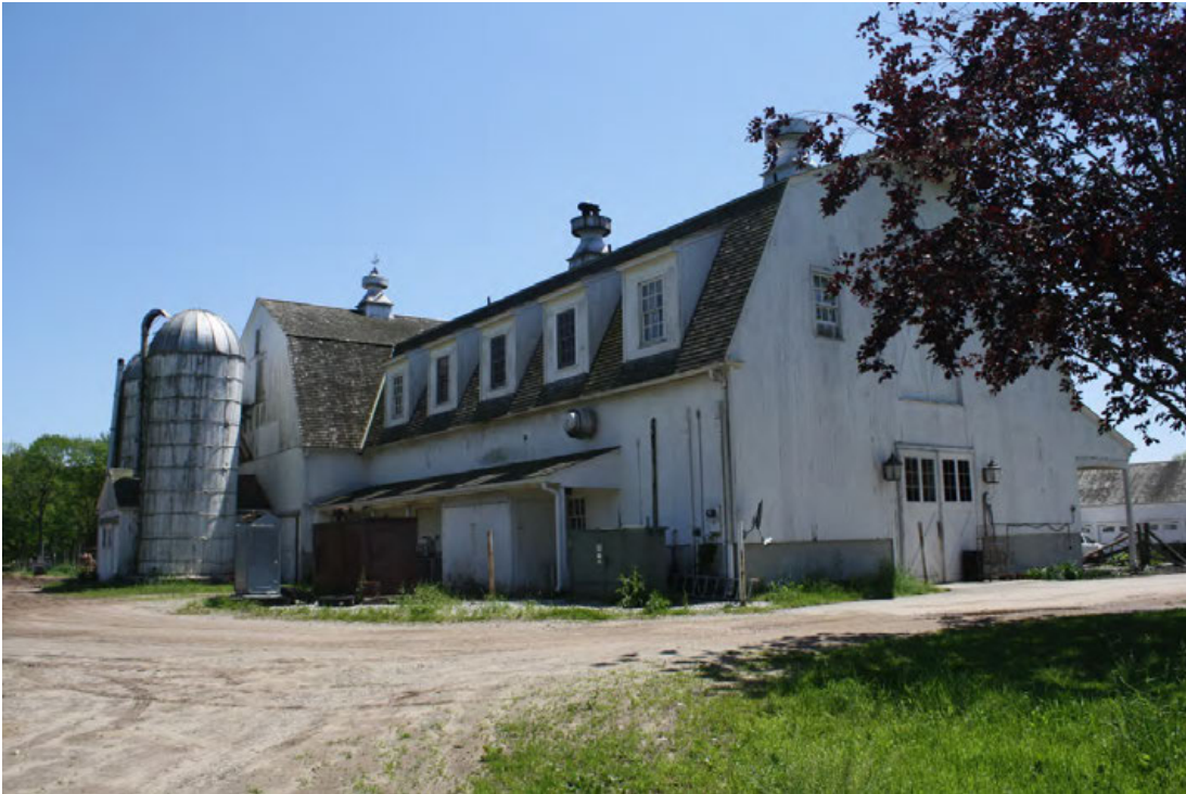
20. Northwest corner of addition, camera facing southeast.
