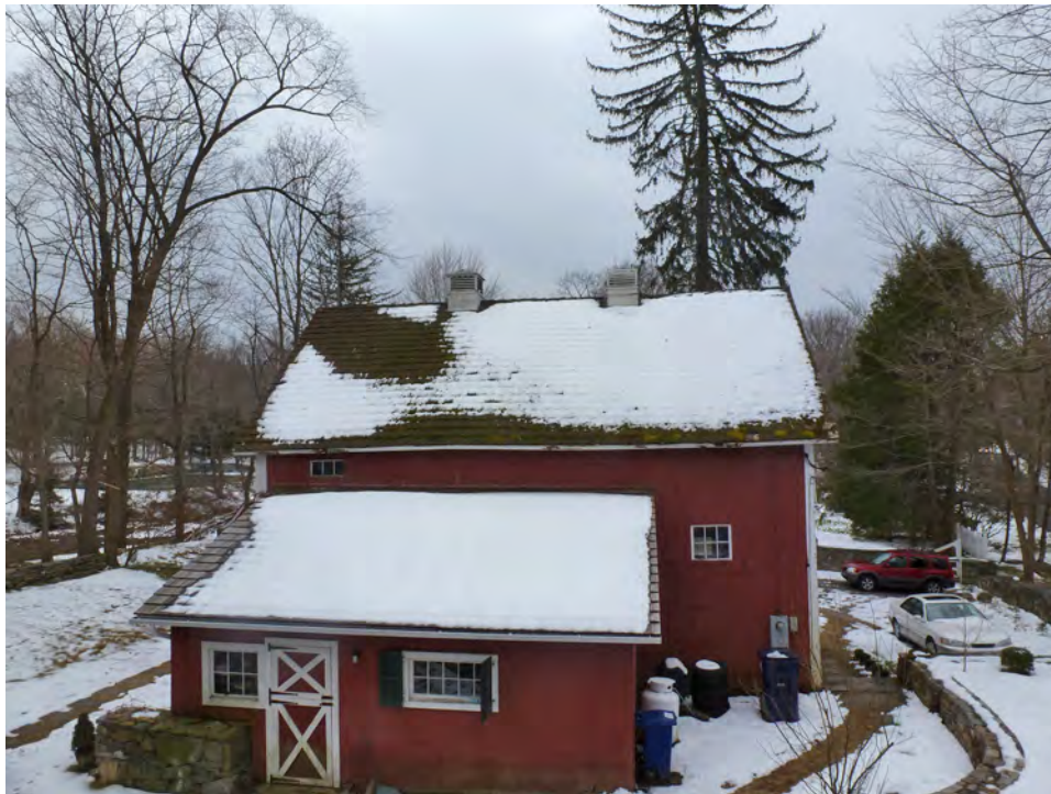
13. North eave-side of the Barn and shed-roof addition. Camera facing south.
