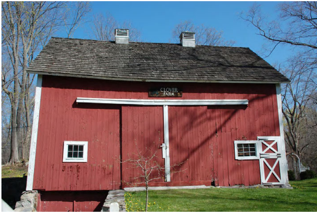
9. South eave-side of the Barn. Camera facing north.
