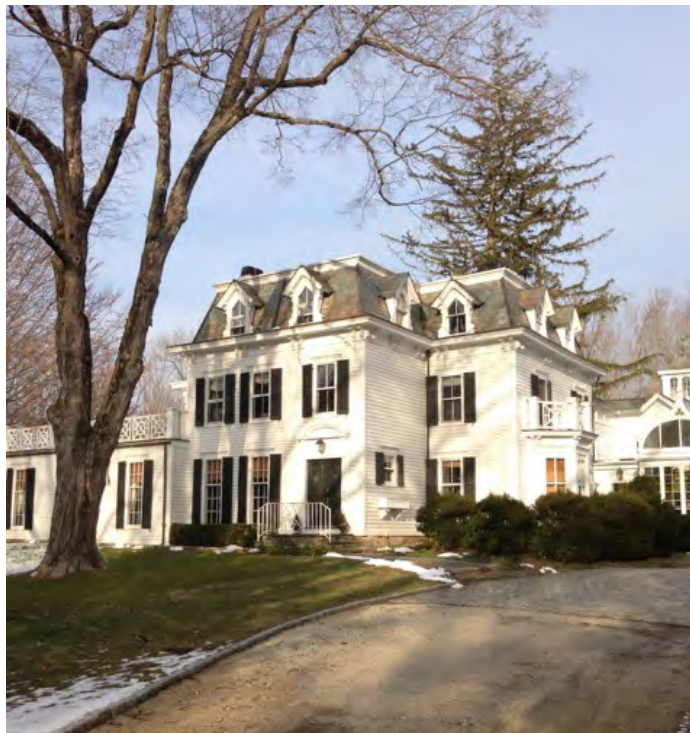
8. Southwest view of the house. Camera facing northeast.
