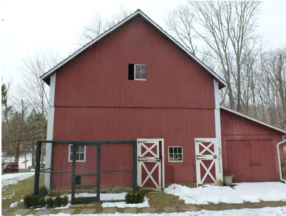
15. East gable-end of the Barn and shed-roof addition. Camera facing west.
