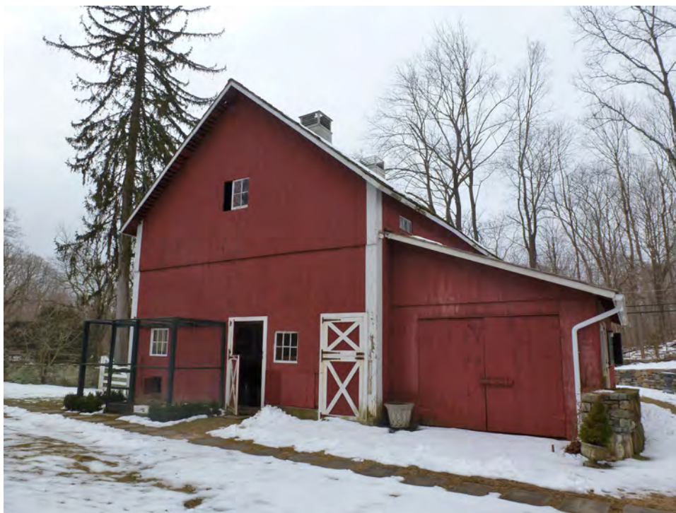
14. East gable-end of the Barn and shed-roof addition. Camera facing west.
