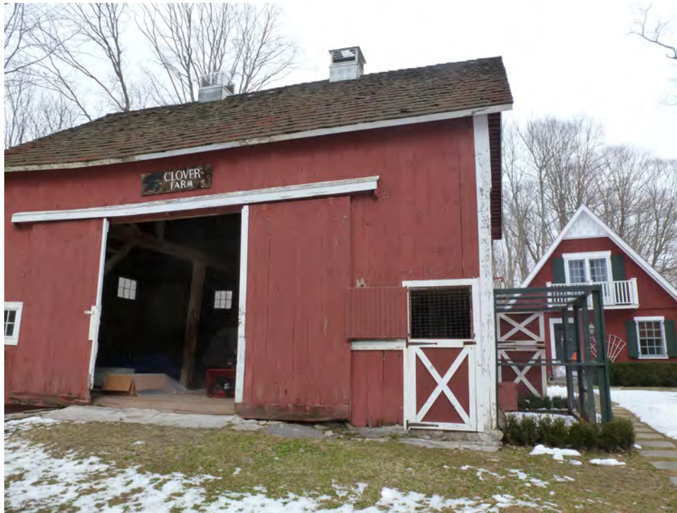
7. South context view of the barn (on the left) and the cottage (in the distance on the right). Camera facing north.
