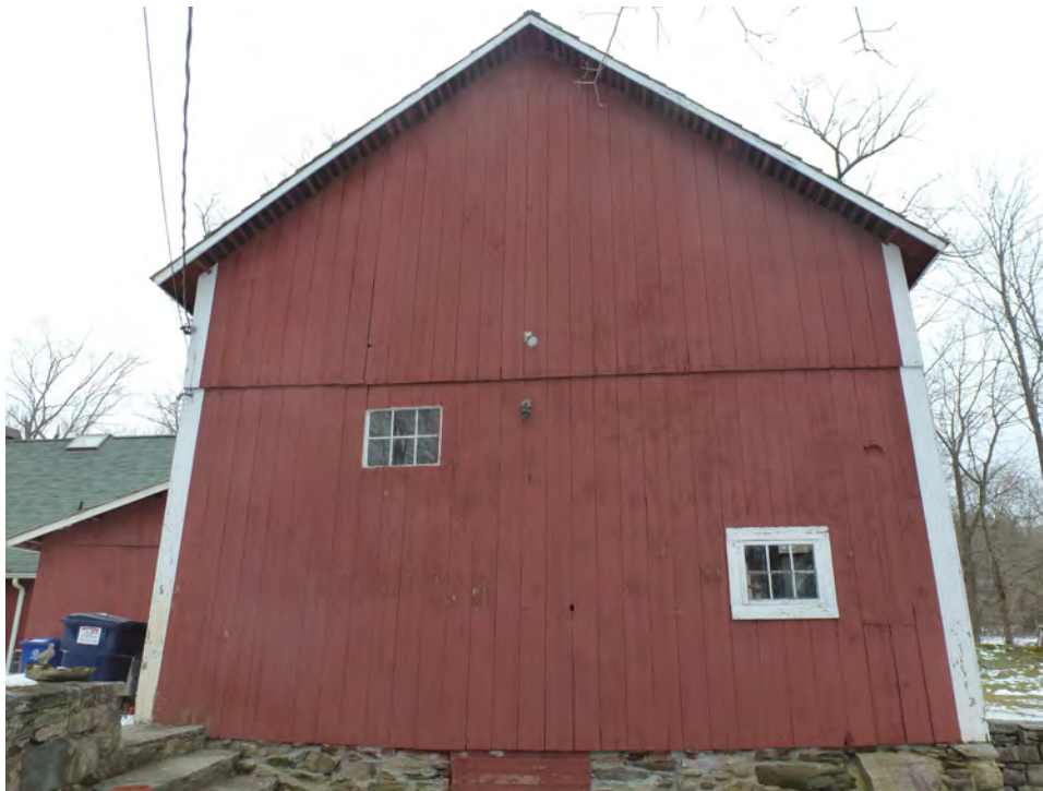
11. West gable-end of the Barn. Camera facing north.
