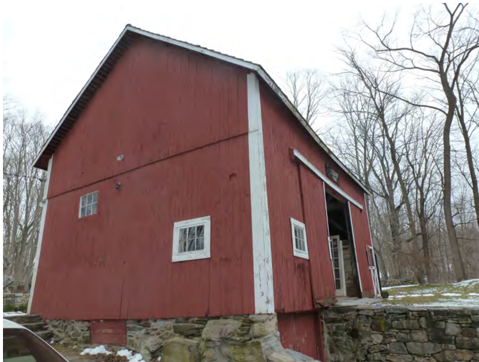
10. South eave-side and west gable-end of the Barn. Camera facing northeast.
