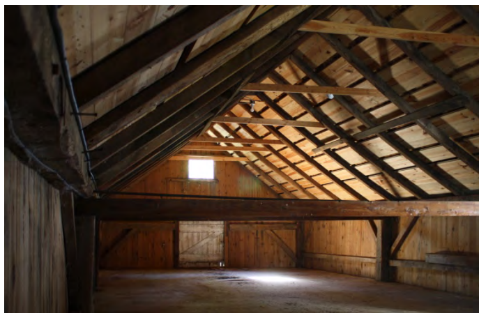
14a-b. Interior upper level of east wing. Left, interior view, camera facing south; right, detail view of tie beam with iron tension tie.
