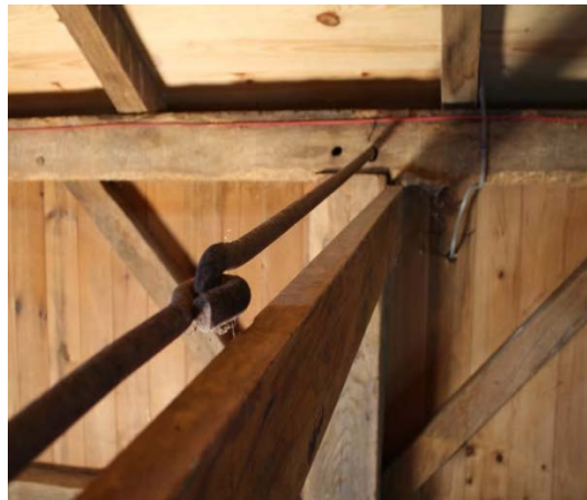
14a-b. Interior upper level of east wing. Left, interior view, camera facing south; right, detail view of tie beam with iron tension tie.
