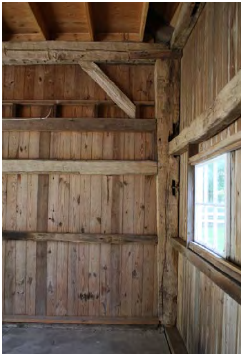
18a-b. Interior of central block. Left, detail of northwest corner showing gunstock post, camera facing northwest; right, detail of south wall reinforcing at garage door openings, camera facing south.
