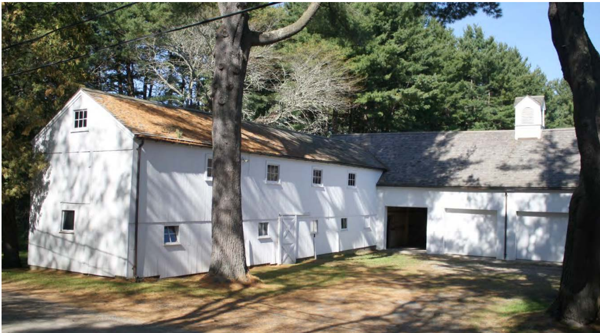
20. Southeast view of yard, showing modern overhead doors, camera facing northwest.
