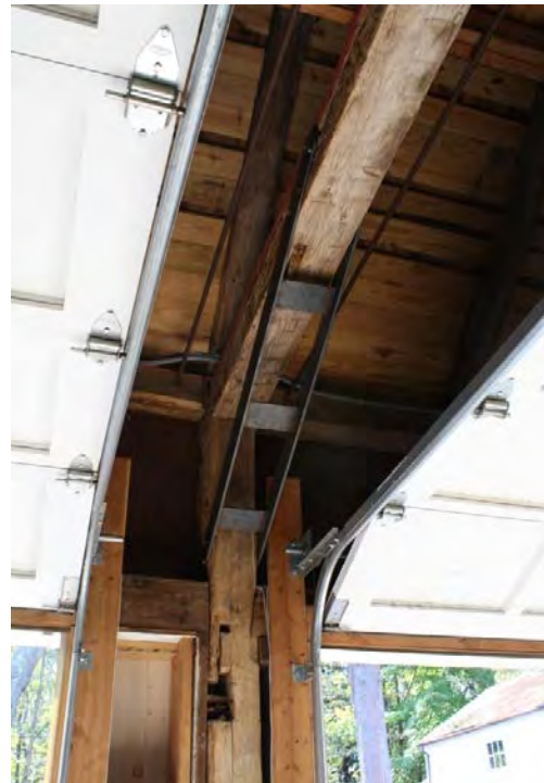
18a-b. Interior of central block. Left, detail of northwest corner showing gunstock post, camera facing northwest; right, detail of south wall reinforcing at garage door openings, camera facing south.
