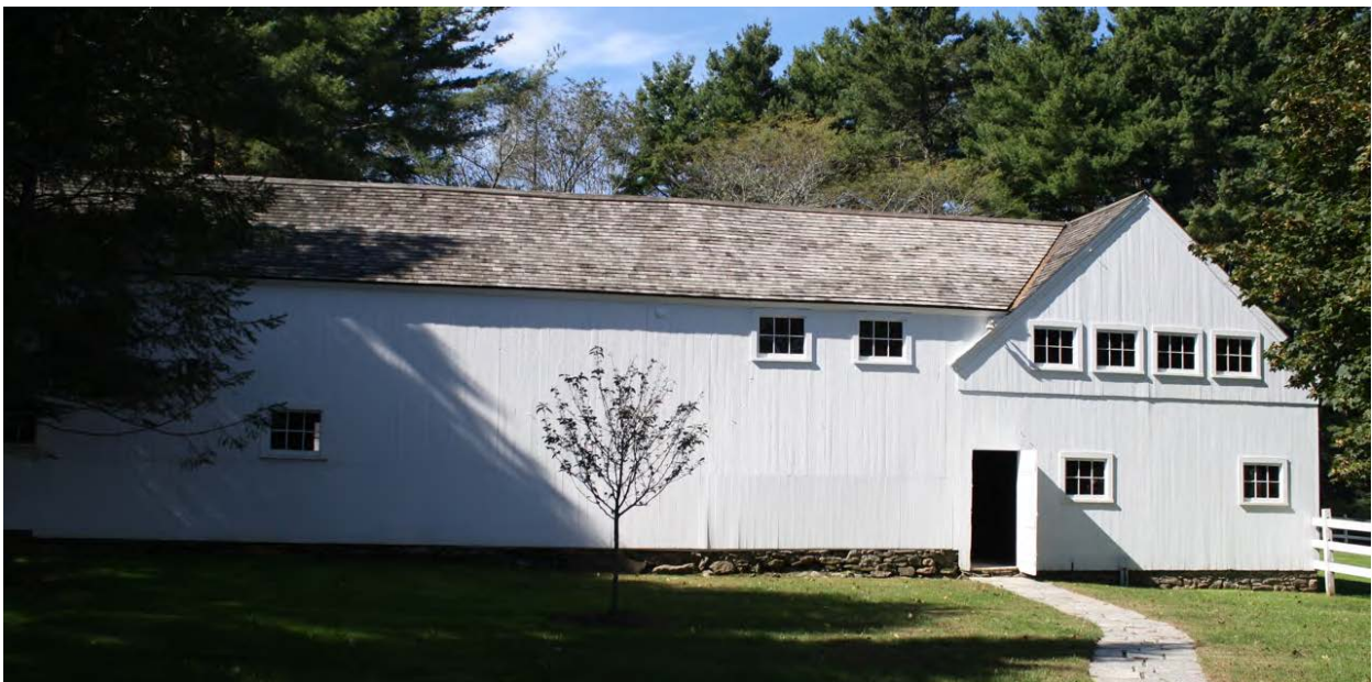
9. East view of east wing, camera facing northwest.
