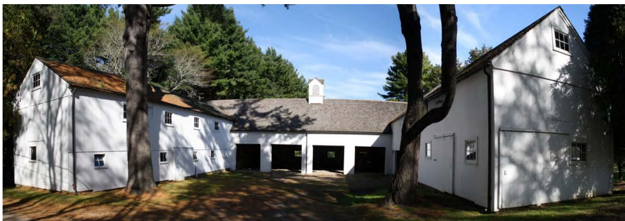
5. South view of barn, camera facing north.
