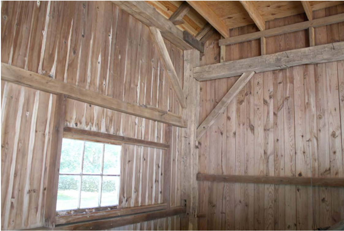
19. Interior of central block showing the dropped girt and square rule framing of the easternmost bent, camera facing northeast.
